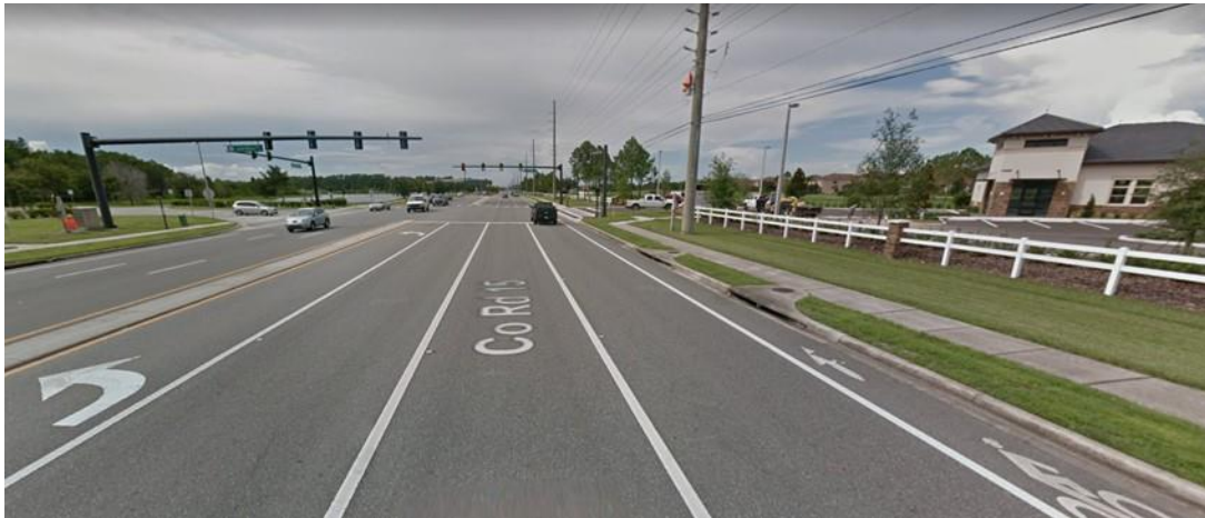
Figure 2.3.1: Pedestrian and Bicycle Facilities along Narcoossee Road
