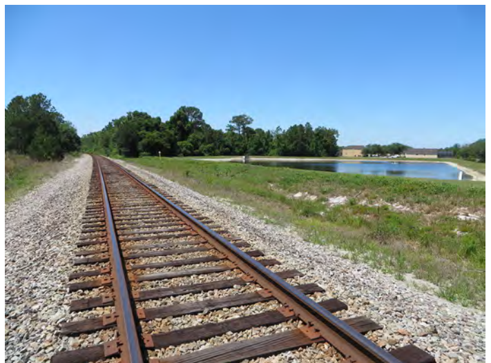
8PO07219_f Facing Southwest
