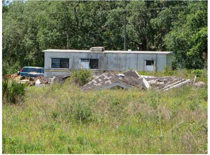
8PO08109_b Facing South
