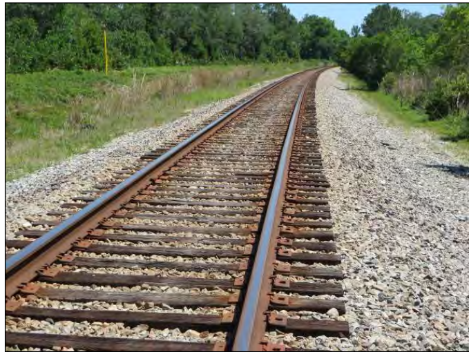
Figure 27. Resource 8PO07219/8OS02540, facing northeast.
