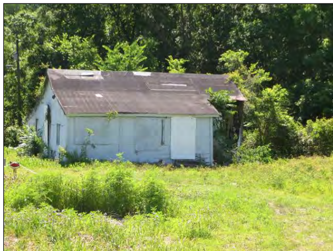
Figure 23. Resource 8PO07156 provides an example of the Frame Vernacular style within the Poinciana Parkway Extension APE. Photograph facing southeast.
