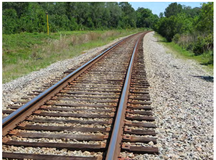
8PO07219_d Facing Northeast
