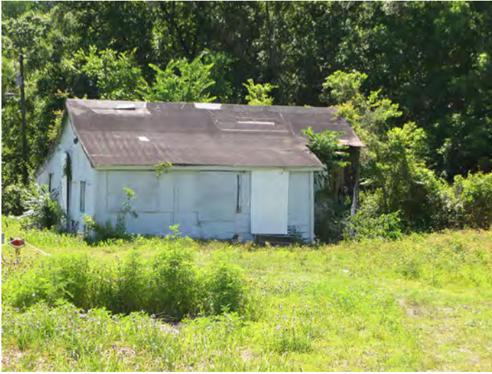
8PO07156_a Facing Southeast
