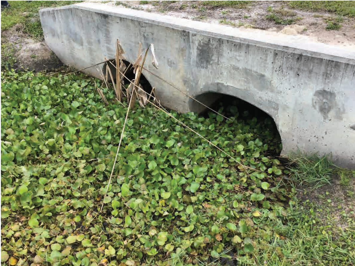
Plate 8 - EX-CD-6 is in Place with Proposed Cross Drains CD-1-08, CD-4-06, CD-5-06, & CD-5B-05B
