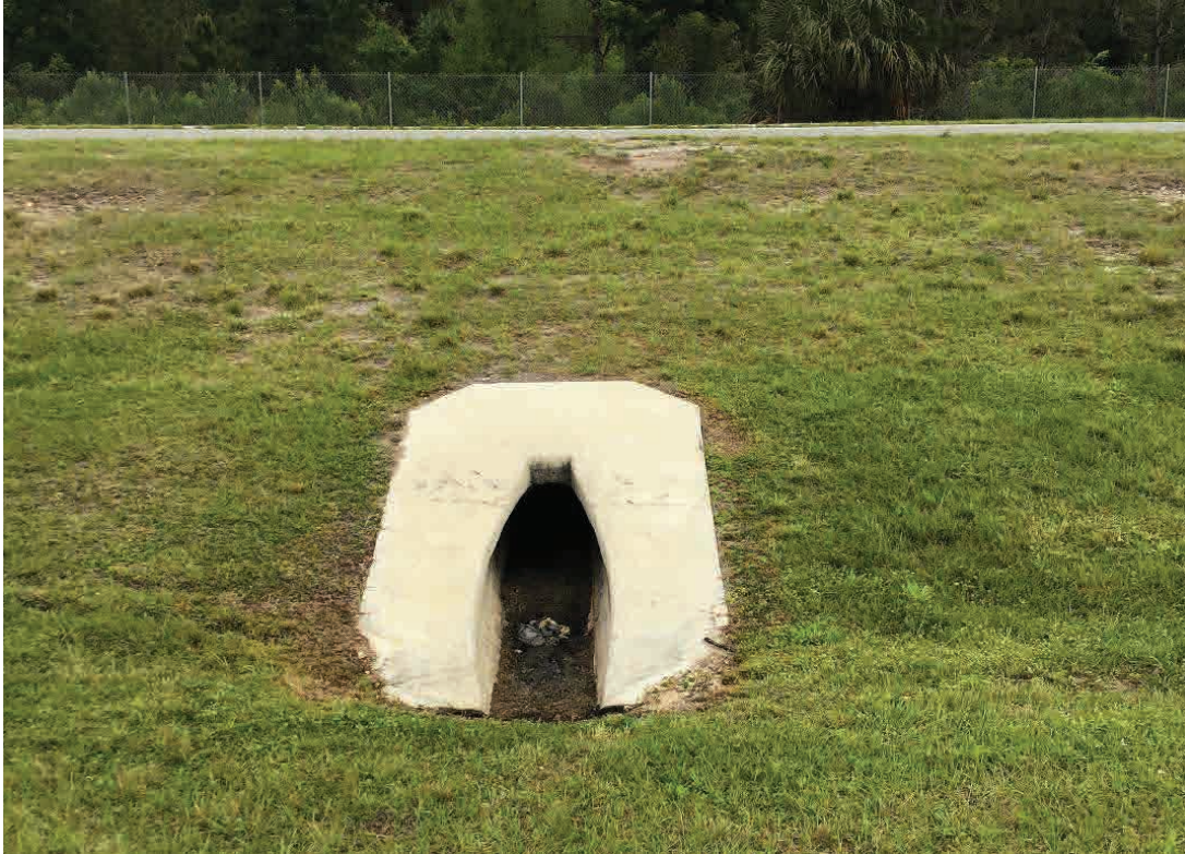
Plate 6 - EX-CD-4A is in Place with Proposed Cross Drain CD-1-06
