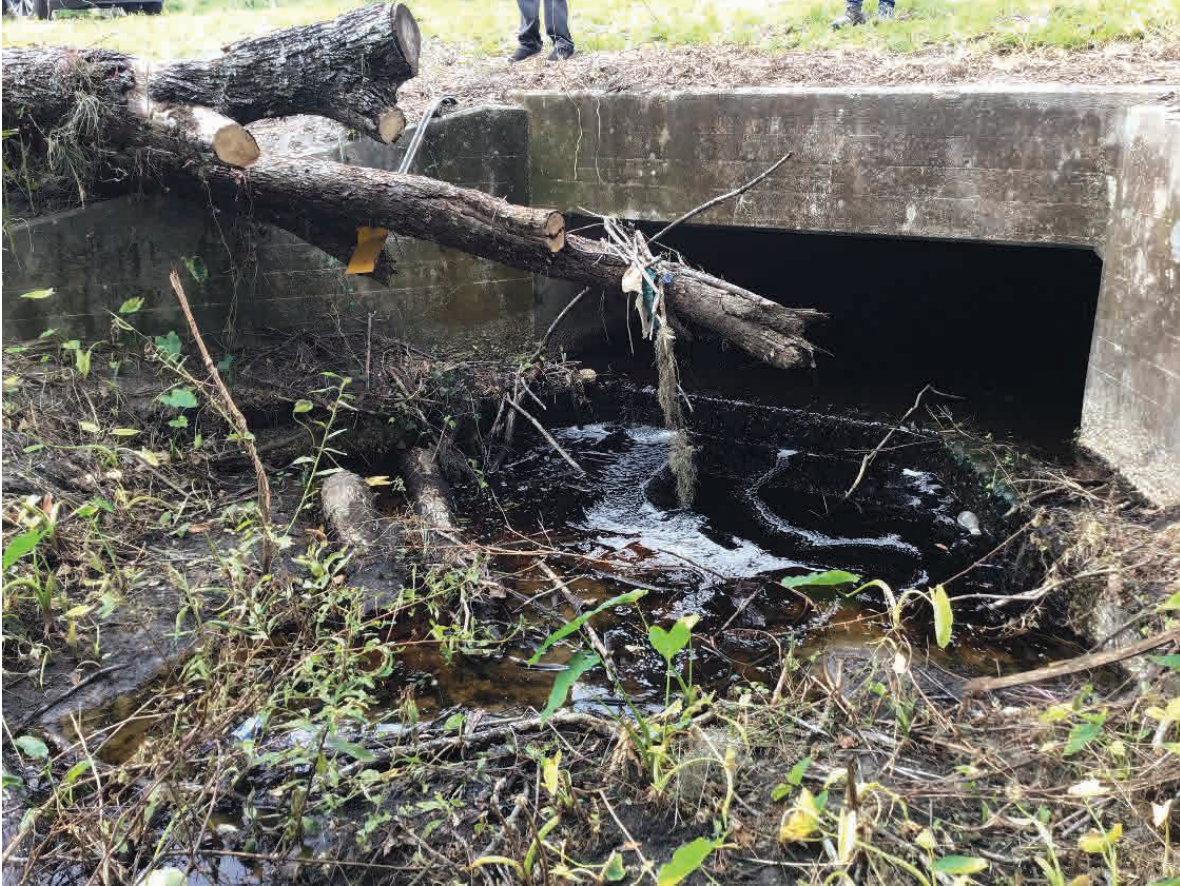
Plate 9 - EX-C is in Place with Proposed Cross Drains CD-4-02 & CD-5-02
