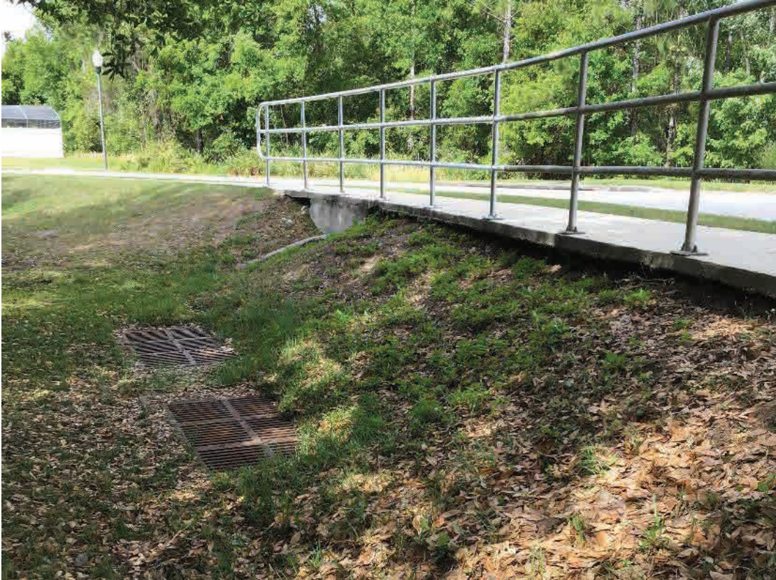
Plate 3 - Inlet Structure for EX-B is Upstream of Proposed Cross Drain CD-1-02
