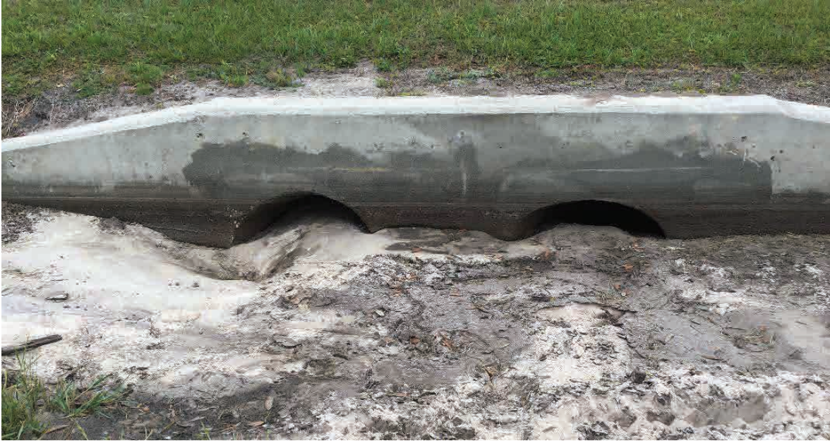
Plate 7 - EX-CD-5 is in Place with Proposed Cross Drains CD-1-07, CD-4-05A, & CD-5-05A and Upstream of Cross Drains CD-4-05B, CD-5-05B
