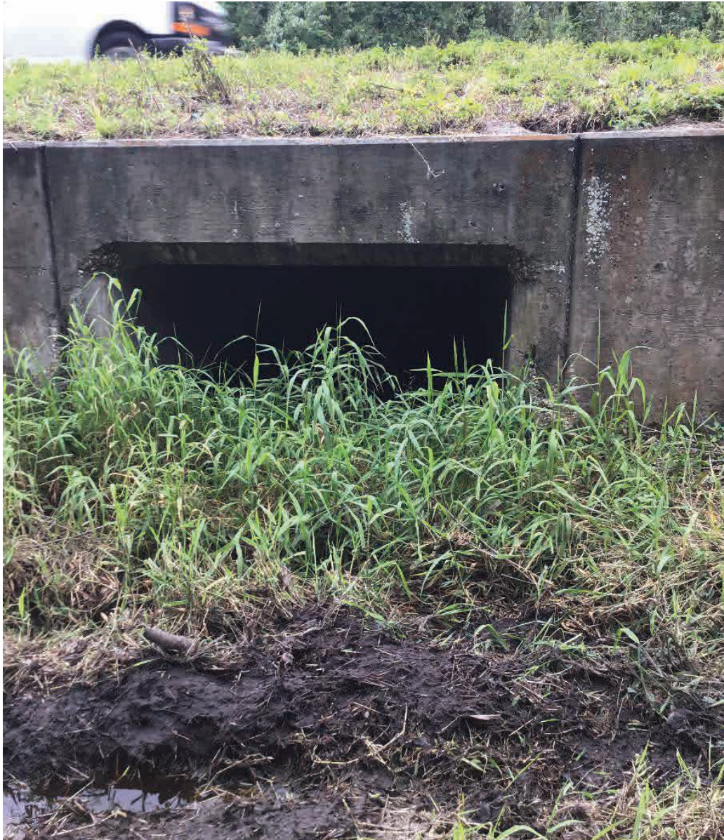
Plate 4 – EX-CD-1 is in Place with Proposed Cross Drain CD-1-03
