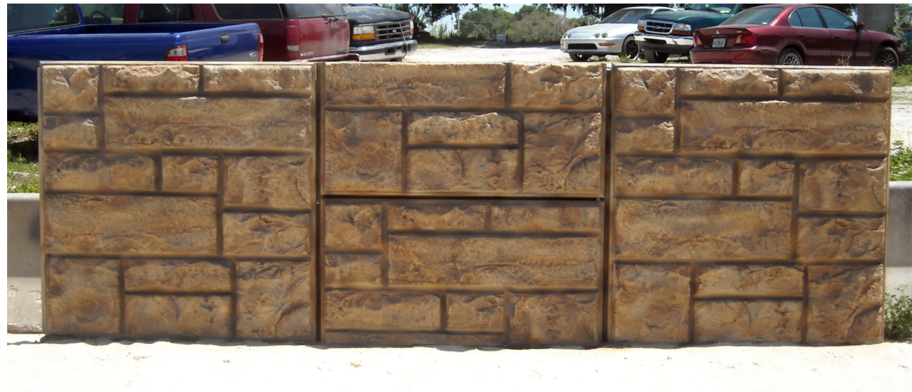
FORMLINER MOCK-UP PANEL
