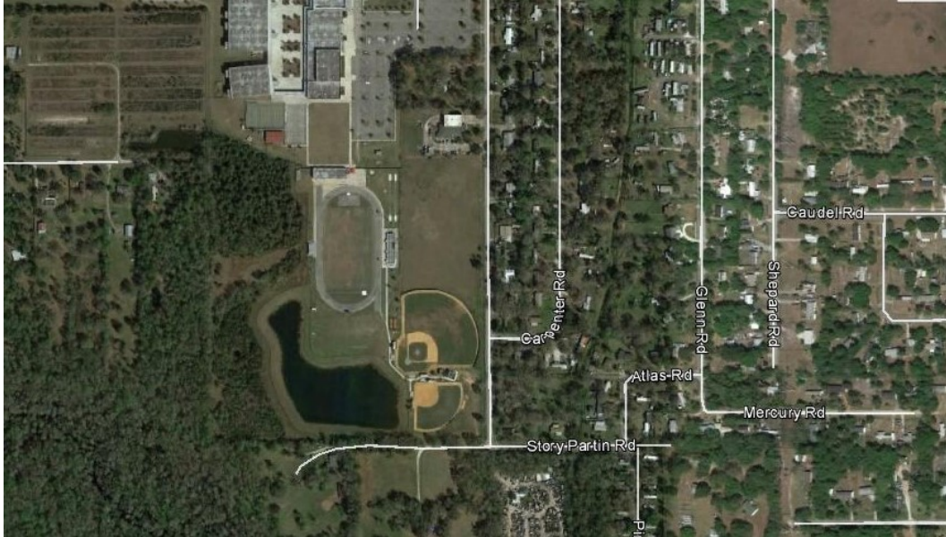
Photograph 6-13 AA-18 Stormwater pond on school grounds, aerial view
