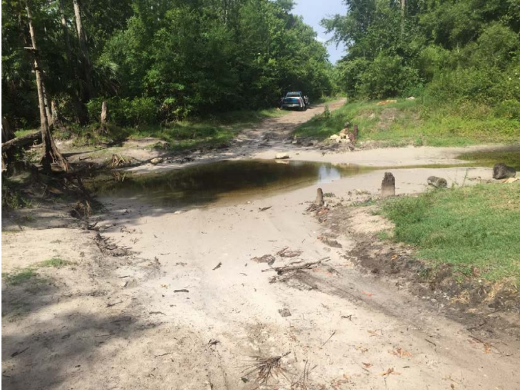
Photograph 6-9 AA-13 where Old Cheney Highway crosses the Econlockhatchee River, facing west
