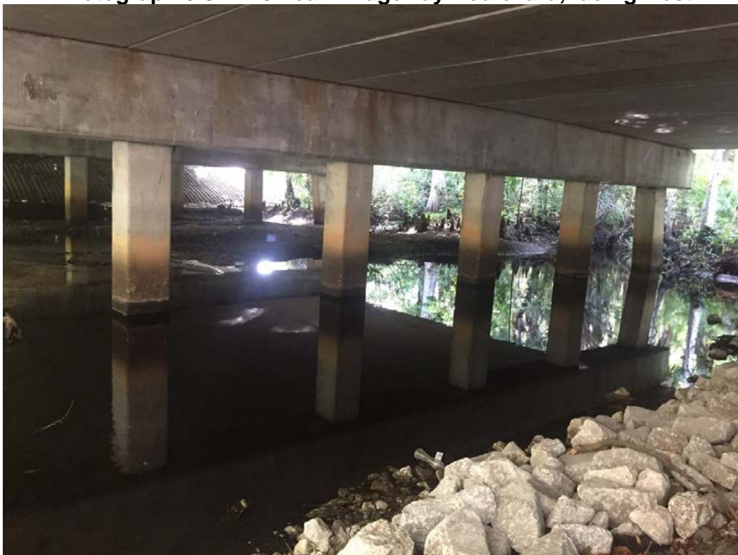
Photograph 6-4 AA-5 beneath Bridgeway Boulevard, facing northeast
