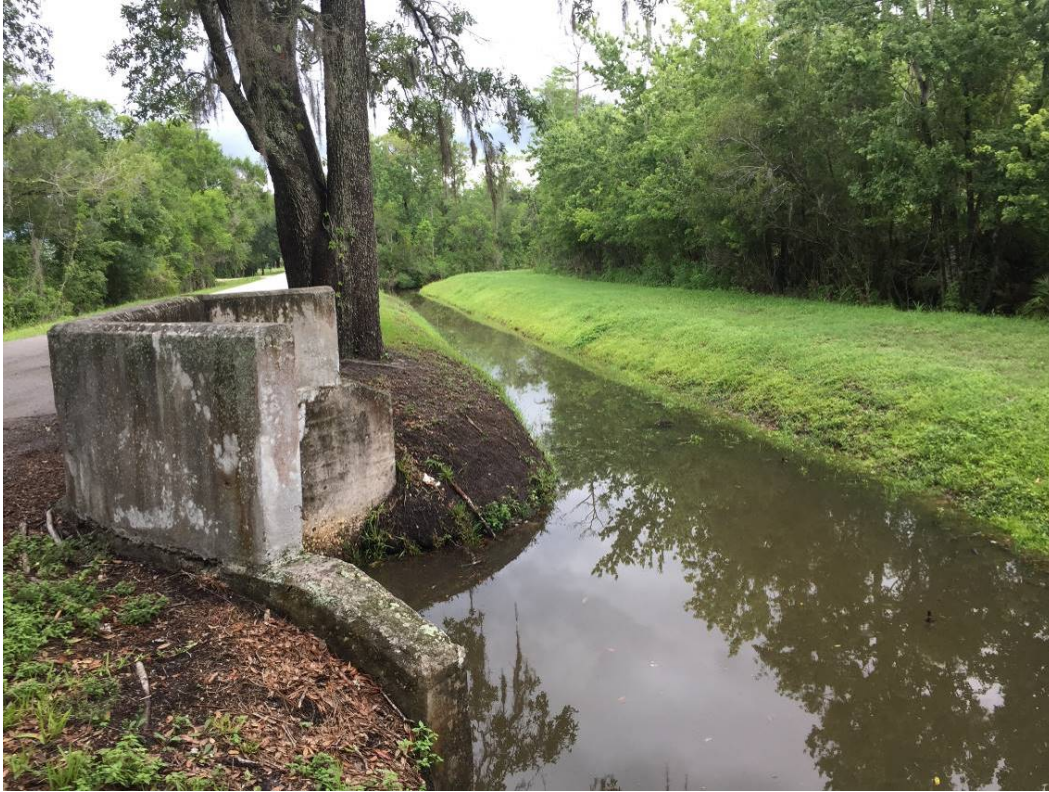
Photograph 6-26 AA-25 drainage north of SR 50, connecting to canal, facing northwest
