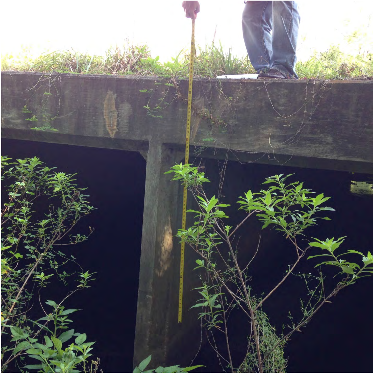
SR 50-CD5(3-10'x6' CBC) (South Side of the Culvert)
