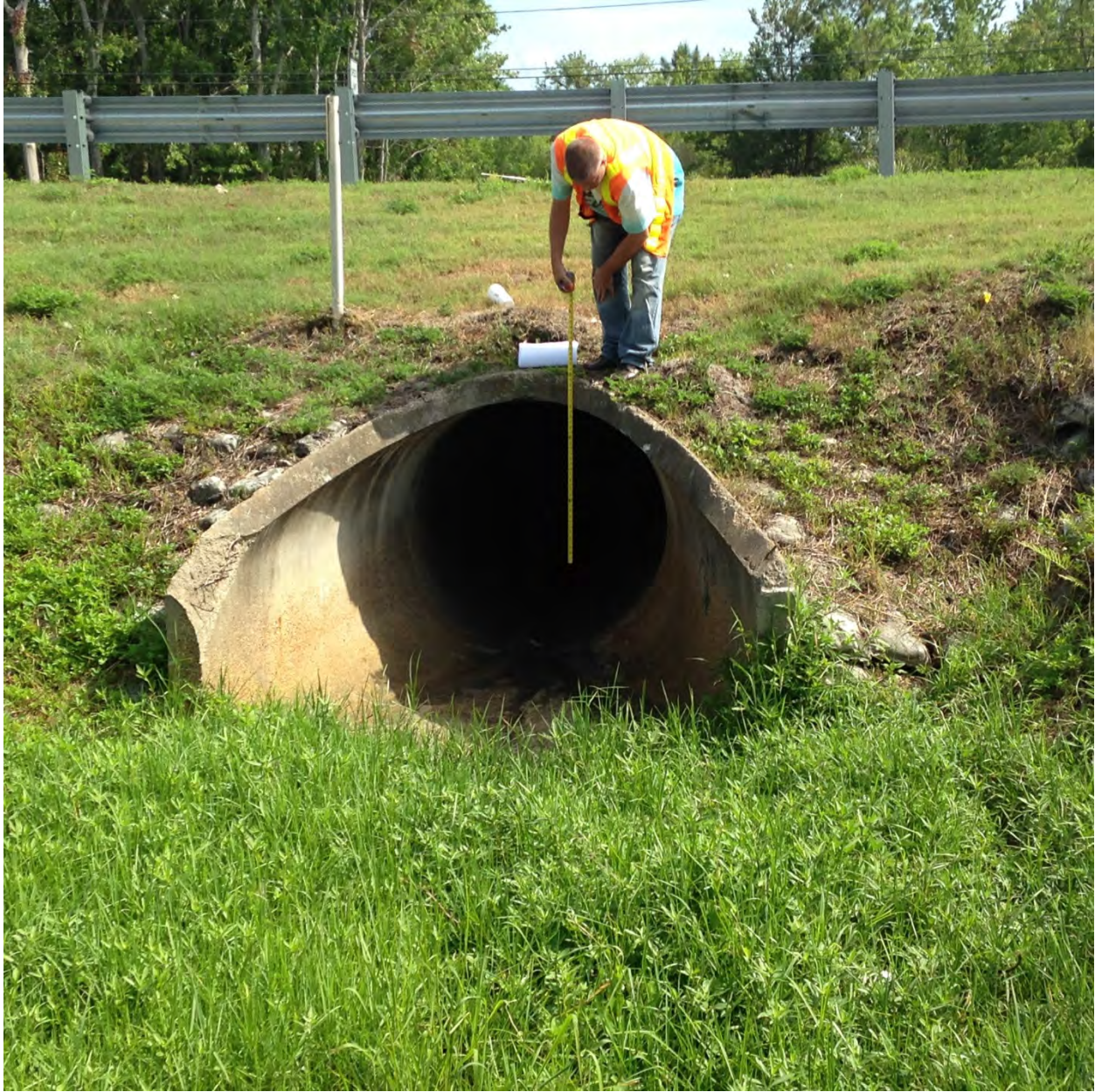
SR 50-CD7 (1-4' x 4' CBC & 1-54" RCP Jointed) (South Side of the Culvert)
