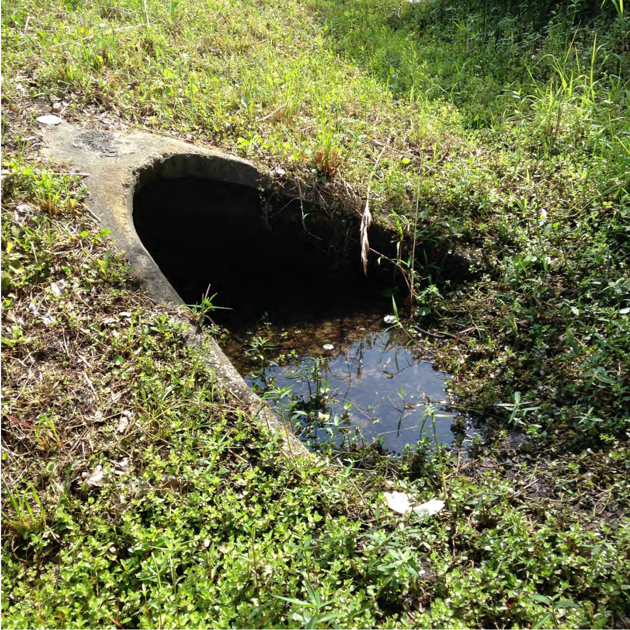
SR 50- CD8 (1-30" RCP) (South side of the culvert)
