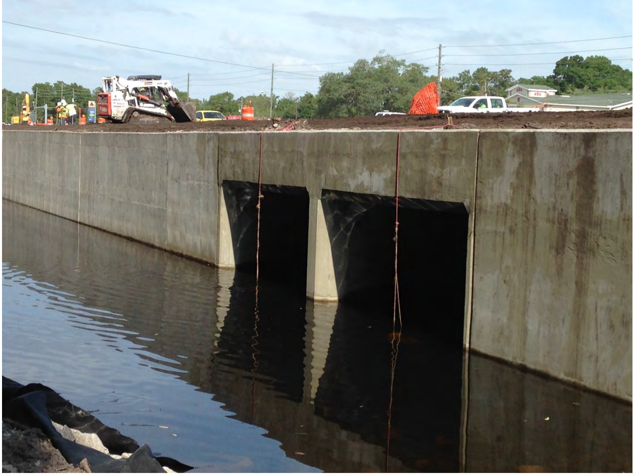
SR 50-CD3 (2-12.95' x 8.5' CBC) (South Side of the Culvert)
