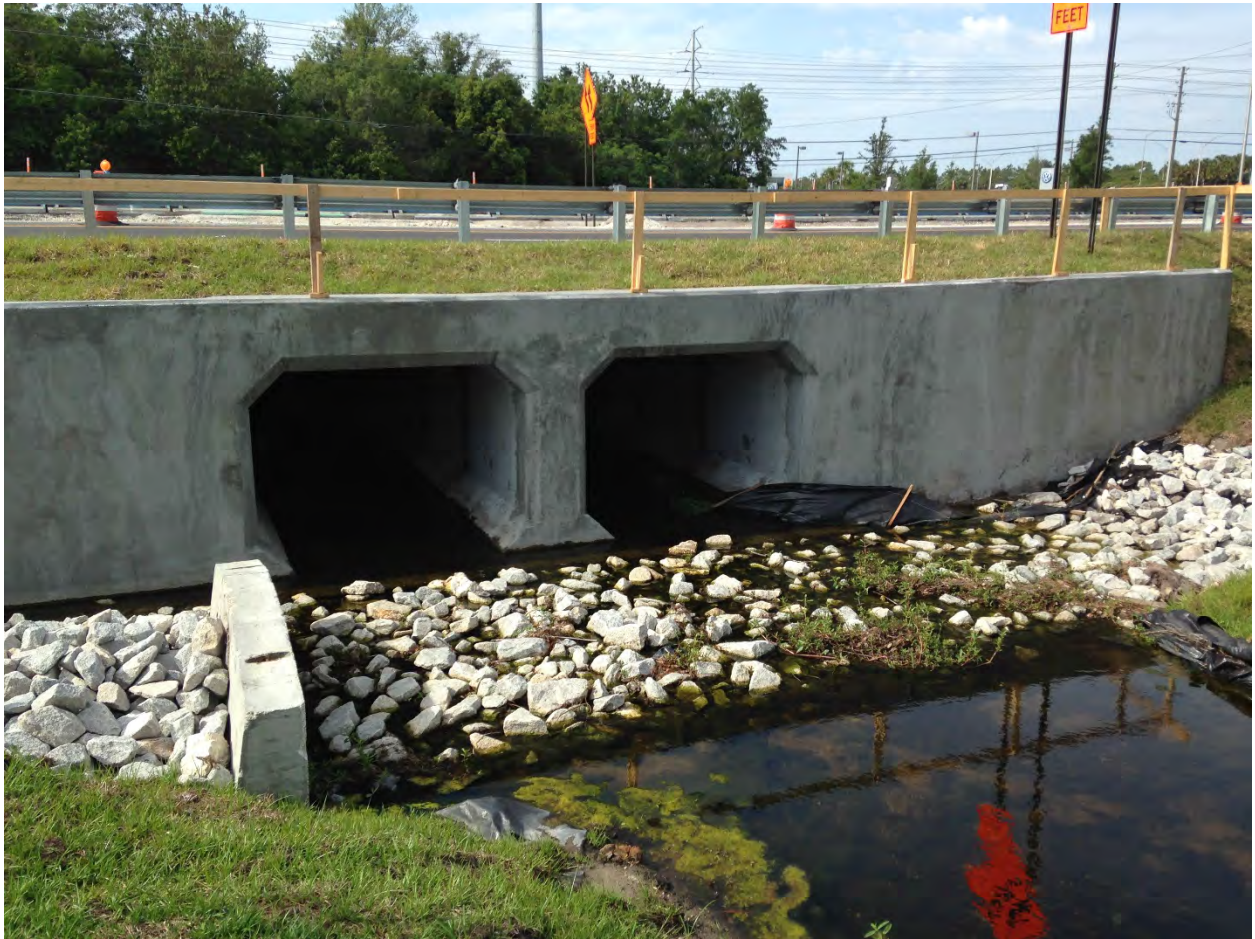
SR 50- CD1 (2-8' x 6' CBC) (Looking North Side of the Culvert)
