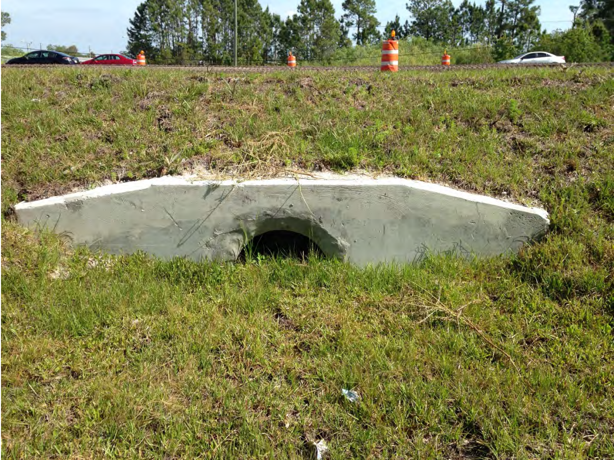
SR 50-CD4 (1-30" RCP) (South Side of the Culvert)
