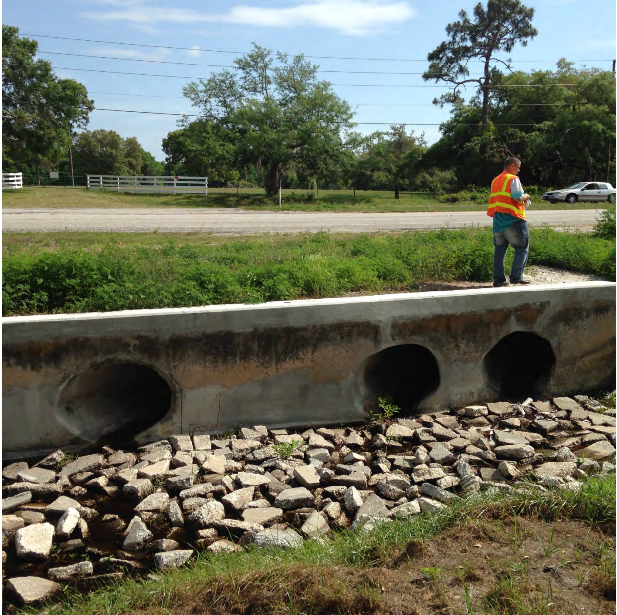
SR 50-CD6 (3-36" RCP) (South side of the Culvert)
