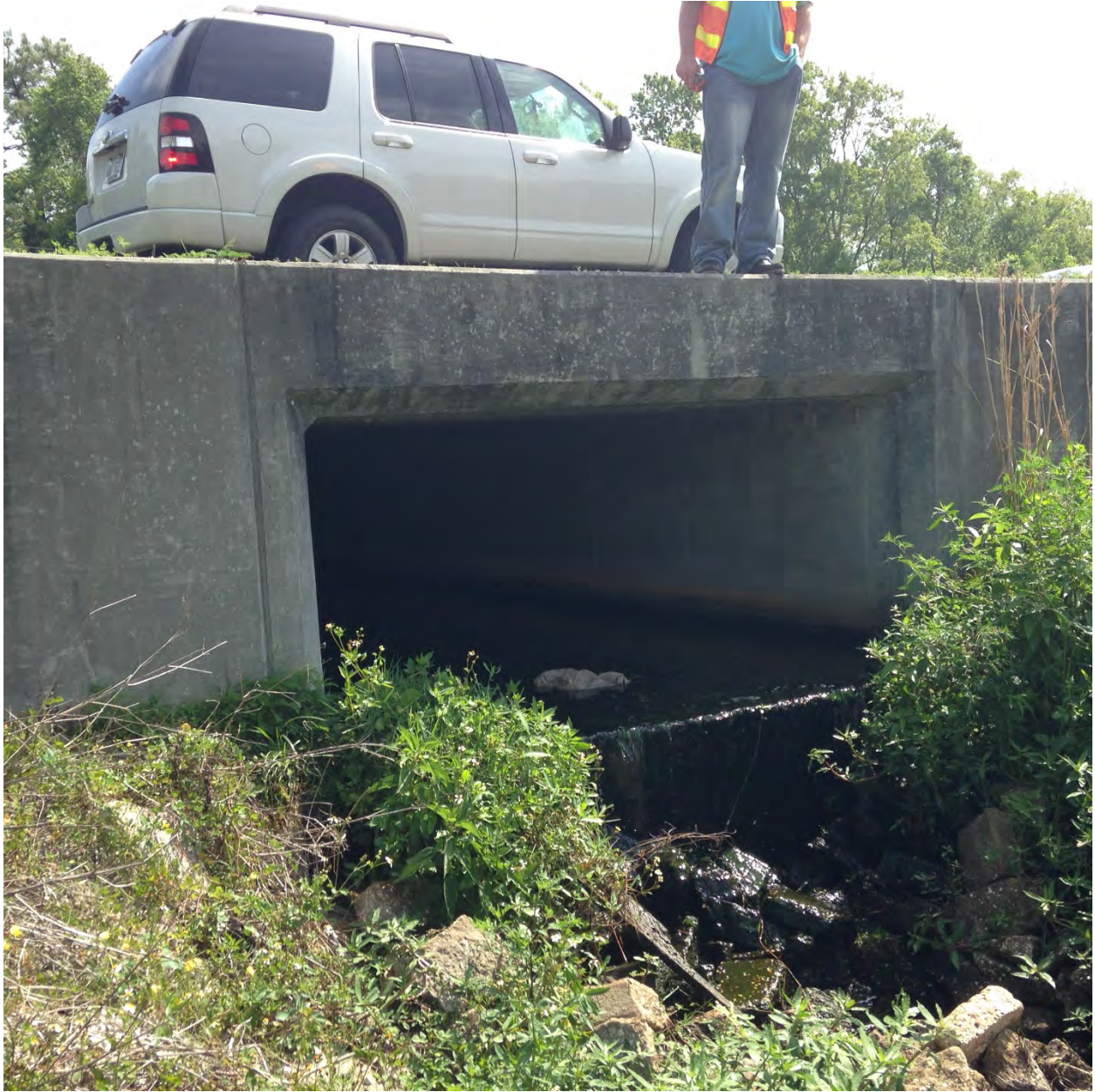
SR 50-CD10 (1-10'x4' CBC) (South Side of the Culvert)
