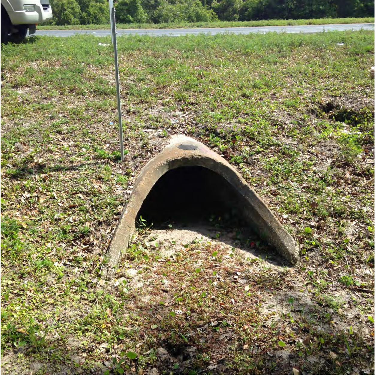
SR 50-CD11 (1-24" RCP) (South Side of the Culvert)
