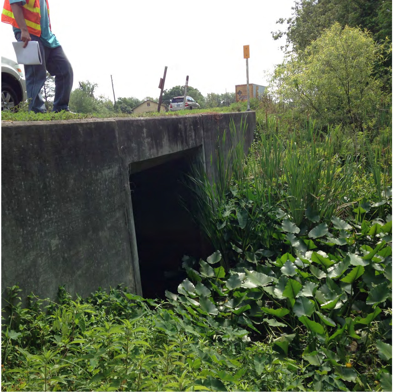
SR 50- CD9 (1-8'x7' CBC) (South Side of the Culvert)
