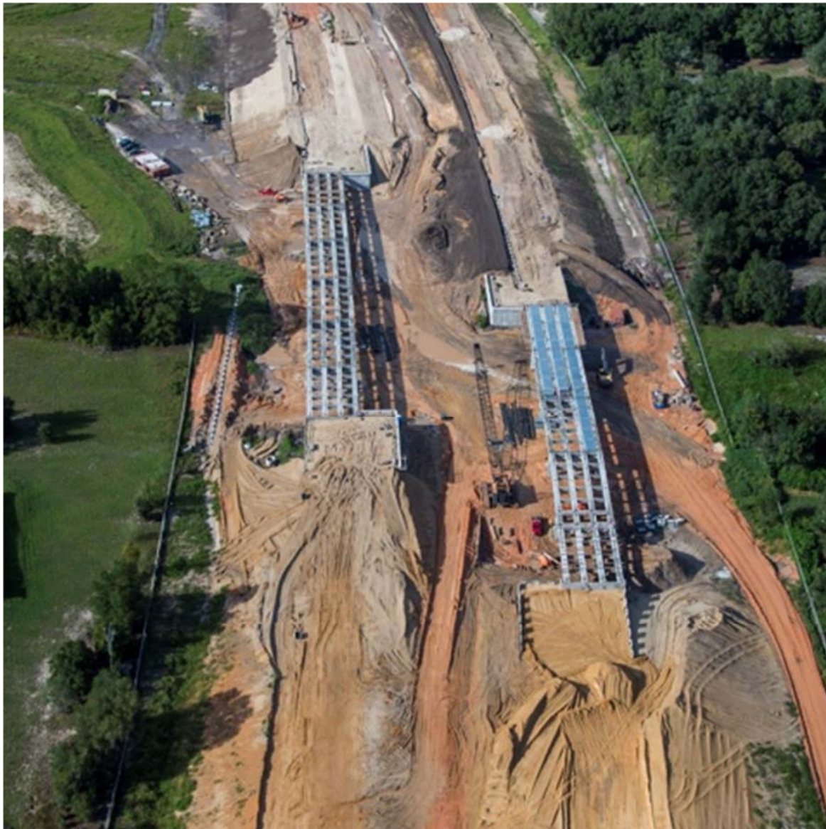
S.R. 429 – Wekiva Parkway Construction (Photo Courtesy of Aerial Innovations)
