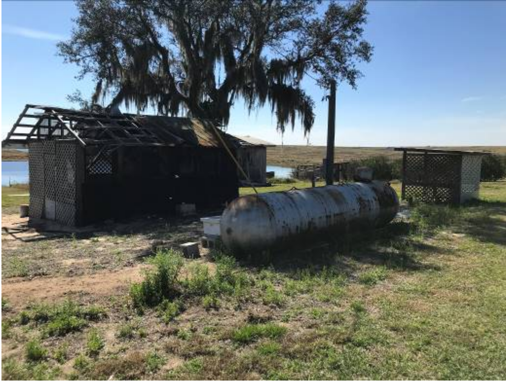
Photograph 5-19 Tank and sheds on north side of AA-7, facing southwest
