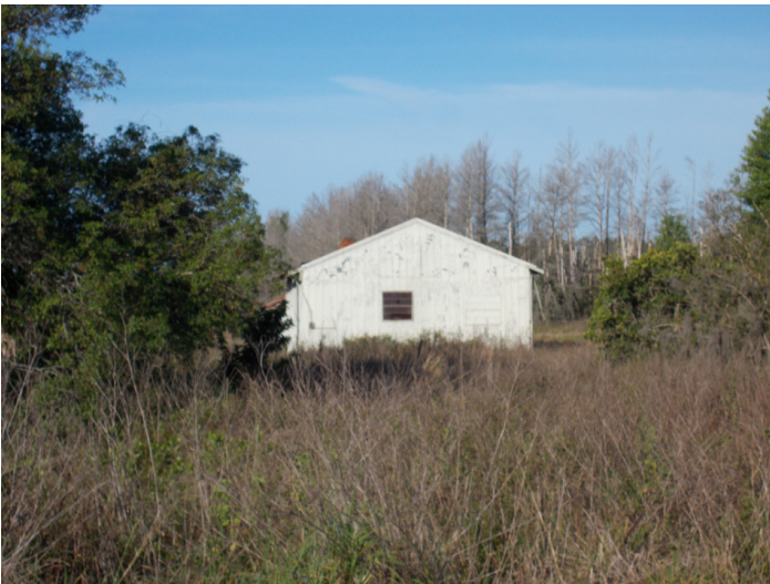
8LA04796_c Facing West
