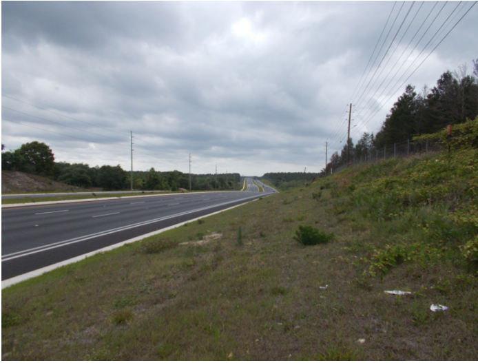
8LA04779_a Facing South
