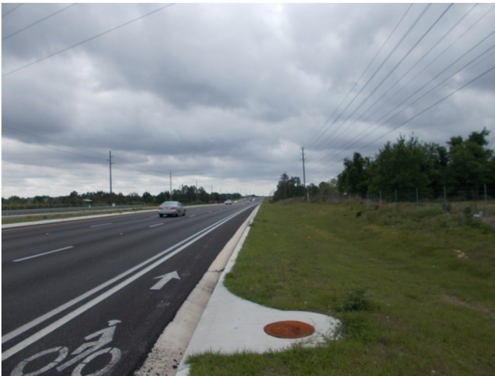
8LA04779_c Facing South
