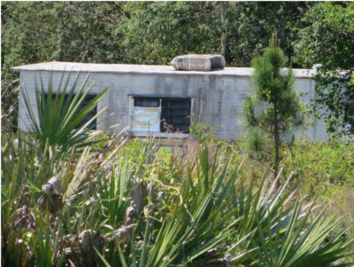
8PO08109_c Facing South
