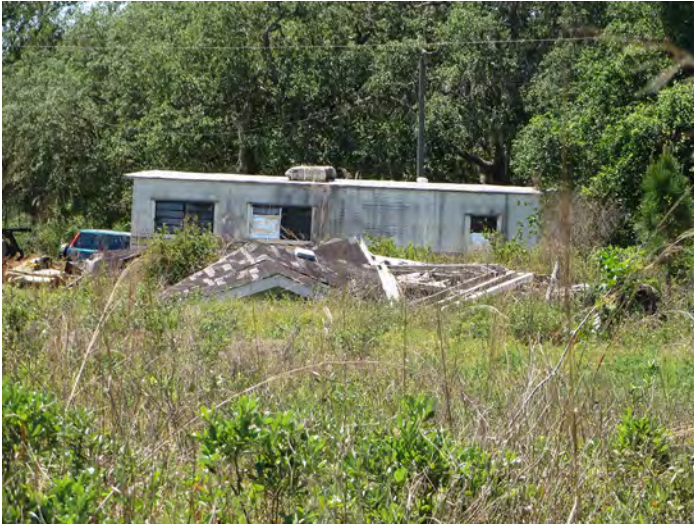
8PO08109_a Facing South
