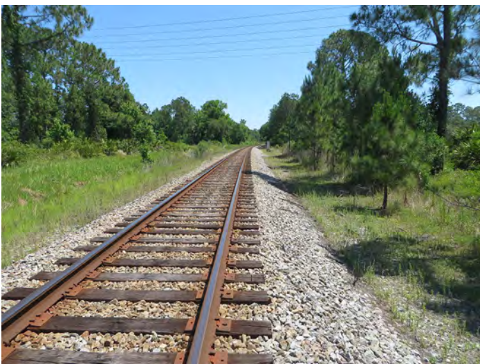
8PO07219_e Facing Northeast
