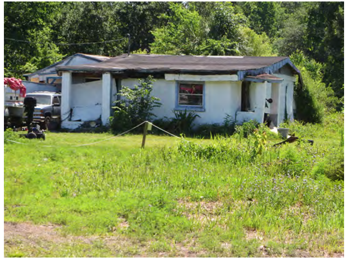
8PO08200_b Facing Southeast
