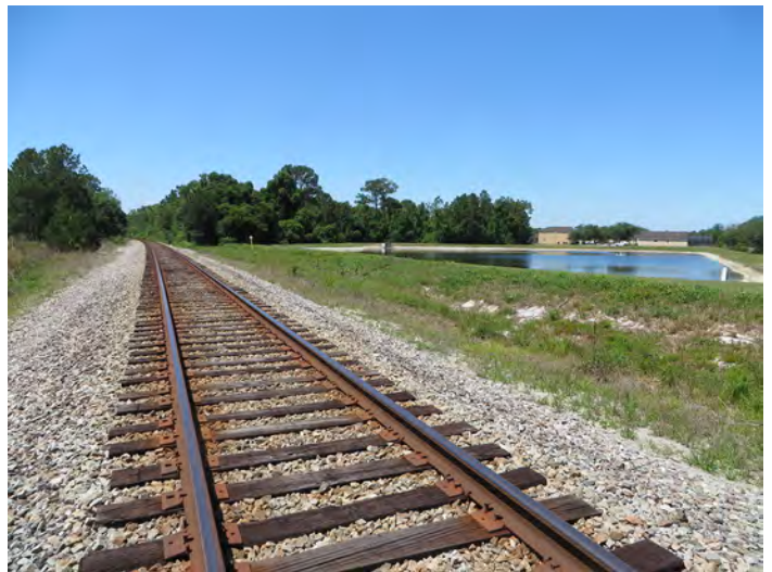
8OS02540_f Facing Southwest
