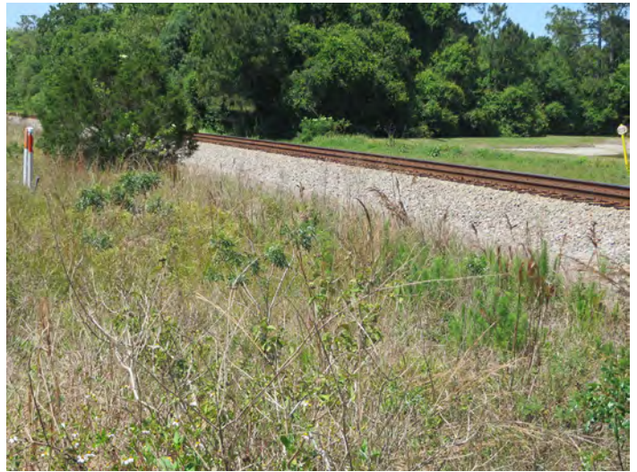
8PO07219_b Facing West
