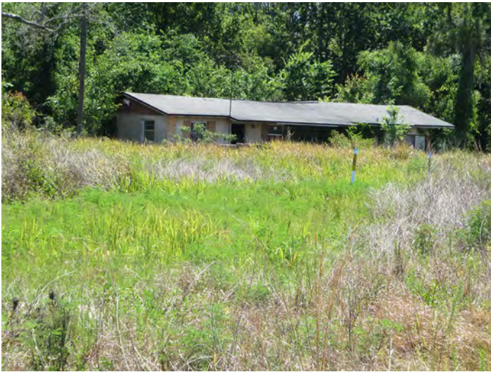
8OS02937_a Facing East
