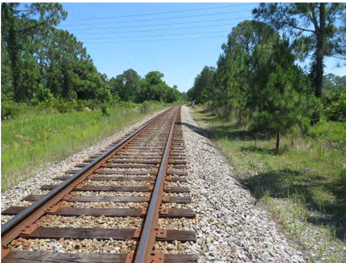
8OS02540_e Facing Northeast
