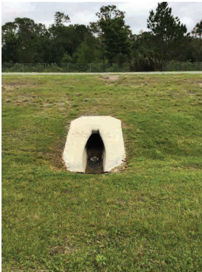
EX-CD-4A; Upstream End (Southwest), Facing Northeast
