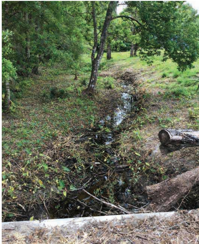
EX-C; Downstream End (Southeast), Facing Northeast
