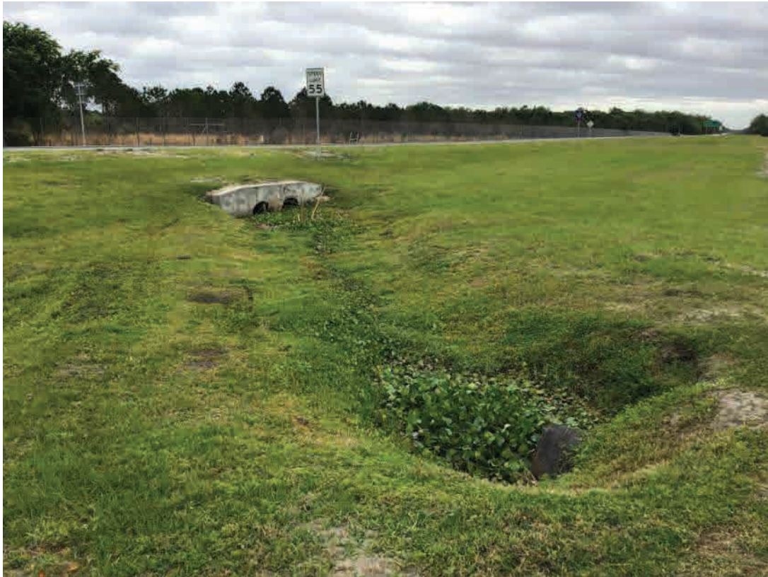
EX-CD-6; Upstream End (Southwest), Facing Northeast
