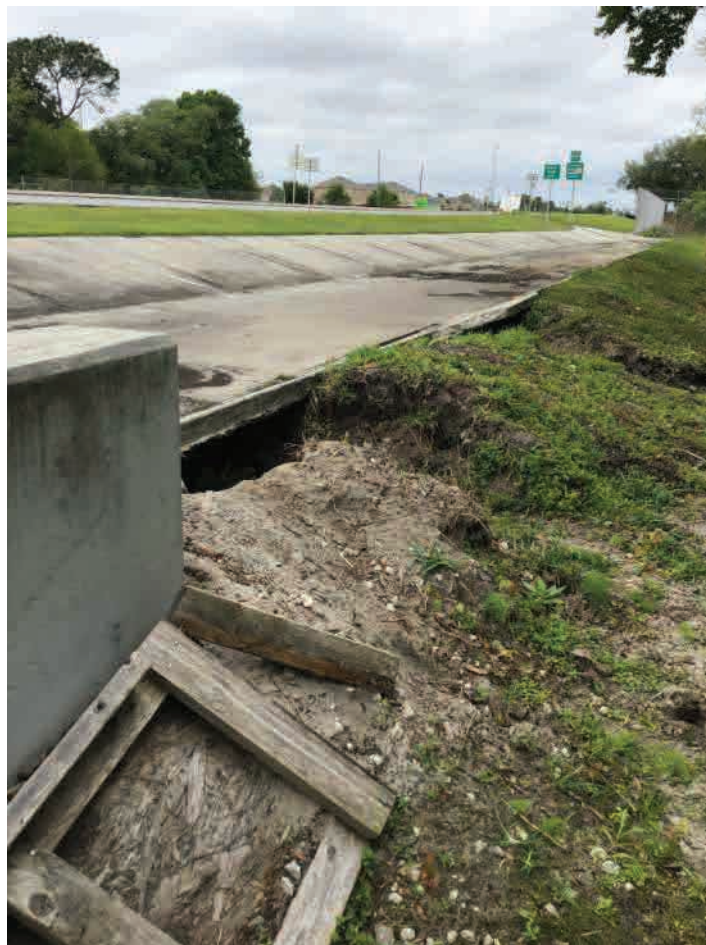
EX-CD-6; Downstream End (Northeast), Facing Northwest
