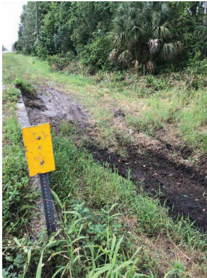
EX-CD-1; Upstream End (Northwest), Facing Southwest
