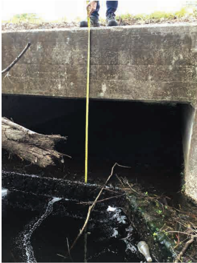
EX-C; Downstream End (Southeast), Facing Northwest
