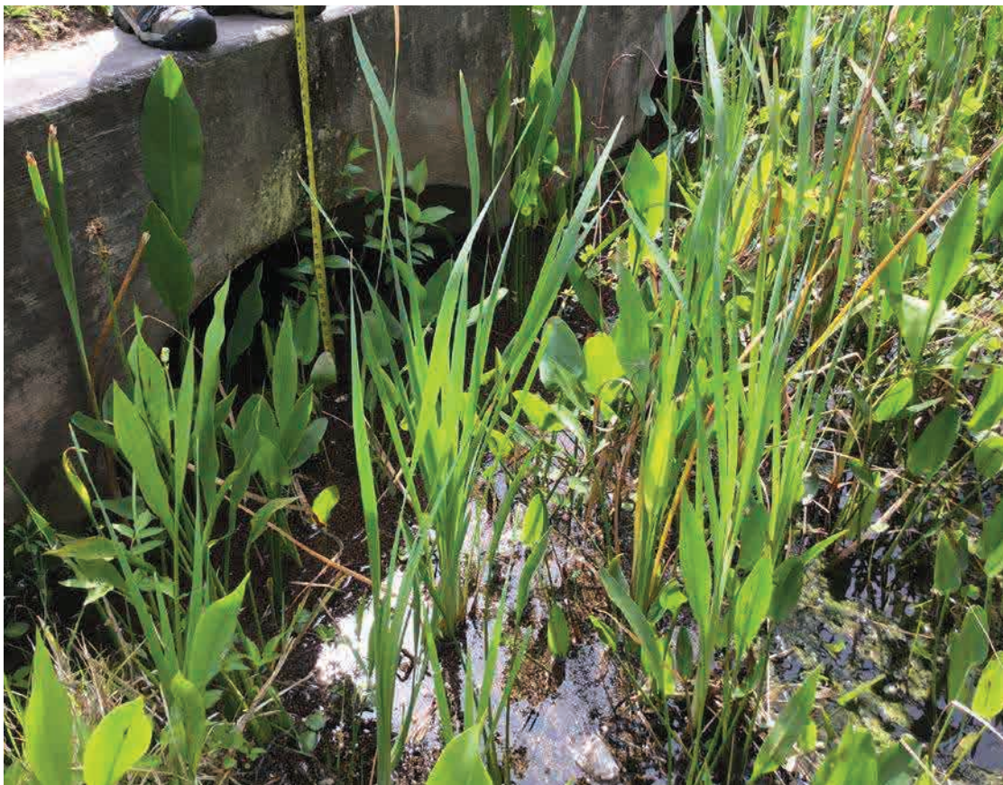
EX-A; Upstream End (West)
