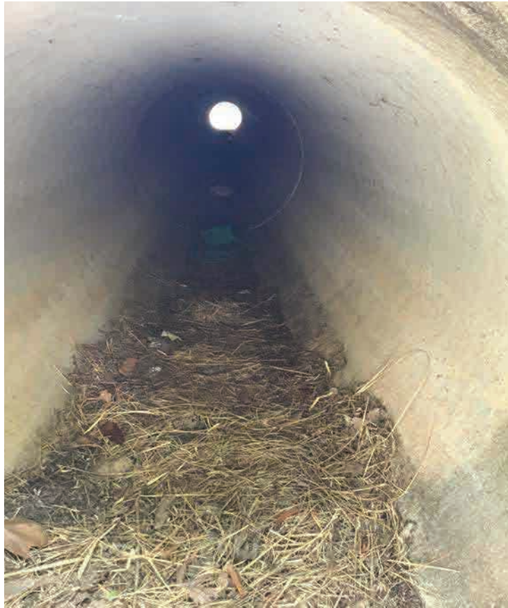
EX-E; Upstream End (West), Facing East
