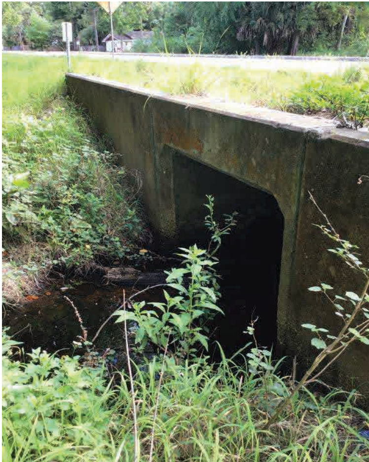
EX-L; Upstream End (Northwest), Facing East
