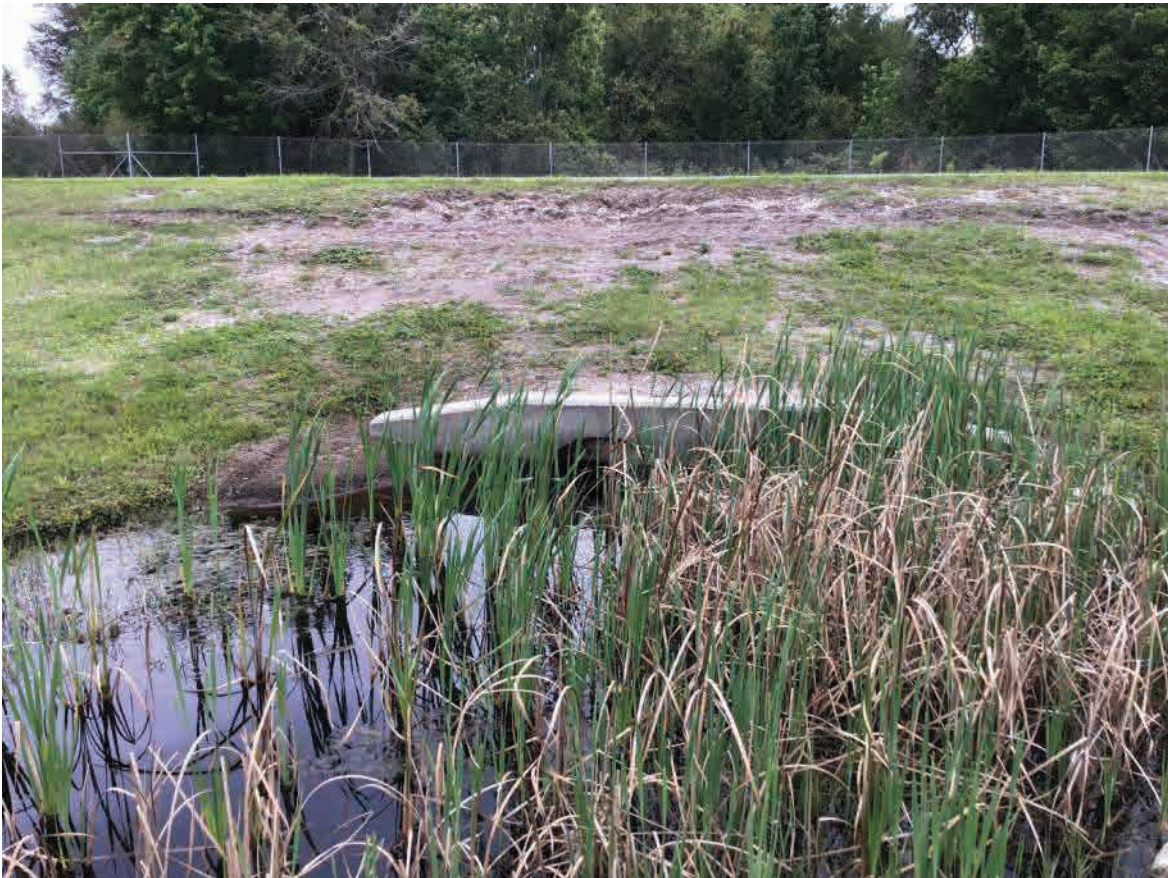
EX-CD-4; Upstream End (Southwest), Facing Northeast
