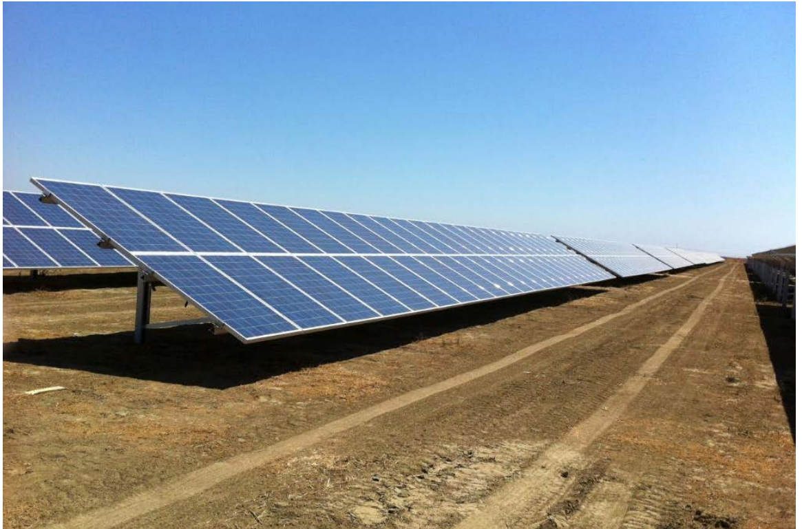
Figure 5.5.1 is an example of a typical fixed tilt racking design for reference
