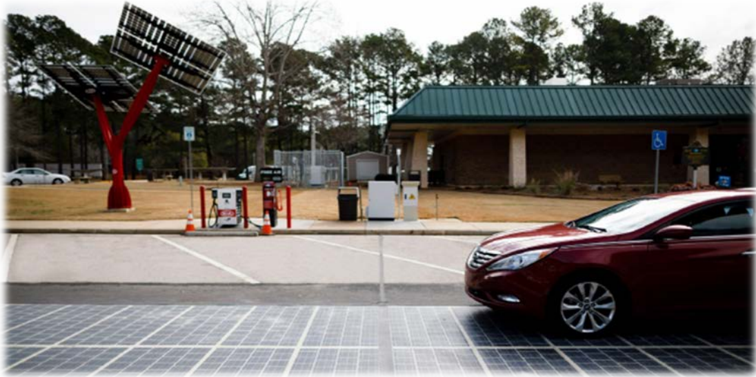
Figure 9.2.1. Wattway Installation in Westpoint, Georgia, Used for Self-Consumption and Charging Station
