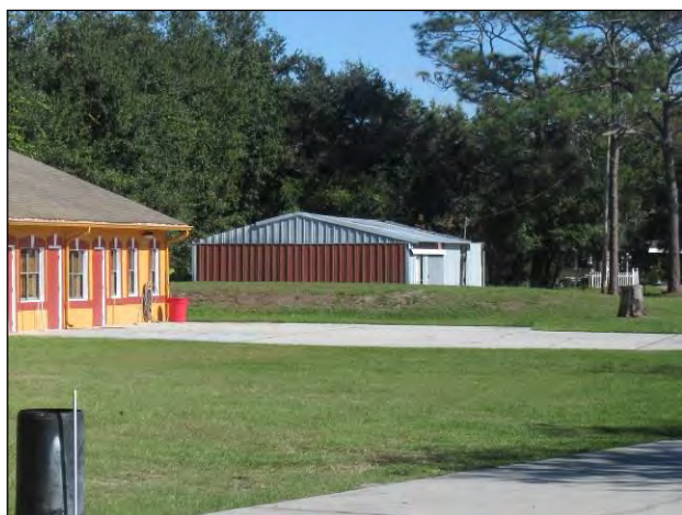
Figure 18. Resource 8OR11098 provides an example of the Industrial Vernacular style within the current project APE. Photograph facing northeast.
