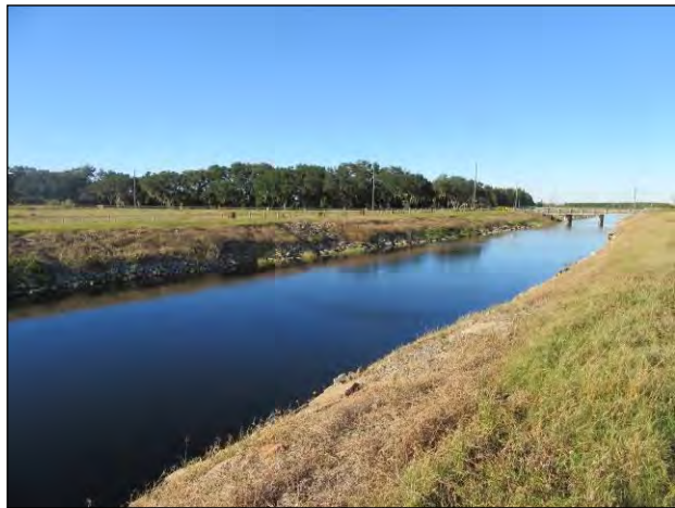
Figure 22. Resource 8OR10228, facing northwest.
