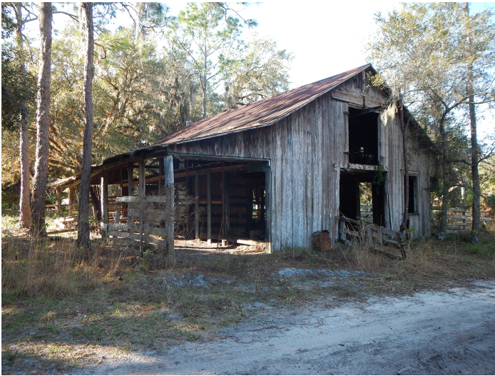
8OS03116_g Facing Southwest
