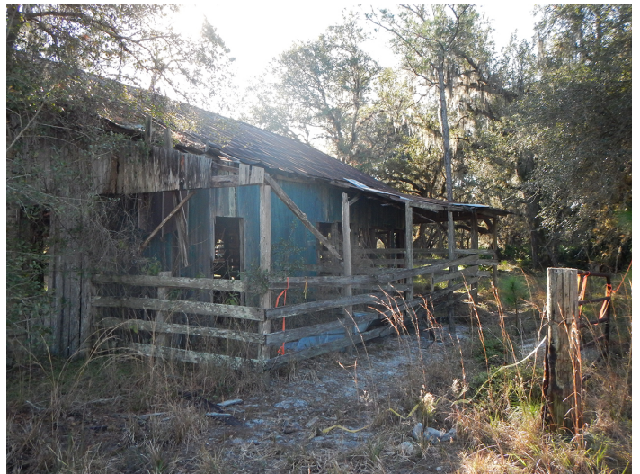
8OS03116_d Facing Southeast
