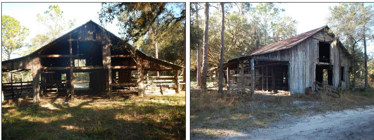
Figure 21. Resource 8OS03116. Left, facing north; right, facing southwest.
