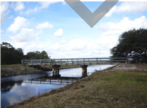
Figure 2.20.1: Bridge over C-32C Canal (Looking North)
