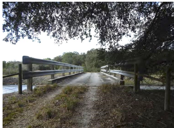
Figure 2.20.2: Bridge over C-32C Canal (Looking West)
