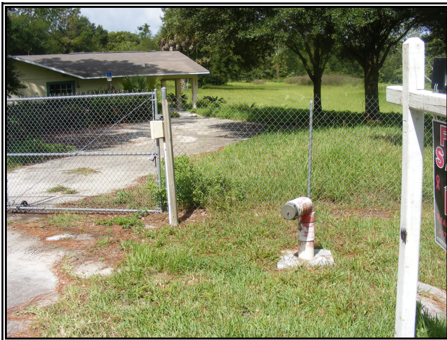
6. LOOKING WEST AT THE FIRE DEPARTMENT STANDPIPE
