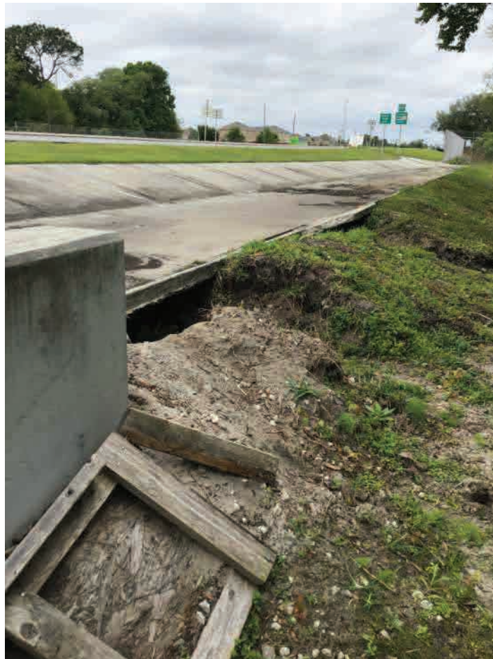
EX-CD-6; Downstream End (Northeast), Facing Northwest
