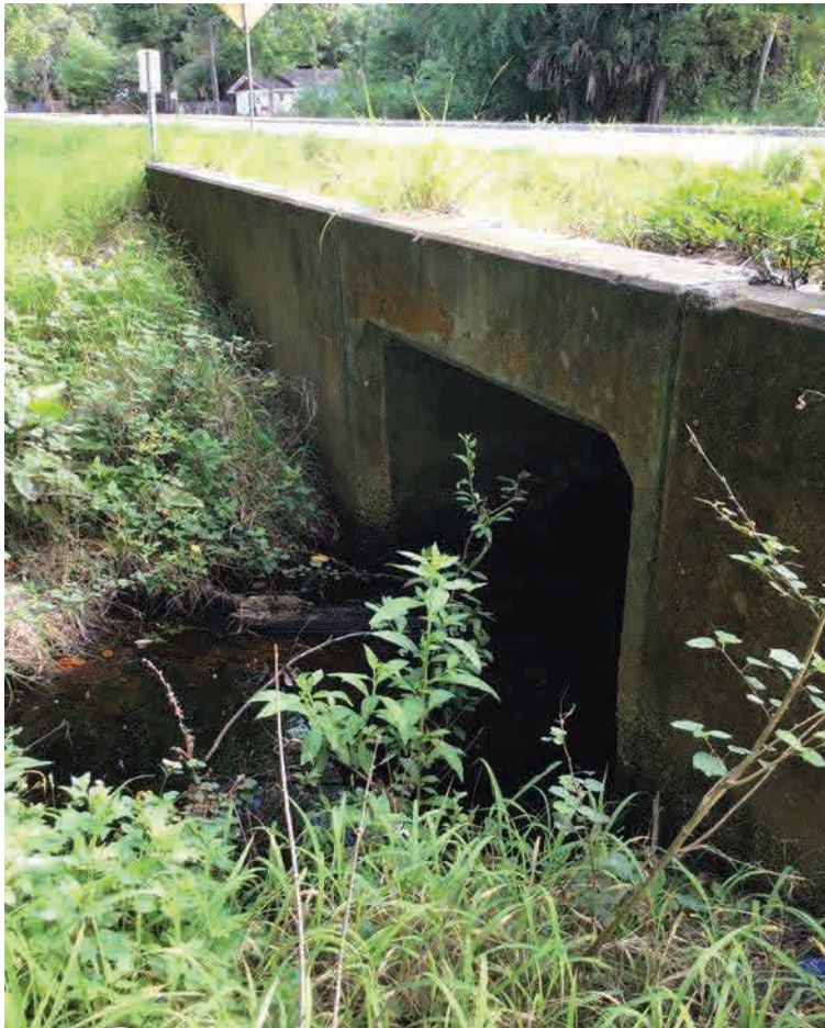
EX-L; Upstream End (Northwest), Facing East
