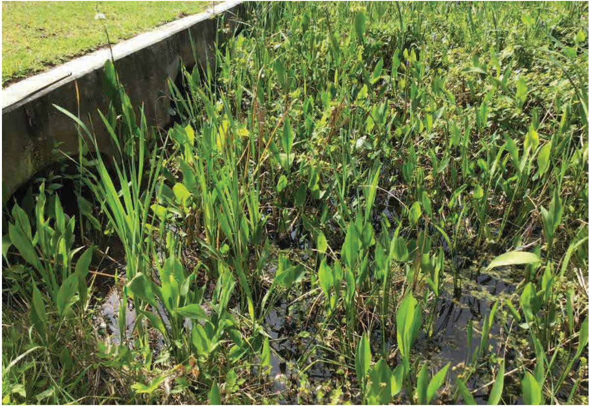
EX-A; Upstream End (West)
