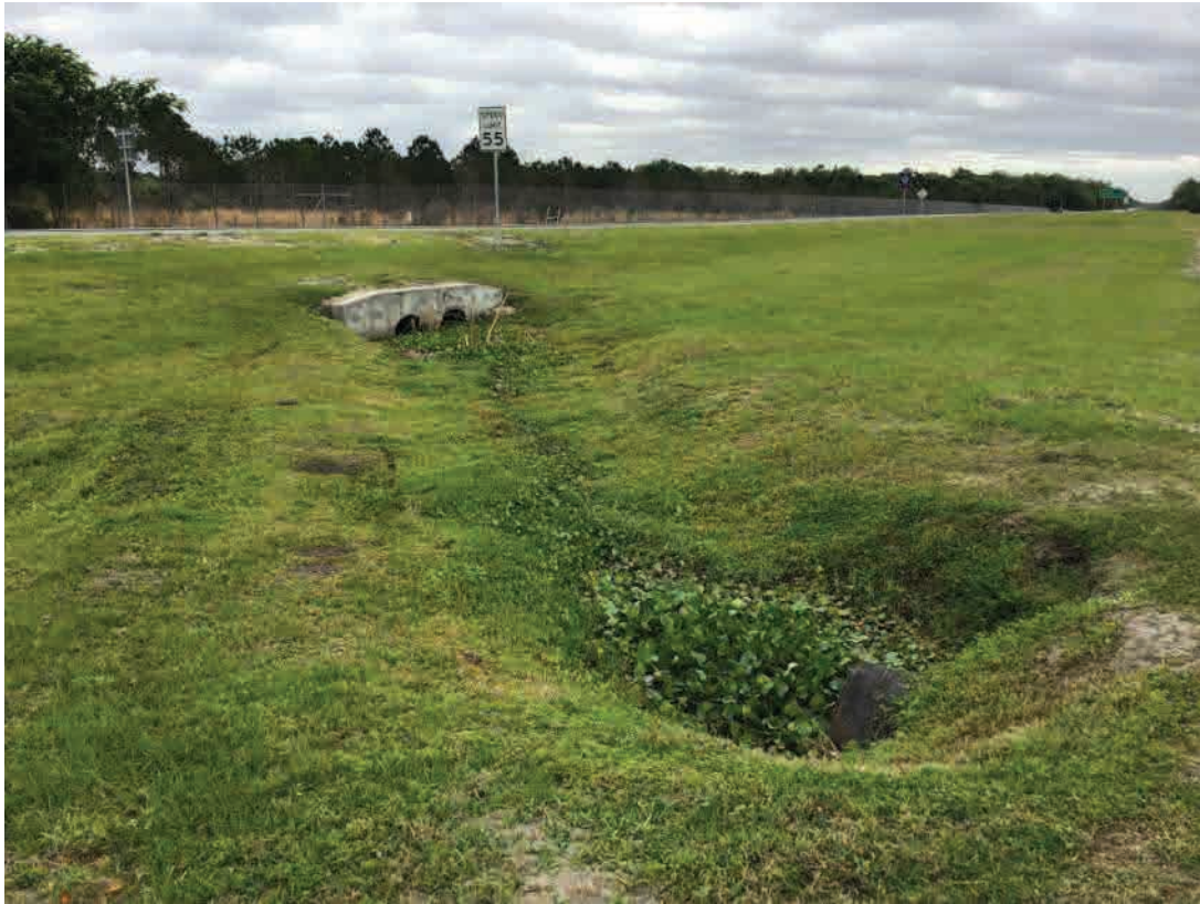
EX-CD-6; Upstream End (Southwest), Facing Northeast
