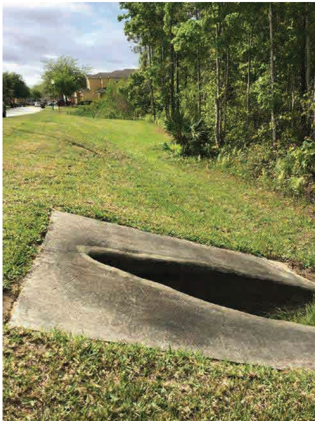
EX-E; Upstream End (West), Facing South
