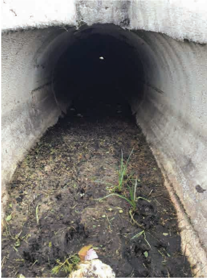
EX-CD-4A; Upstream End (Southwest), Facing Northeast
