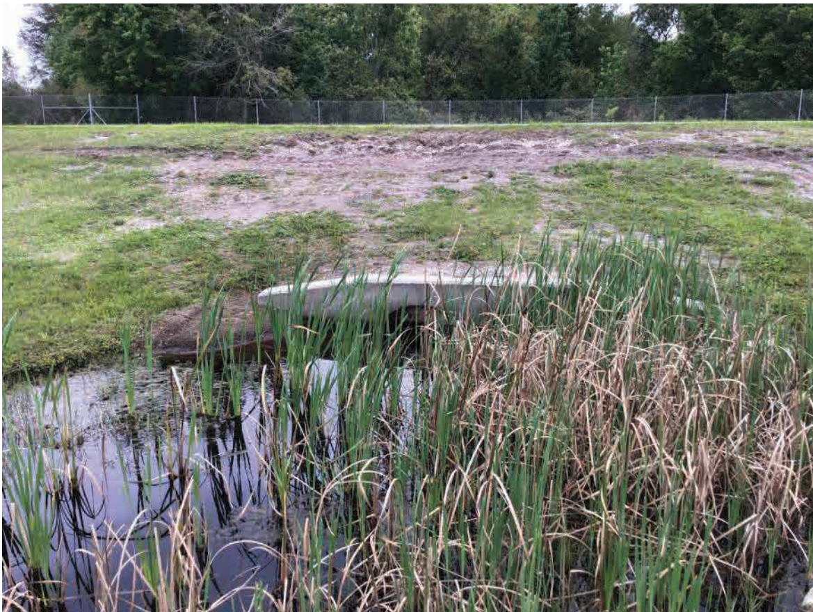
EX-CD-4; Upstream End (Southwest), Facing Northeast
