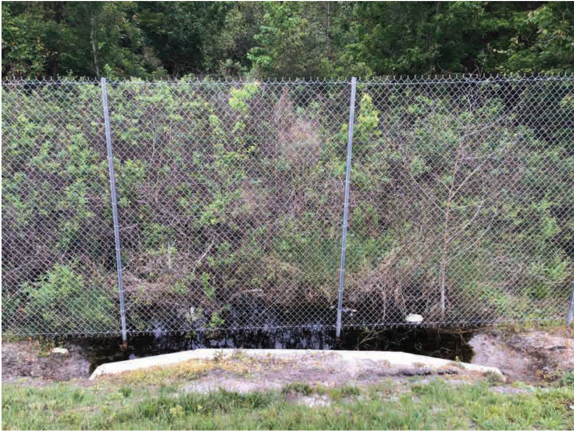
EX-CD-4; Downstream End (Northeast), Facing Northeast
