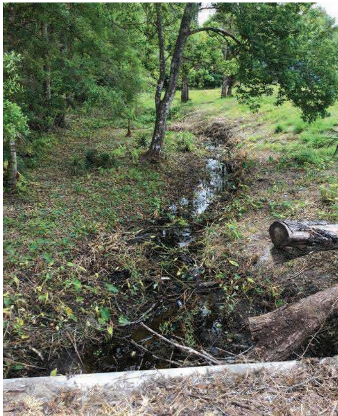
EX-C; Downstream End (Southeast), Facing Northeast
