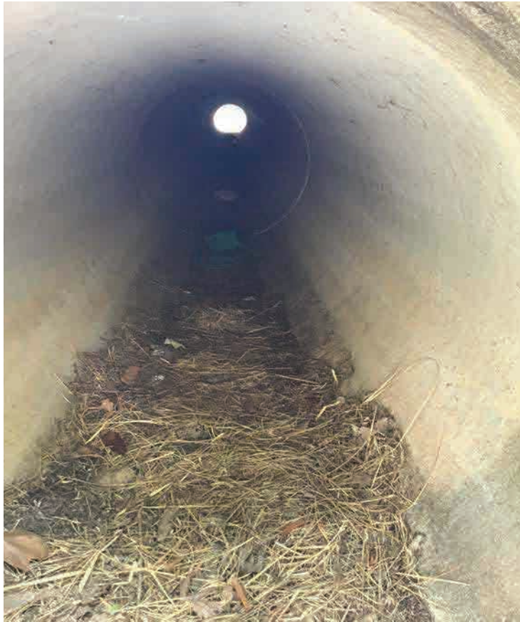
EX-E; Upstream End (West), Facing East
