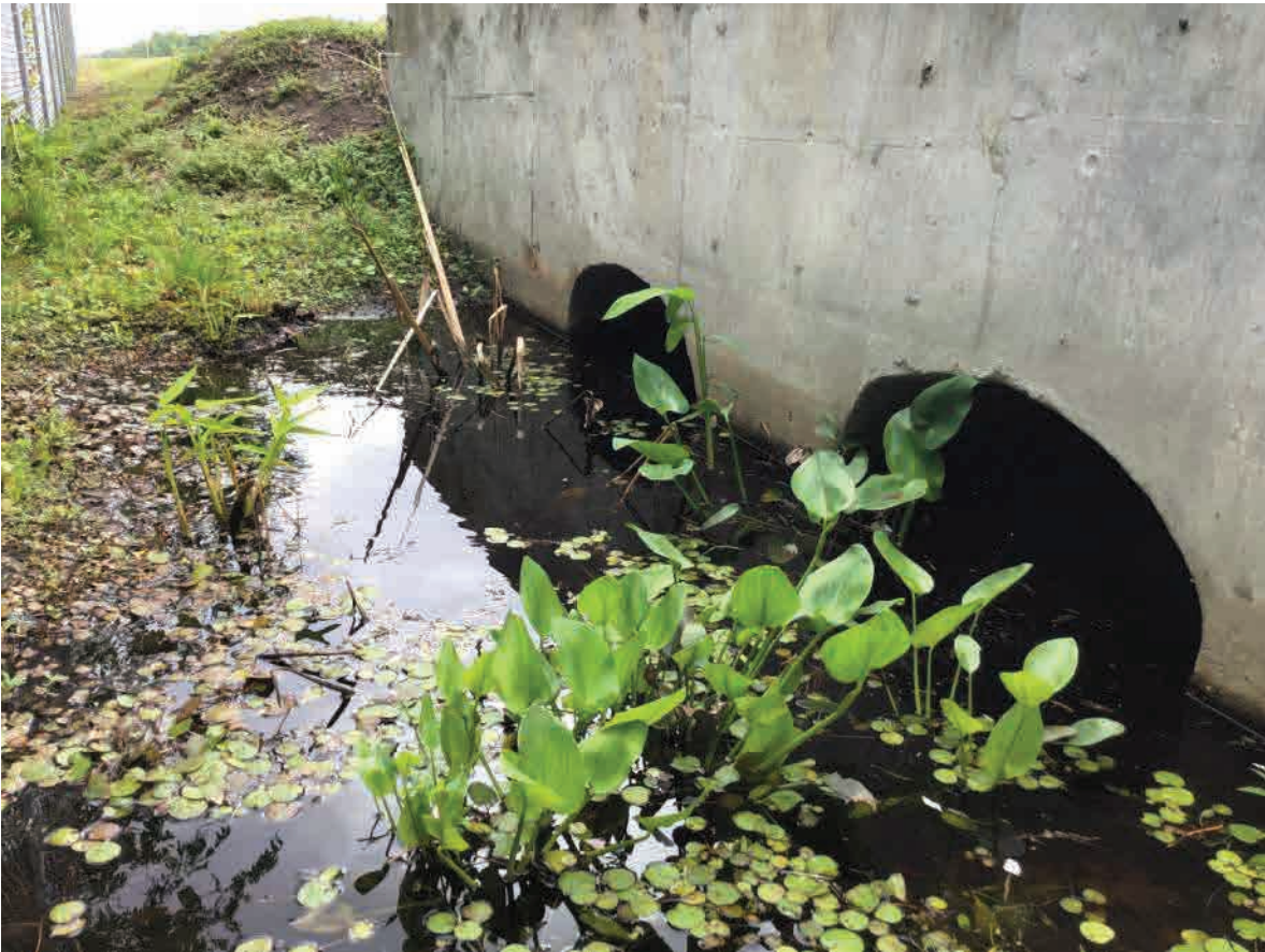
EX-CD-6; Downstream End (Northeast)
