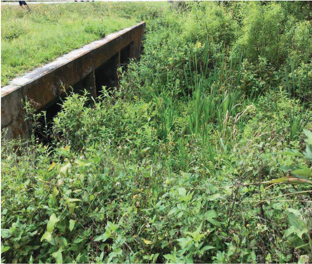
EX-N; Upstream (Northwest), Facing Southwest
