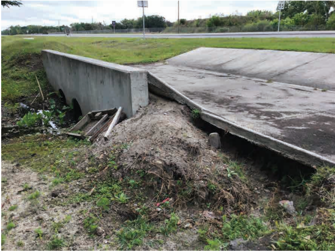
EX-CD-6; Downstream End (Northeast), Facing Southeast
