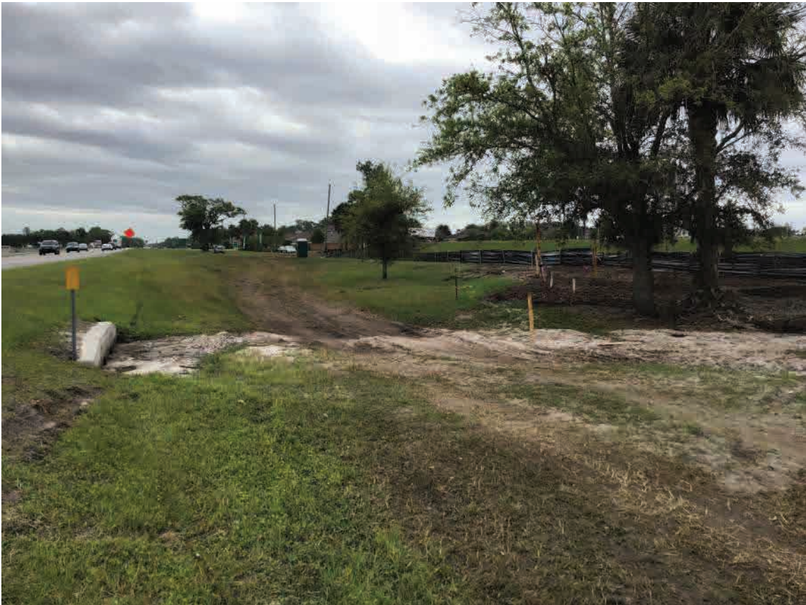
EX-CD-5; Upstream End (Southwest), Facing East
