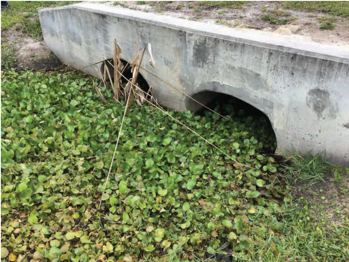
EX-CD-6; Upstream End (Southwest)
