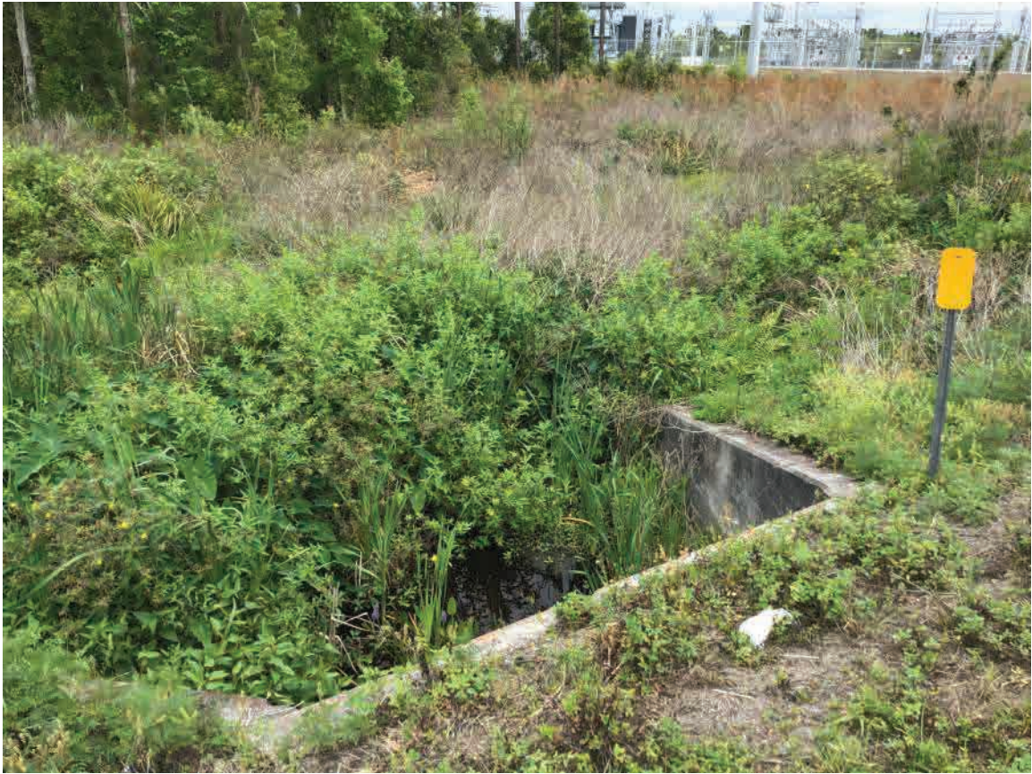
EX-C; Upstream End (Northwest), Facing North
