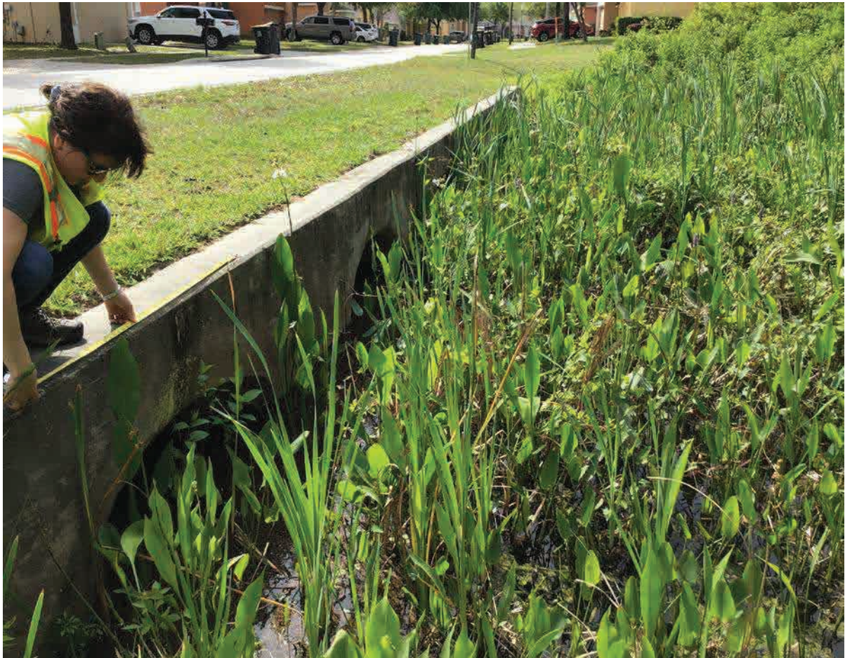
EX-A; Upstream End (West)
