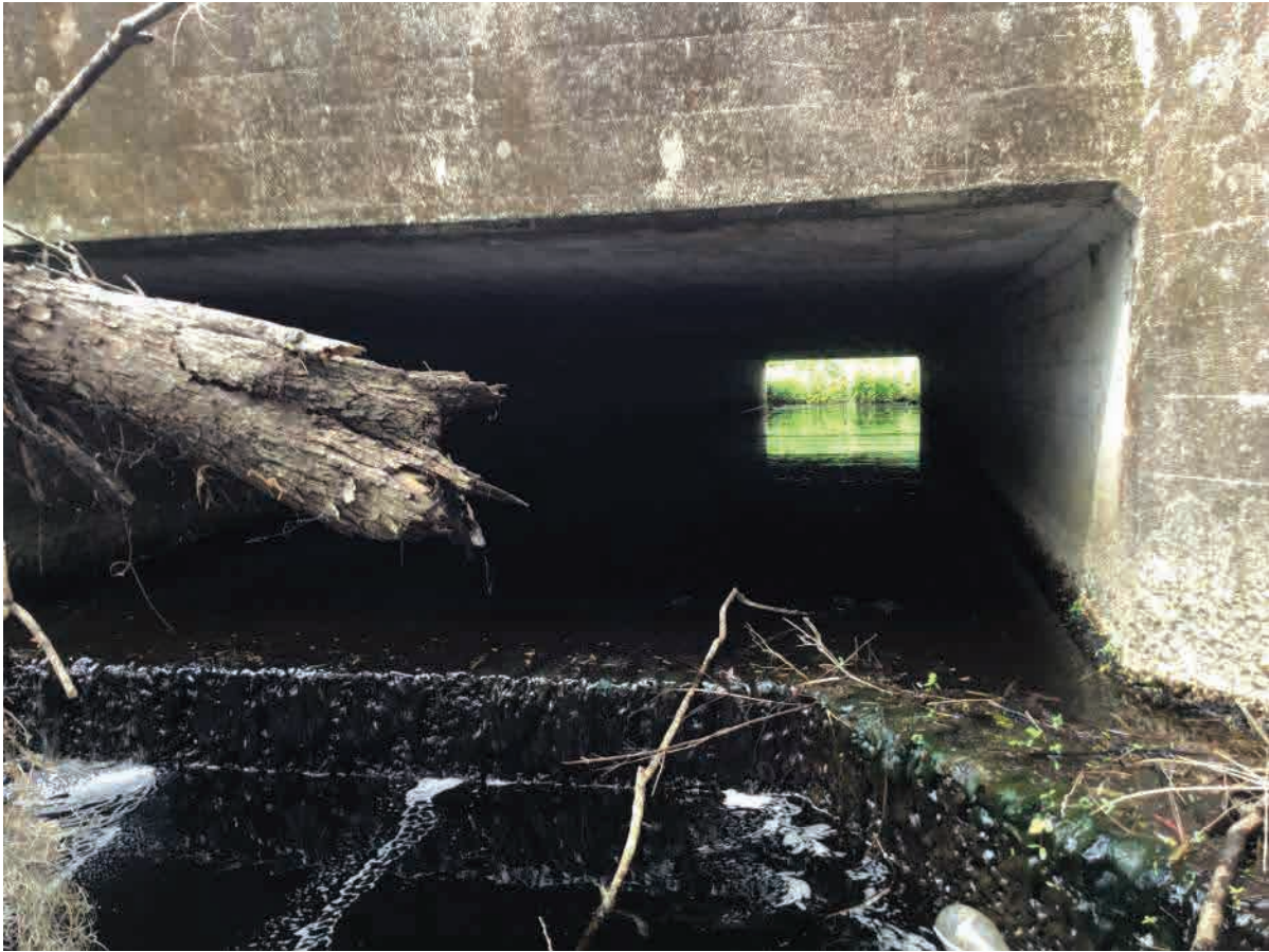
EX-C; Downstream End (Southeast), Facing Northwest
