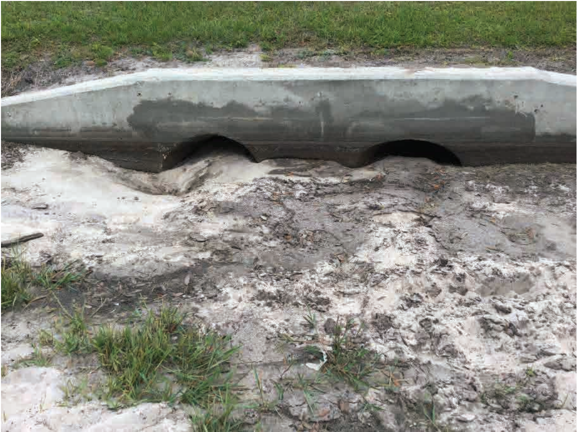
EX-CD-5; Upstream End (Southwest), Facing Northeast
