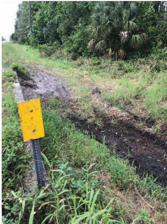
EX-CD-1; Upstream End (Northwest), Facing Southwest
