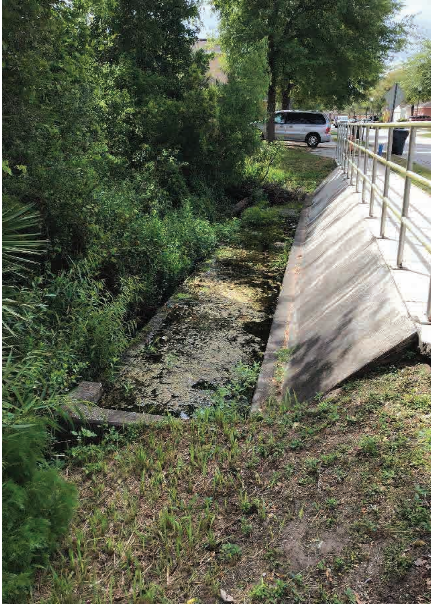
EX-A; Downstream End (East), Facing South
