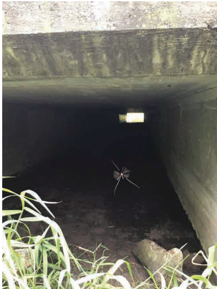
EX-CD-1; Upstream End (Northwest), Facing Southeast
