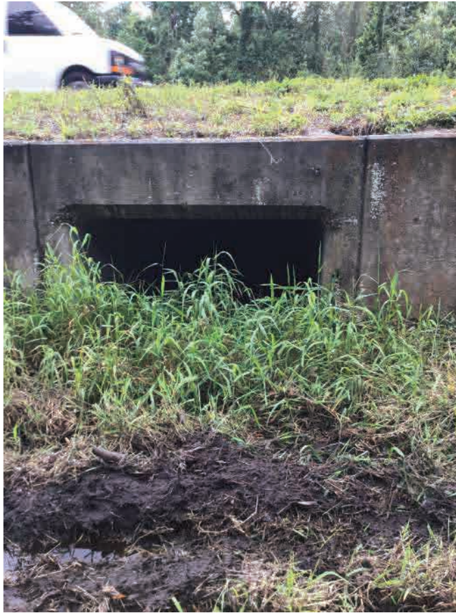
EX-CD-1; Upstream End (Northwest), Facing Southeast
