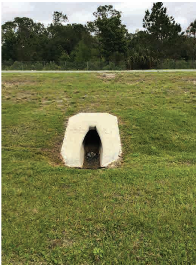
EX-CD-4A; Upstream End (Southwest), Facing Northeast
