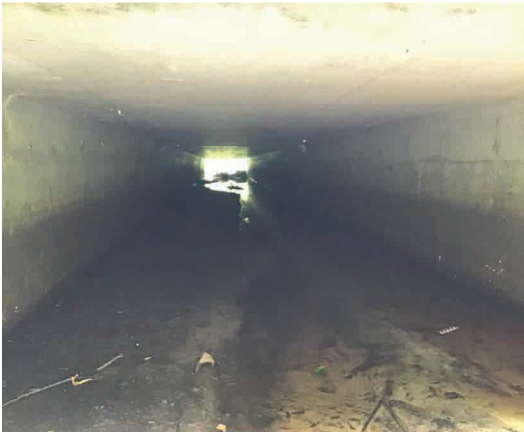
EX-D; Downstream End (Southeast), Facing Northwest
