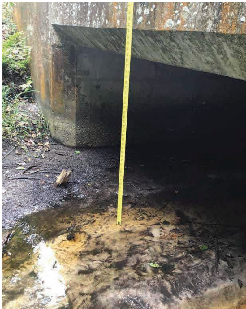
EX-D; Downstream End (Southeast)
