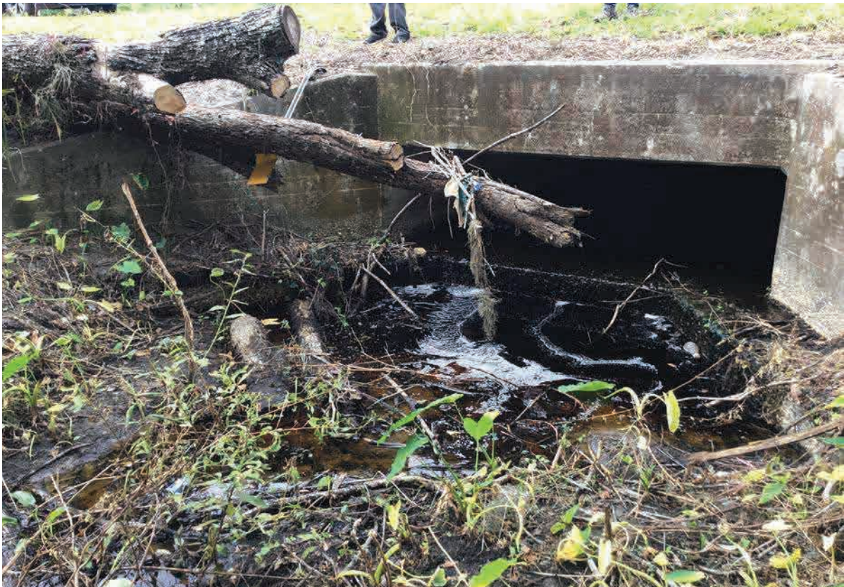
EX-C; Downstream End (Southeast), Facing Northwest
