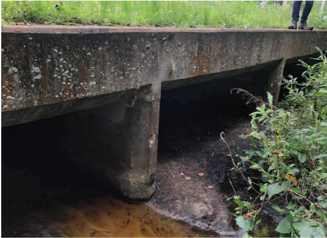
EX-D; Downstream End (Southeast)
