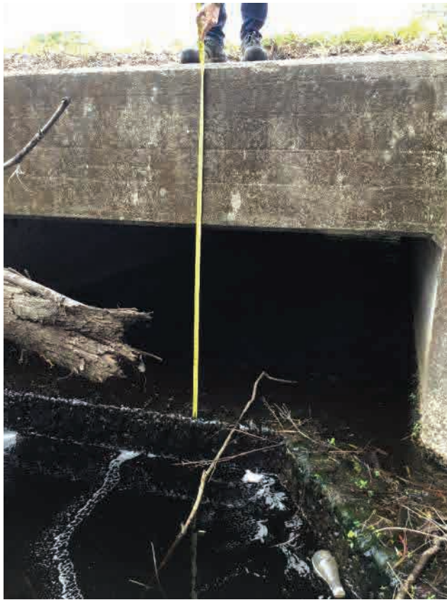
EX-C; Downstream End (Southeast), Facing Northwest
