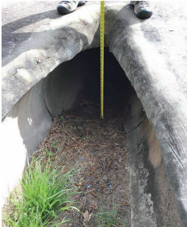
EX-E; Upstream End (West), Facing East
