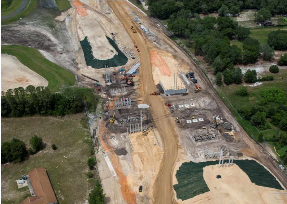
Wekiva Parkway Construction from Ponkan Road to Kelly Park Road
