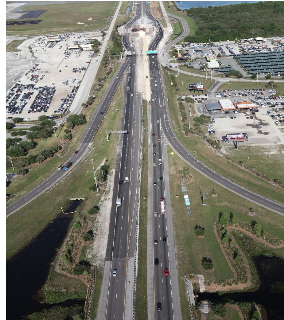
SR 528 Airport Mainline Toll Plaza Demolition
