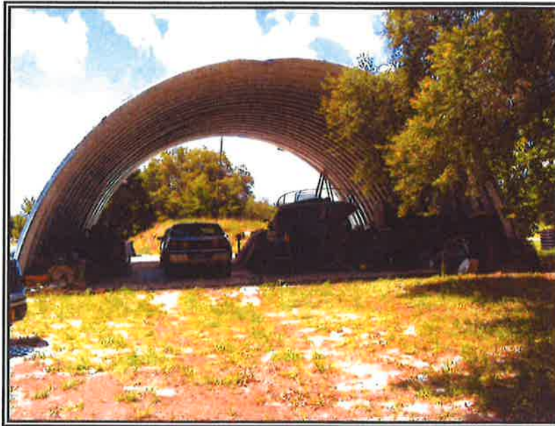
5. LOOKING SOUTH AT THE QUONSET HUT SHED
