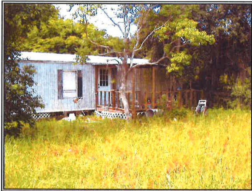
8. LOOKING SOUTHWEST AT THE ABANDONED MANUFACTURED HOME IN THE TAKING
