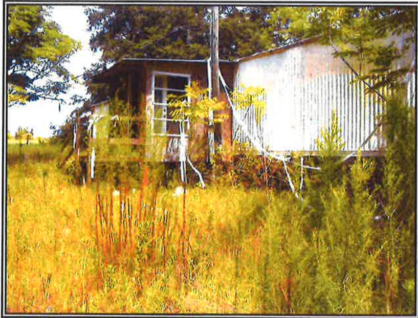
9. REAR VIEW OF THE OLD MANUFACTURED HOME
