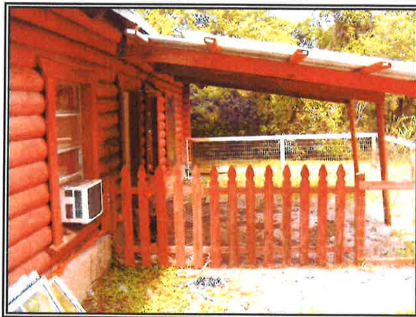
6. LOOKING WEST AT THE RESIDENCE
