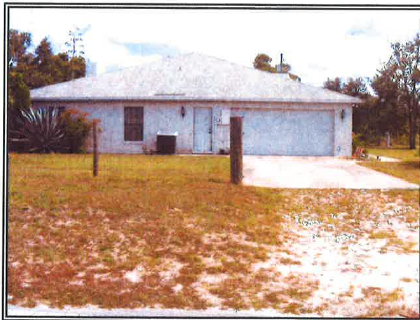
2. LOOKING NORTH AT THE DRIVE
