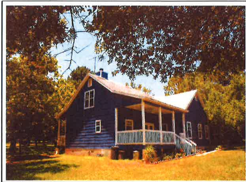
(8) Southwesterly (side & rear) view of the subject residence. Photograph taken by Thomas A. Riddle, MAI on July 30, 2014
