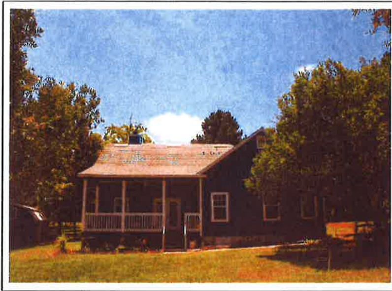
(7) Southerly (rear) view of the subject residence. Photograph taken by Thomas A. Riddle, MAI on July 30, 2014
