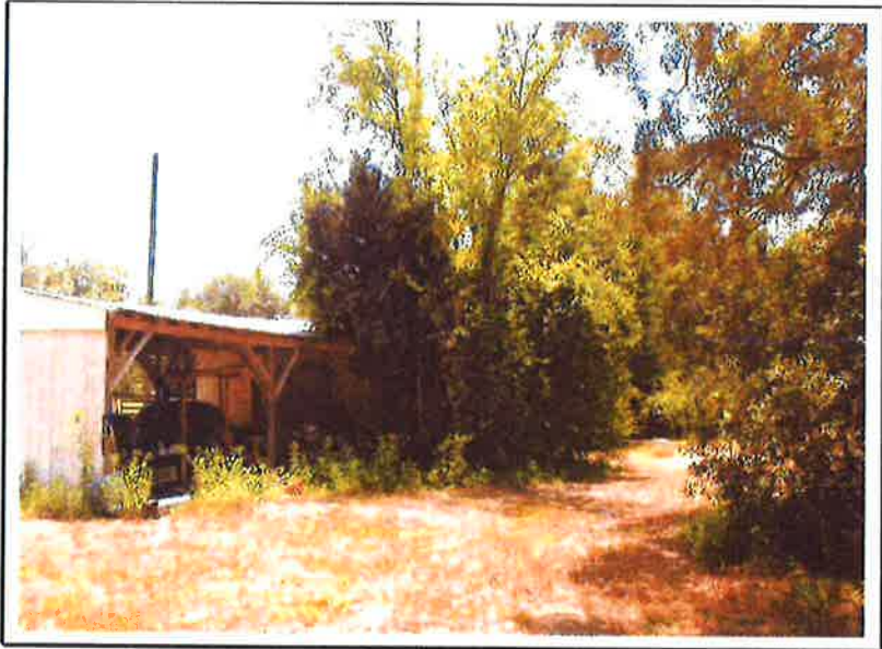
(6) Southwesterly (rear) view of the subject residence. Photograph taken by Thomas A. Riddle, MAI on July 30, 2014
