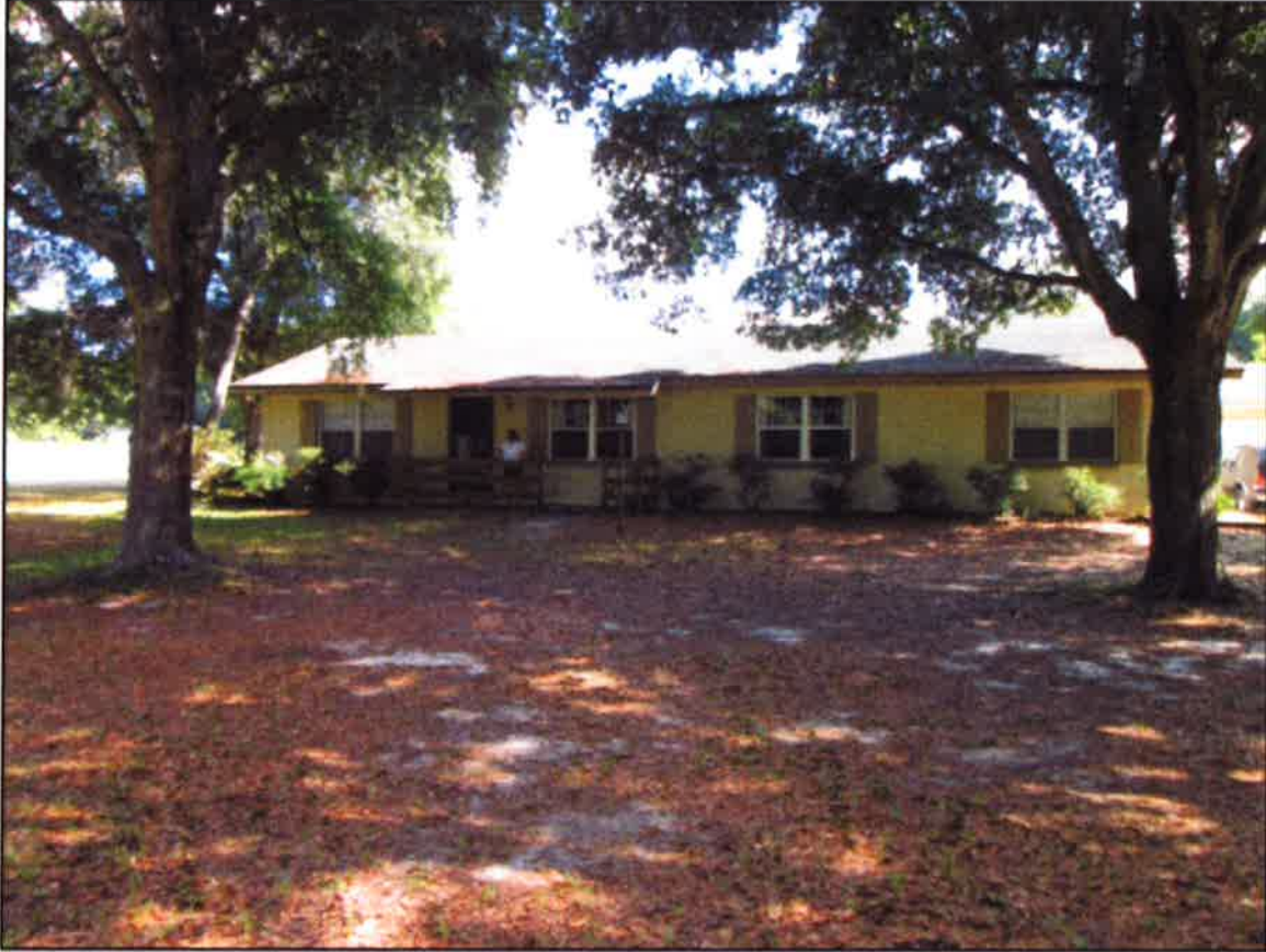
Wekiva Parkway - Section 429-206, Parcel 322 & Parcel 822 22521 Coronado Somerset Drive Sorrento, Florida
