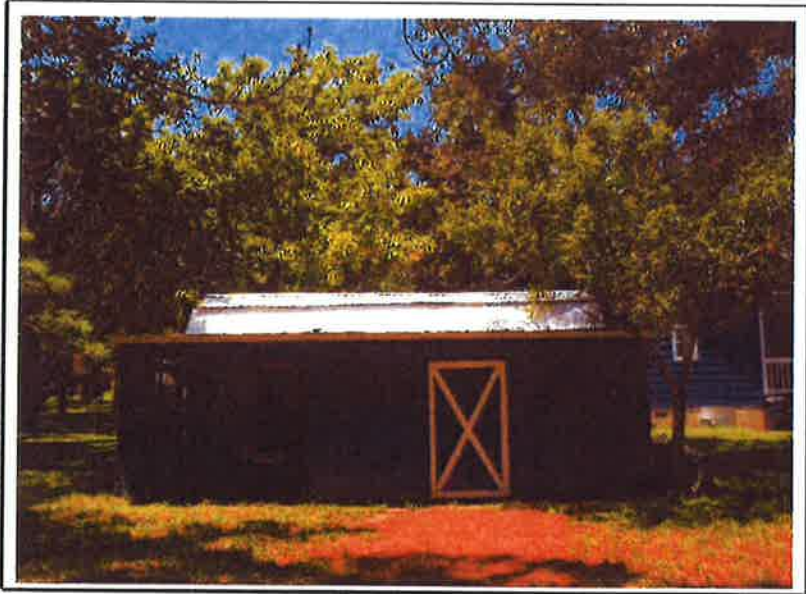
(10) View of the barn/stables. Photograph taken by Thomas A. Riddle, MAI on July 30, 2014
