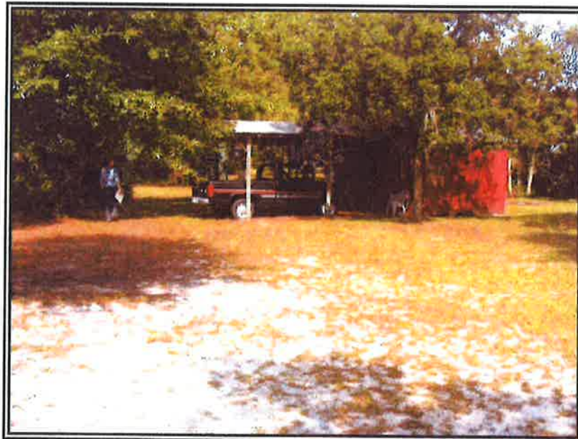
6. LOOKING WEST AT THE CARPORT/SHED
