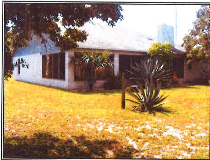
4. LOOKING SOUTHEAST AT THE RESIDENCE
