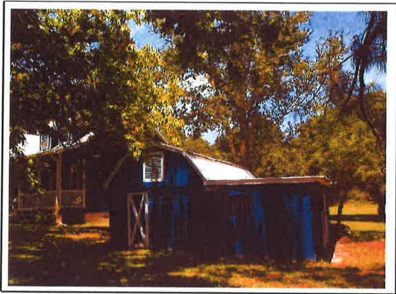
(9) View of the barn/stables. Photograph taken by Thomas A. Riddle, MAI on July 30, 2014
