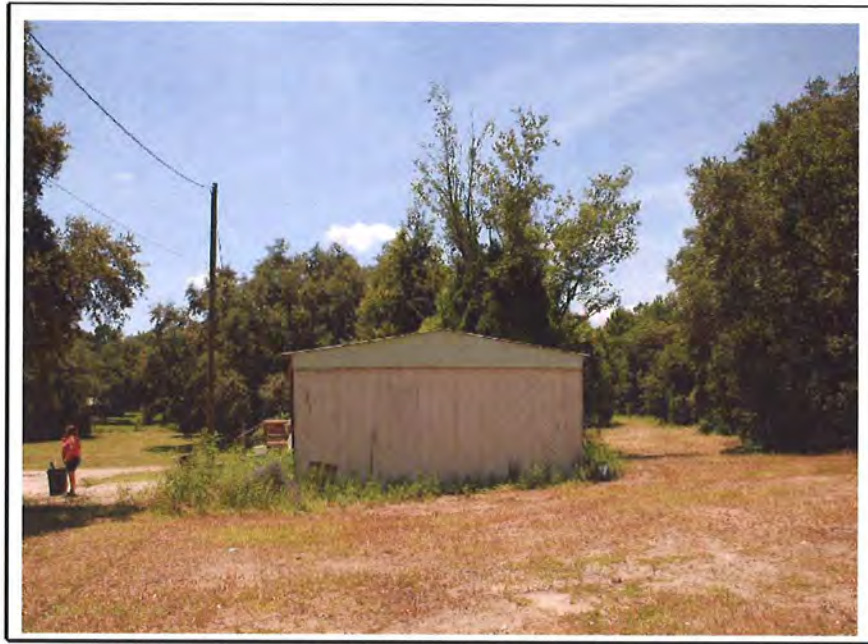
(5) Westerly (side) view of the subject residence. Photograph taken by Thomas A. Riddle, MAI on July 30, 2014
