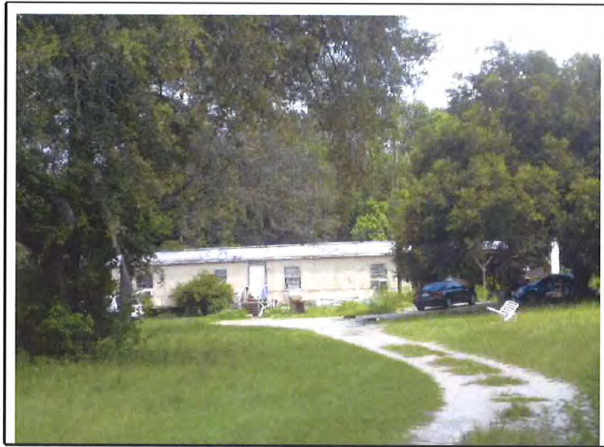
(3) Northerly view of the driveway leading to the subject property from Coronado Somerset Drive. Photograph taken by Thomas A. Riddle, MAI on July 21, 2015
