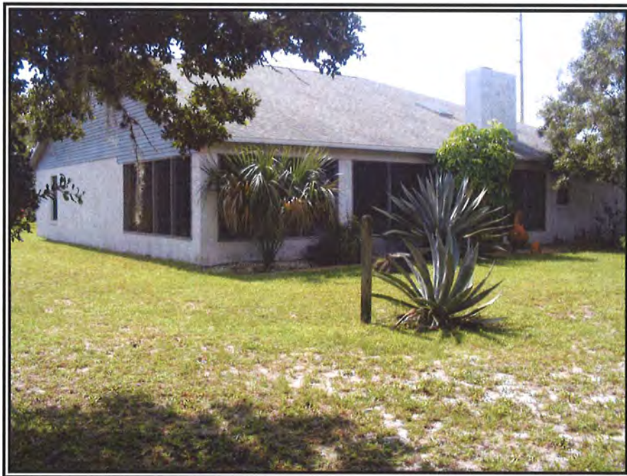
4. LOOKING SOUTHEAST AT THE RESIDENCE
