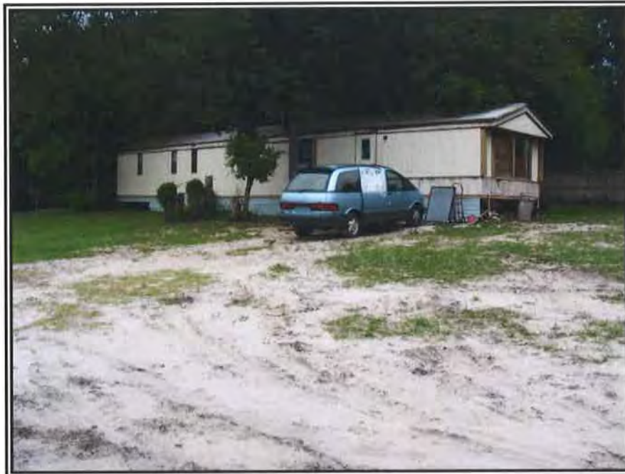
8. LOOKING NORTHWEST AT THE MANUFACTURED HOME
