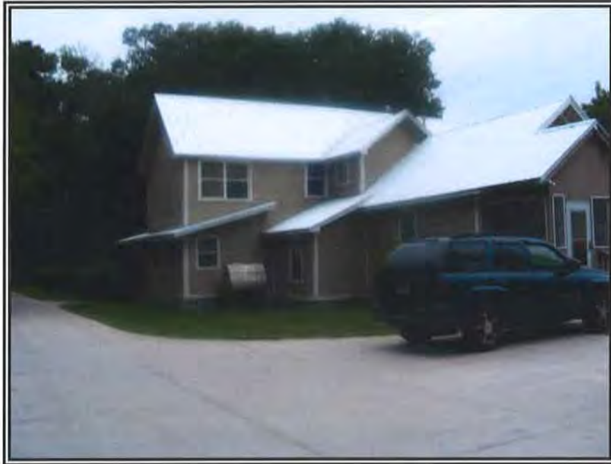
3. LOOKING SOUTHEAST AT THE SINGLE FAMILY RESIDENCE
