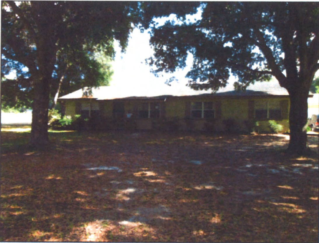
Wekiva Parkway - Section 429-206, Parcel 322 & Parcel 822 22521 Coronado Somerset Drive Sorrento, Florida
