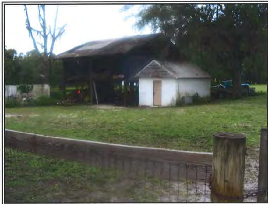
6. LOOKING SOUTHWEST AT THE SHED AND POLE BARN
