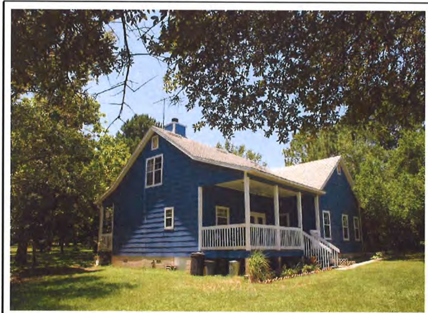
(8) Southwesterly (side & rear) view of the subject residence. Photograph taken by Thomas A. Riddle, MAI on July 30, 2014
