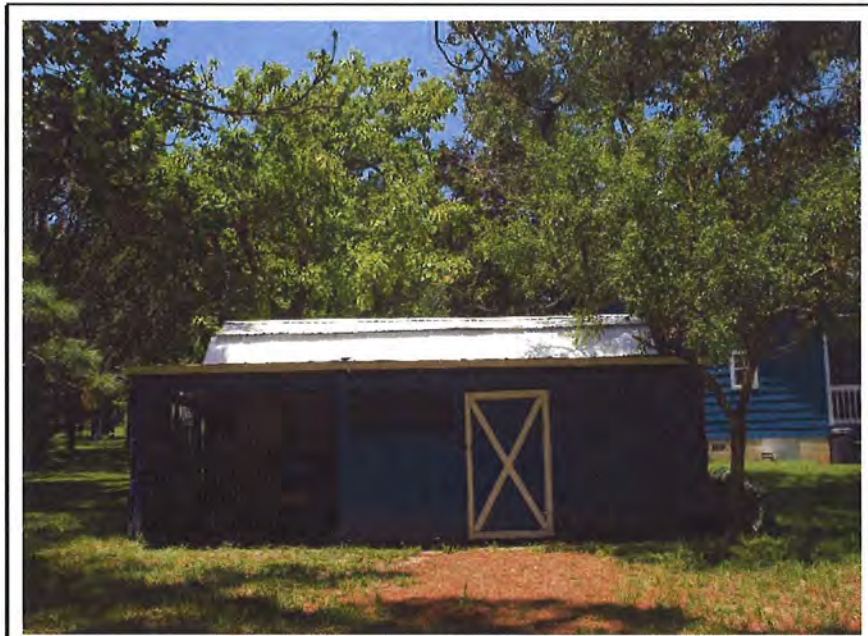
(10) View of the barn/stables. Photograph taken by Thomas A. Riddle, MAI on July 30, 2014
