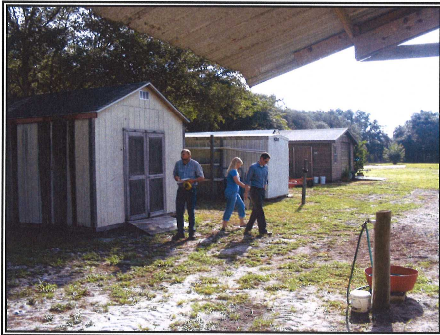
11. LOOKING NORTHEAST AT SOME OF THE SHEDS
