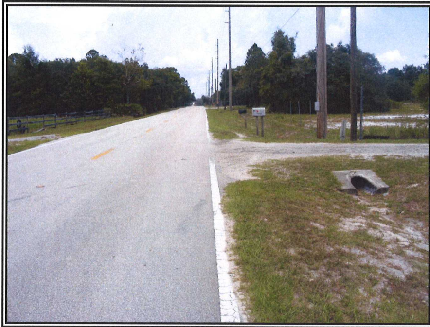
1. LOOKING EAST AT THE FRONTAGE ALONG ONDICH ROAD
