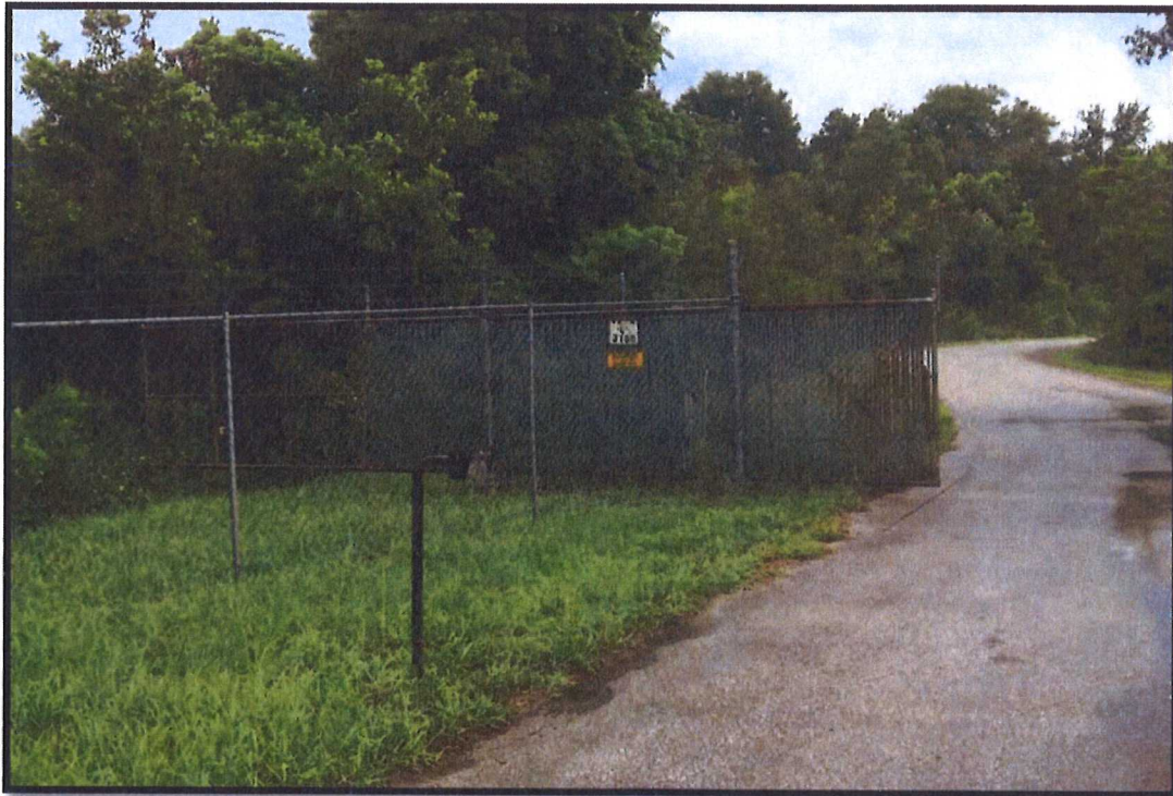
Southern view of rolling mechanical gate, asphalt drive and electronic keypad (Photo #4)
