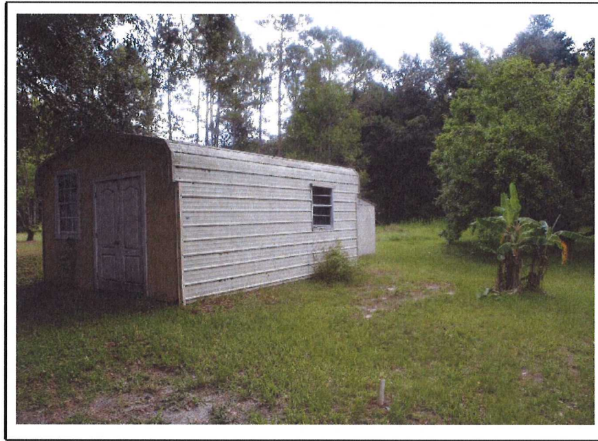
(9) View of one of the two shed buildings on the property. Photograph taken by Thomas A. Riddle, MAI on July 31, 2014
