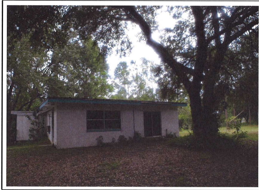
(7) Northerly view of the subject residence. Photograph taken by Thomas A. Riddle, MAI on July 31, 2014
