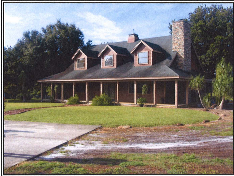
3. LOOKING SOUTHEAST AT THE RESIDENCE
