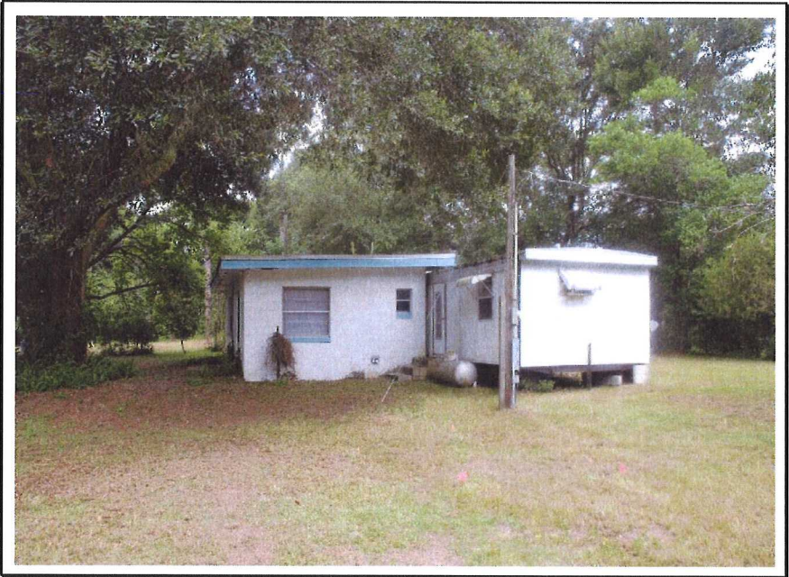
(6) Westerly view of the subject residence. Photograph taken by Thomas A. Riddle, MAI on July 31, 2014
