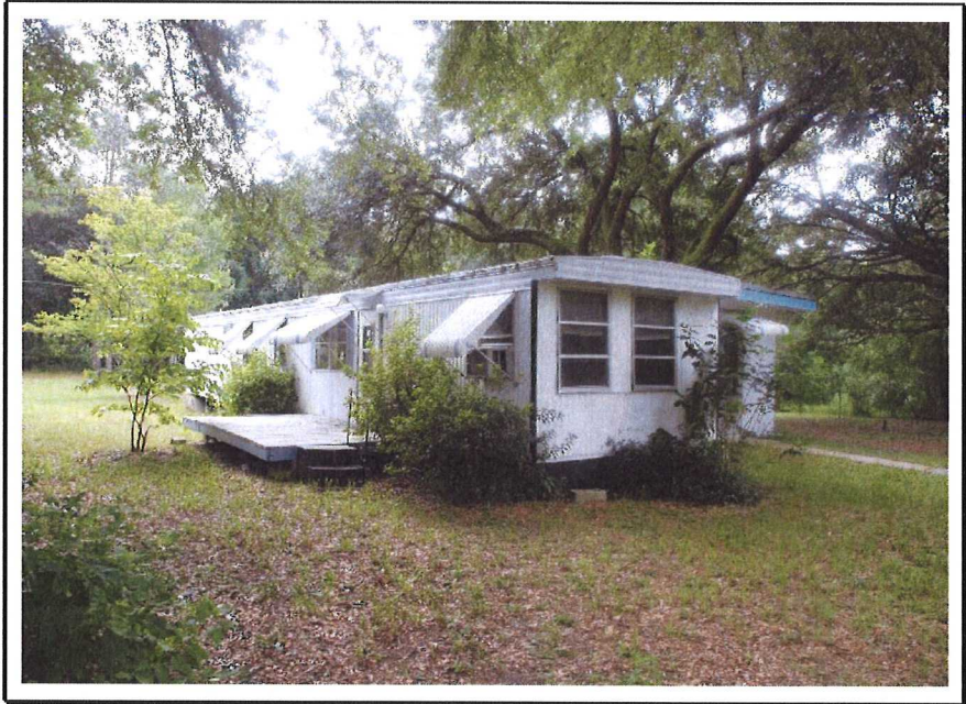
(4) Southeasterly view of the subject residence. Photograph taken by Thomas A. Riddle, MAI on July 31, 2014
