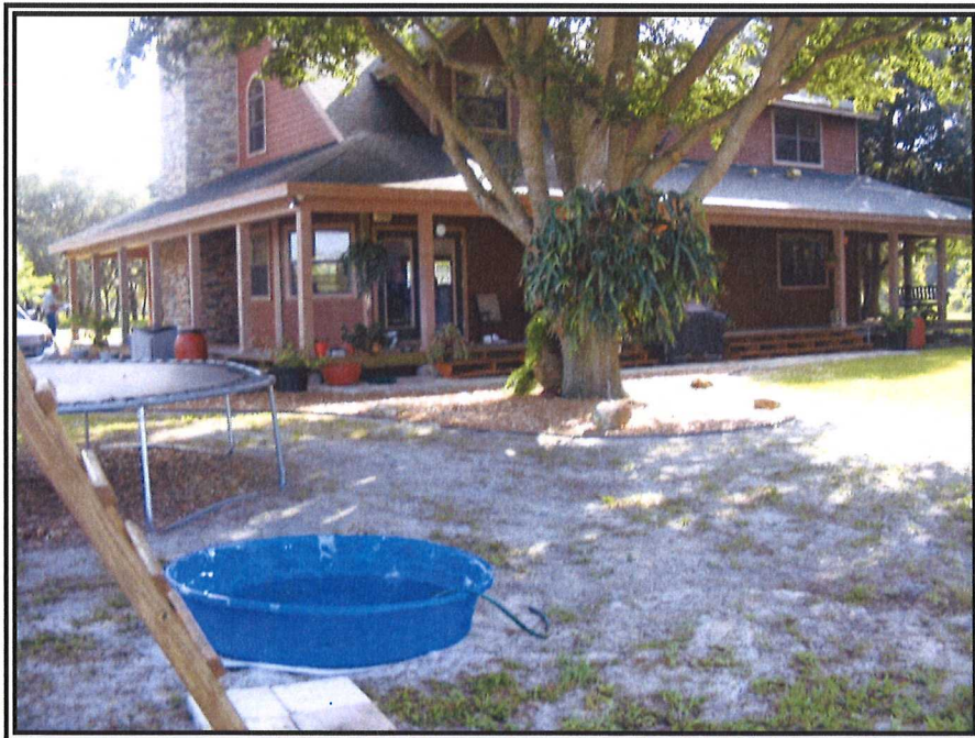
4. LOOKING NORTHEAST AT THE RESIDENCE
