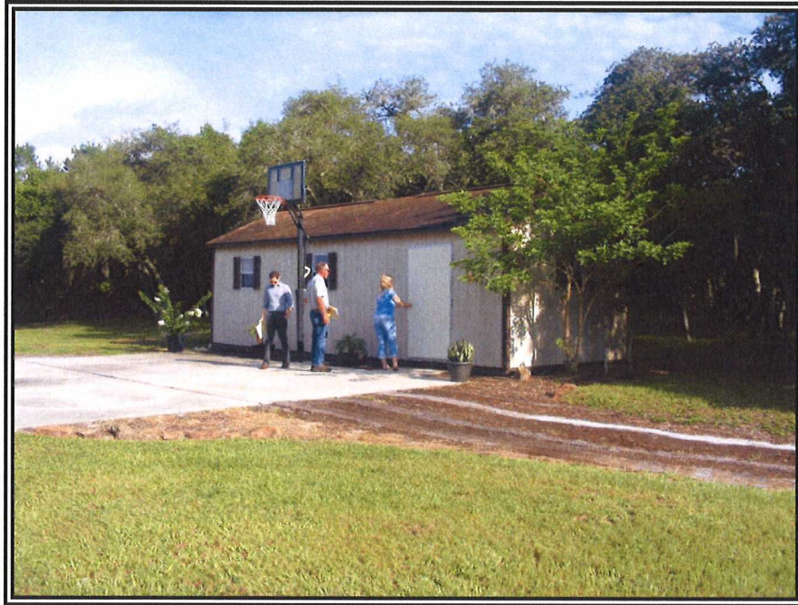
9. LOOKING NORTHWEST AT THE LARGE SHED
