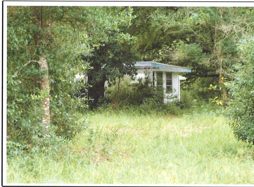
(11) Southeasterly view of the subject from Coronado Somerset Drive. Photograph taken by Richard K. MacMillan, MAI on August 27, 2015
