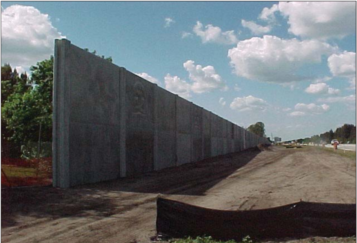
Typical 22 foot high noise barrier (under construction)
