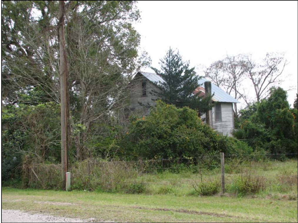
Exhibit C-5: Bock House, Facing Southeast
