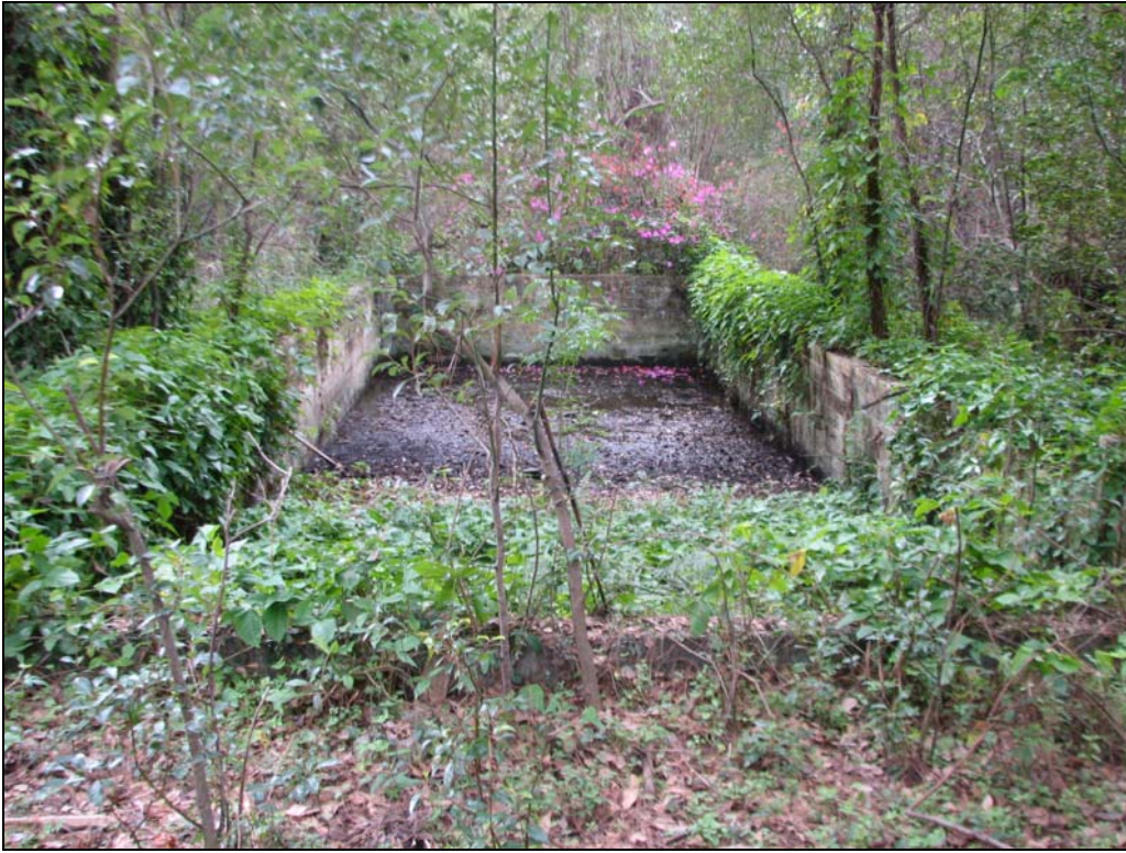
Exhibit C-14: Historic Swimming Pool at the Strite House, Facing South
