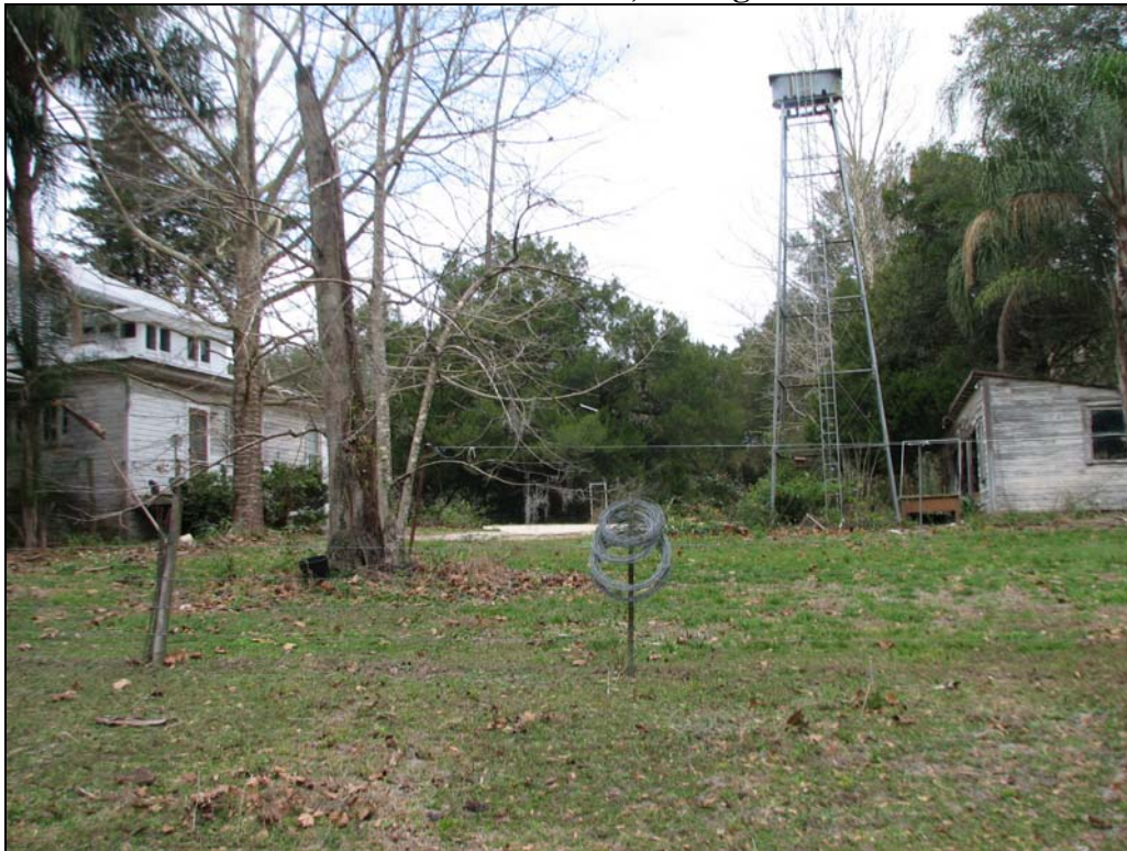
Exhibit C-13: Strite House and Ancillary Structures, Facing North
