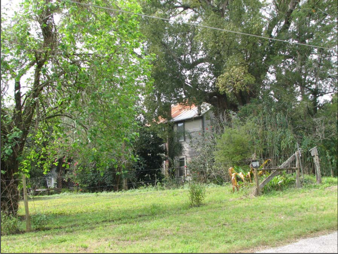
Exhibit C-7: Bock House and Associated Property from Boch Road, Facing Southwest
