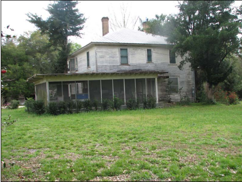
Exhibit C-12: Strite House, Facing Southeast
