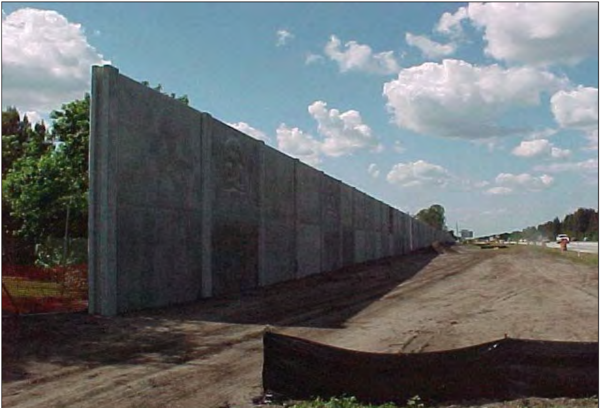
Typical 22 foot high noise wall (under construction)
