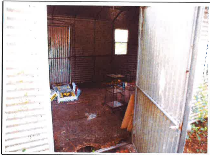
(14) Interior view of the storage shed. Photograph taken by Thomas A. Riddle, MAI on July 31, 2014
