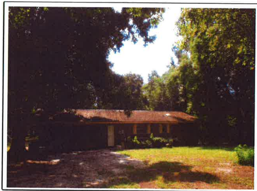
(6) Easterly (side) view of the subject residence. Photograph taken by Thomas A. Riddle, MAI on July 31, 2014
