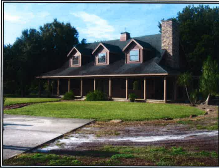
3. LOOKING SOUTHEAST AT THE RESIDENCE
