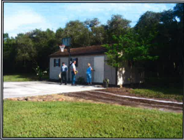
9. LOOKING NORTHWEST AT THE LARGE SHED
