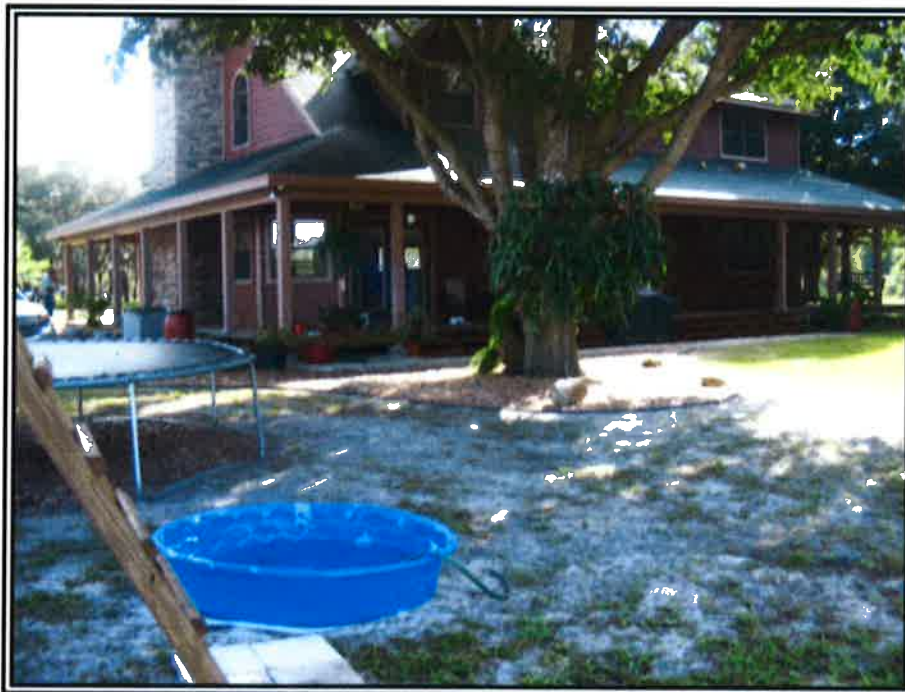
4. LOOKING NORTHEAST AT THE RESIDENCE
