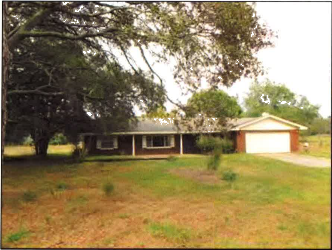
Wekiva Parkway - Section 429-206, Parcel 320 and Parcel 820 22437 Coronado Somerset Drive Sorrento, Florida
