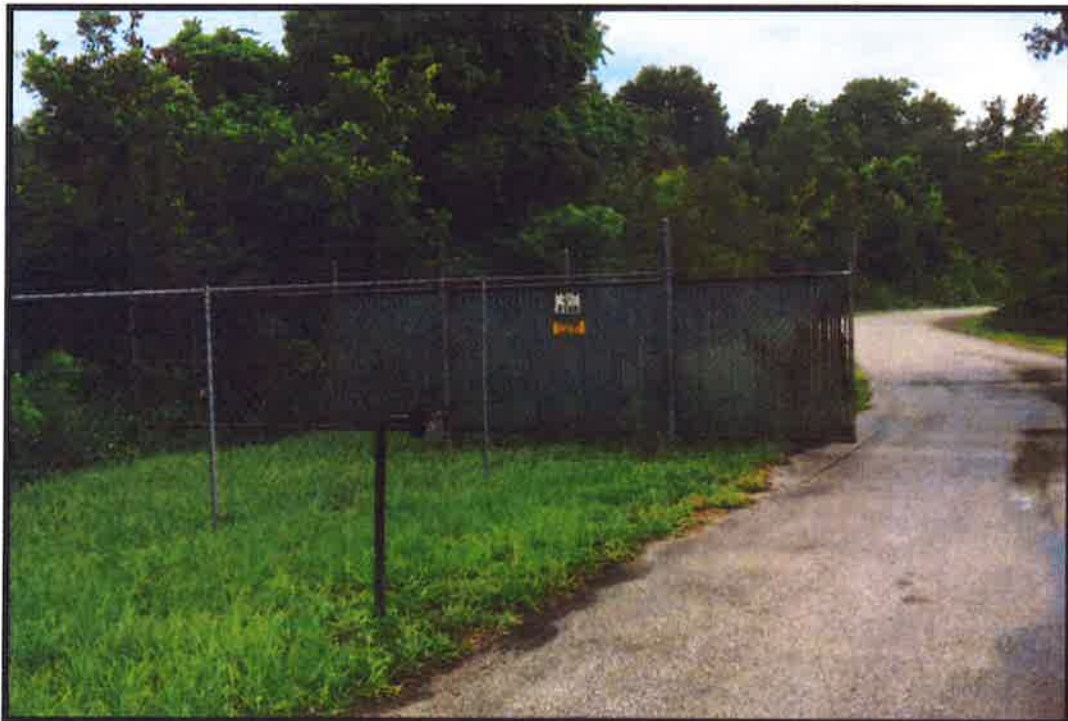
Southern view of rolling mechanical gate, asphalt drive and electronic keypad (Photo #4)
