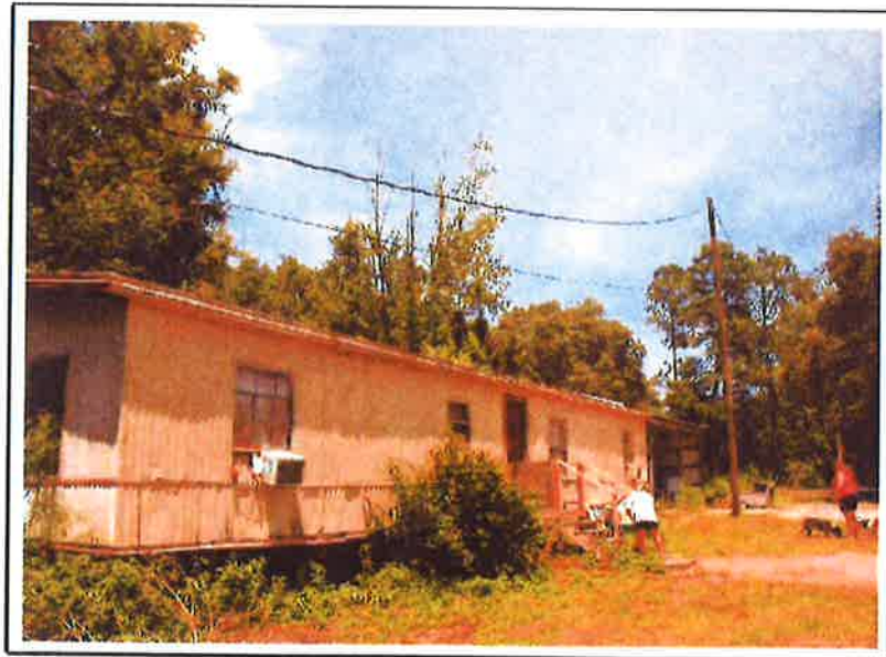
(8) Northeasterly (front) view of the subject residence. Photograph taken by Thomas A. Riddle, MAI on July 30, 2014
