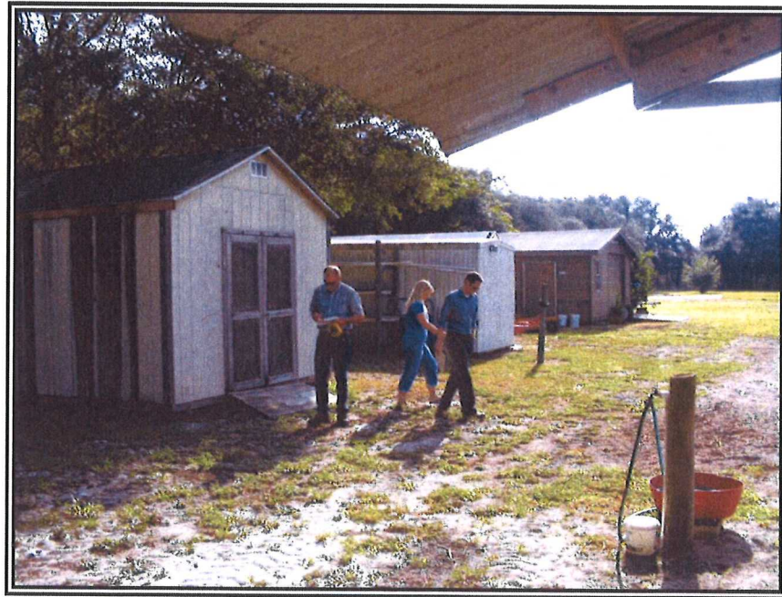
11. LOOKING NORTHEAST AT SOME OF THE SHEDS
