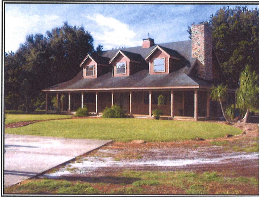
3. LOOKING SOUTHEAST AT THE RESIDENCE
