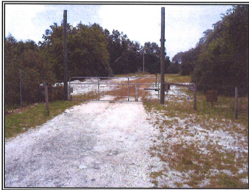
2. LOOKING SOUTH AT THE ACCESS ROAD FROM ONDICH ROAD
