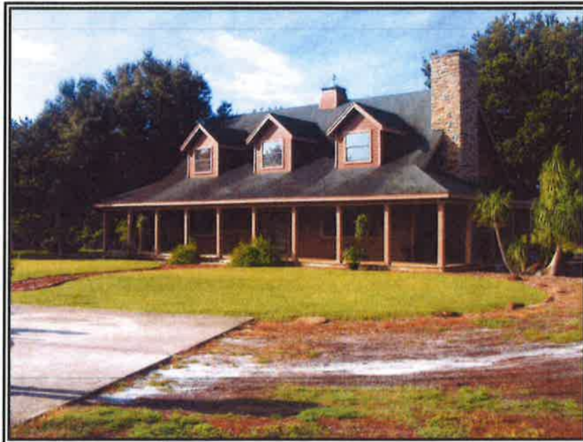
3. LOOKING SOUTHEAST AT THE RESIDENCE
