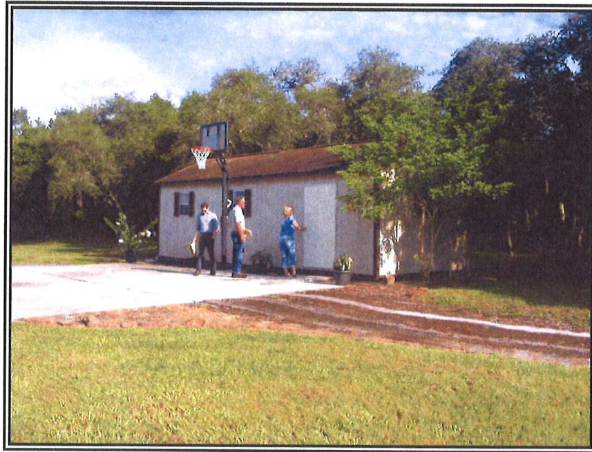
9. LOOKING NORTHWEST AT THE LARGE SHED
