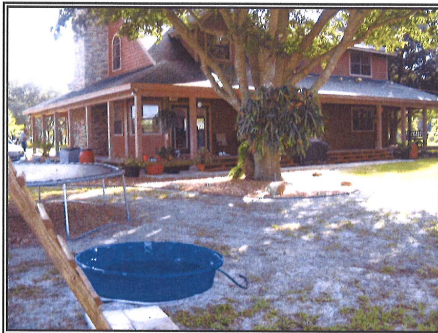
4. LOOKING NORTHEAST AT THE RESIDENCE
