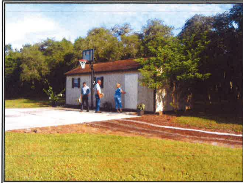
9. LOOKING NORTHWEST AT THE LARGE SHED
