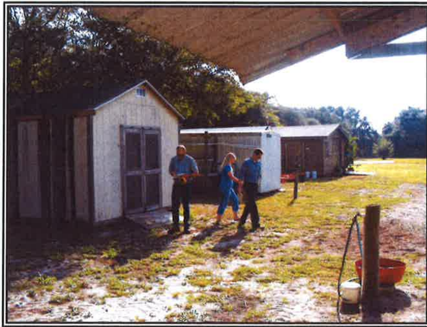
11. LOOKING NORTHEAST AT SOME OF THE SHEDS
