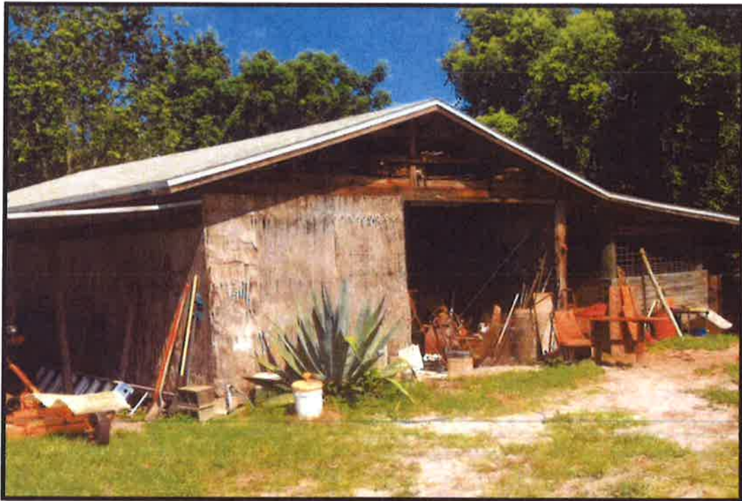
A view of the horse barn. (Photo 5)
