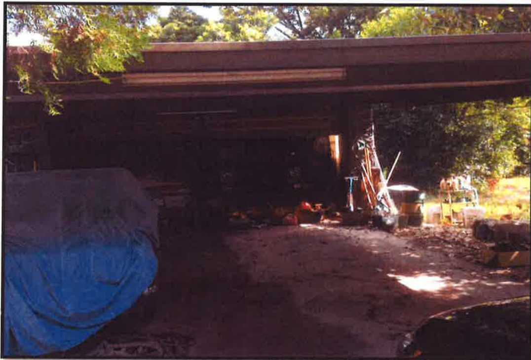
View of carport area. (Photo #2)
