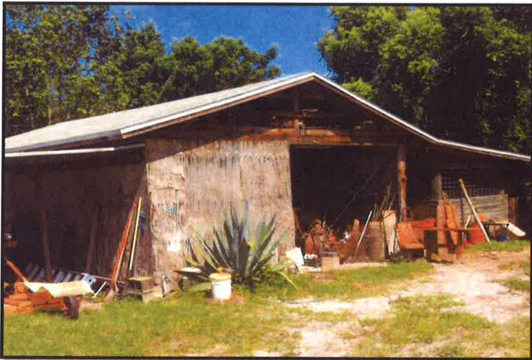
A view of the horse barn. (Photo 5)
