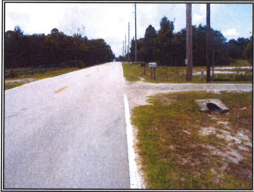
1. LOOKING EAST AT THE FRONTAGE ALONG ONDICH ROAD
