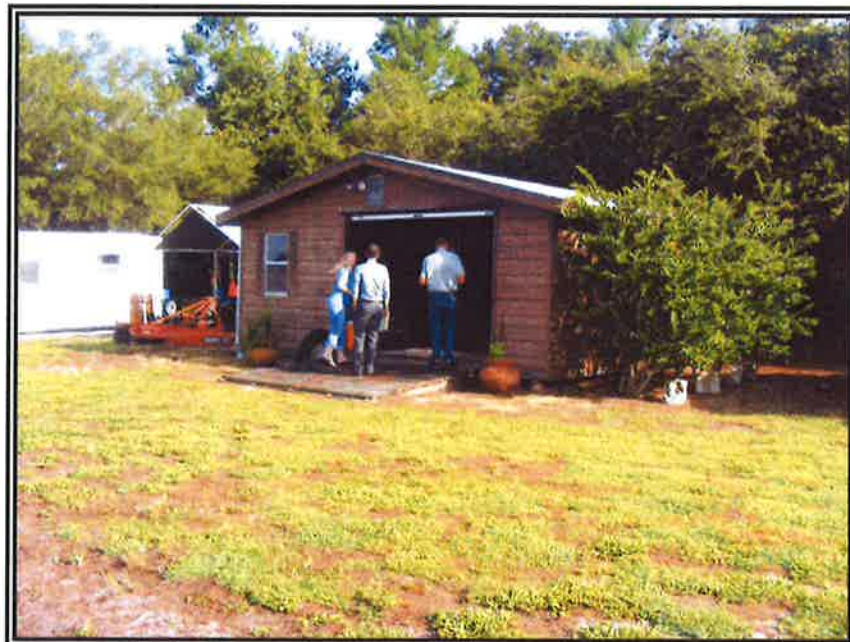
10. LOOKING NORTHWEST AT A SHED
