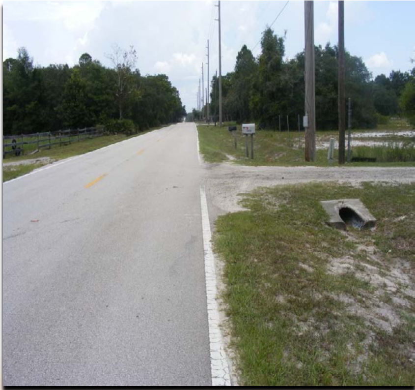
Looking East at the Frontage Along Ondich Road
