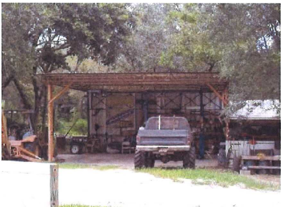
View of carport/ work shed (Photo Taken on July 11, 2013)
