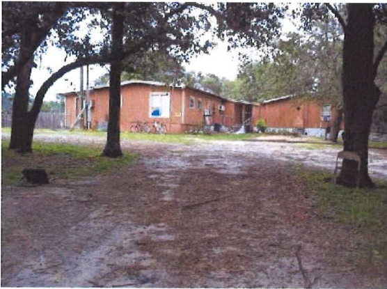
Southern view of larger manufactured home and gate (Photo Taken on July 11, 2013)
