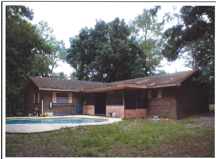
(8) Northwesterly (rear) view of the subject residence. Photograph taken by Thomas A. Riddle, MAI on July 31, 2014
