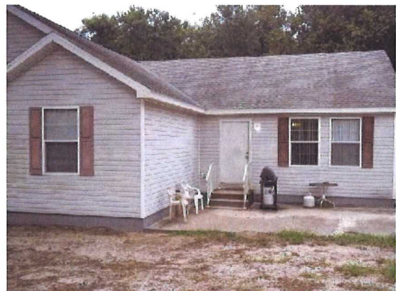
Western elevation of larger modular home (Photo Taken on July 11, 2013)
