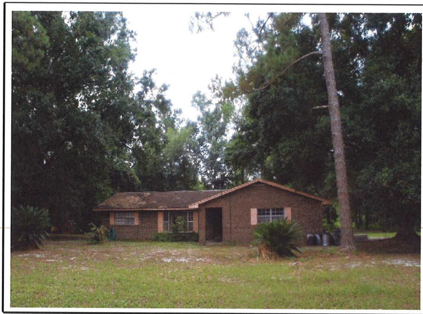
(5) Southerly (front) view of the subject residence. Photograph taken by Thomas A. Riddle, MAI on July 31, 2014
