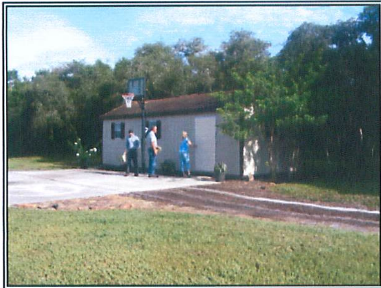
9. LOOKING NORTHWEST AT THE LARGE SHED
