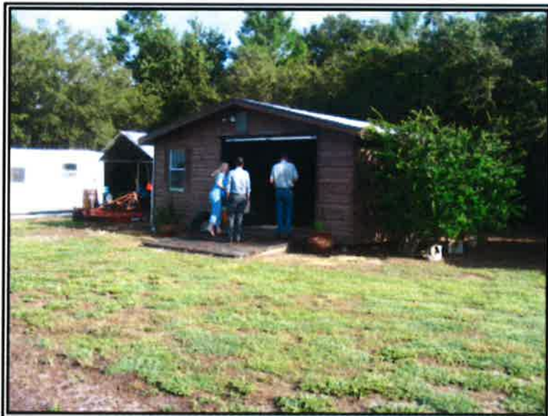
10. LOOKING NORTHWEST AT A SHED
