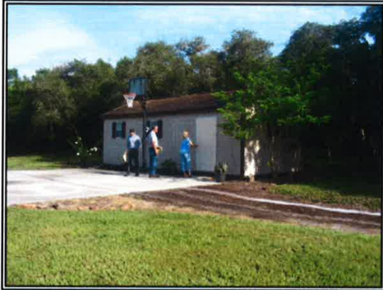
9. LOOKING NORTHWEST AT THE LARGE SHED
