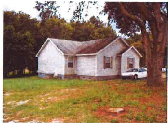
View of larger modular home, facing southeast (Photo Taken on July 11, 2013)
