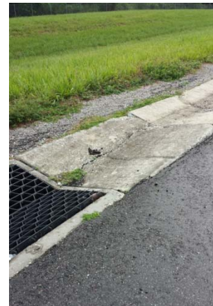
Picture 10 – Storm Drain Deficiency on SR 429 West Road NB Off Ramp
