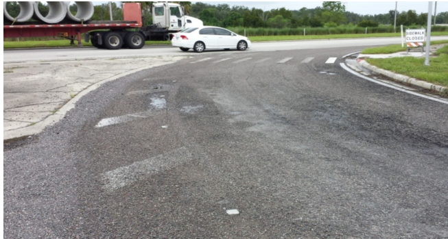
Picture 6 – Stripping on SR 417 SB Off Ramp to Boggy Creek Road
