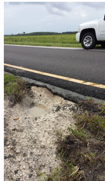
Picture 7 – Soil Shoulder Erosion at SR 417 Boggy Creek NB On Ramp
