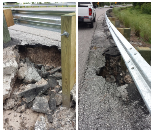
Picture 5– Paved Shoulder Erosion on SR 417 SB Off Ramp to WB SR 528
