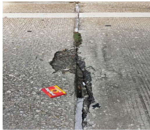
Photos 1 & 2 Critical Item Condition – Pavement Void at Plaza Apron
