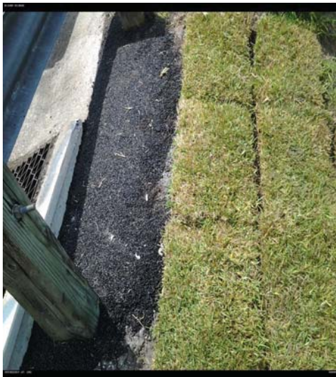
Photos 3 & 4 - Erosion backfilled, compacted, and sod replaced
