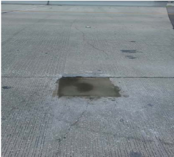
Photos 3 & 4 - Spall Repaired – Lee Vista Bridge Deck
