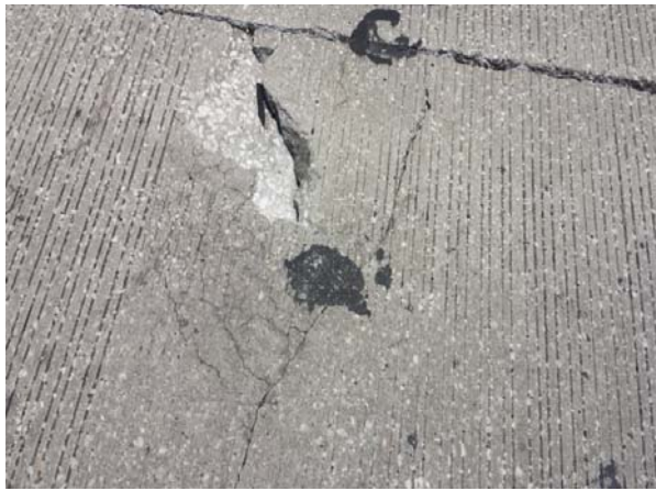
Photos 1 & 2 Critical Item Condition - Lee Vista Bridge Deck Spall
