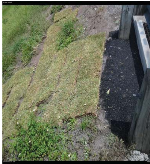
Photos 3 & 4 - Erosion backfilled, compacted, and sod replaced
