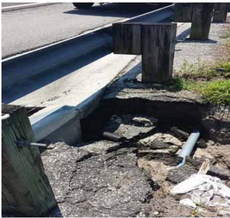
Photos 1 & 2 Critical Item Condition – Soil Shoulder Erosion
