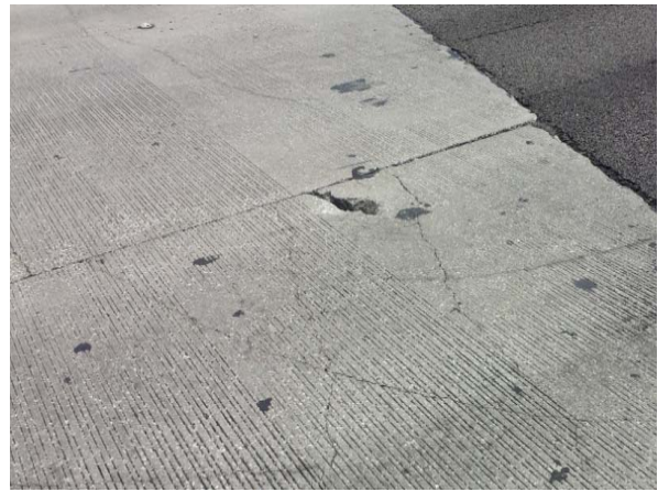
Photos 1 & 2 Critical Item Condition - Lee Vista Bridge Deck Spall
