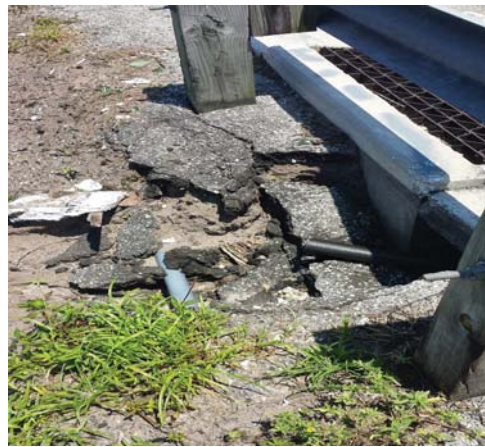
Photos 1 & 2 Critical Item Condition – Soil Shoulder Erosion
