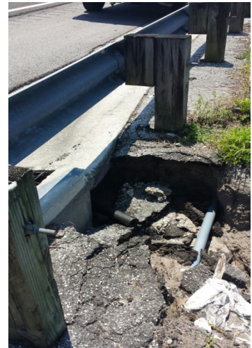
Picture 4 – SR 417 Soil Shoulder Erosion
