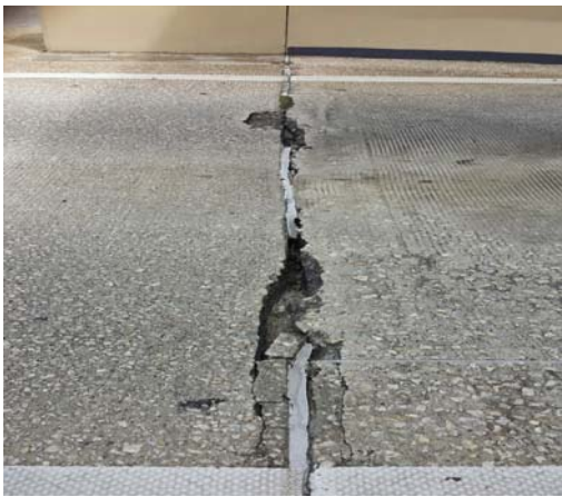
Photos 1 & 2 Critical Item Condition – Pavement Void at Plaza Apron
