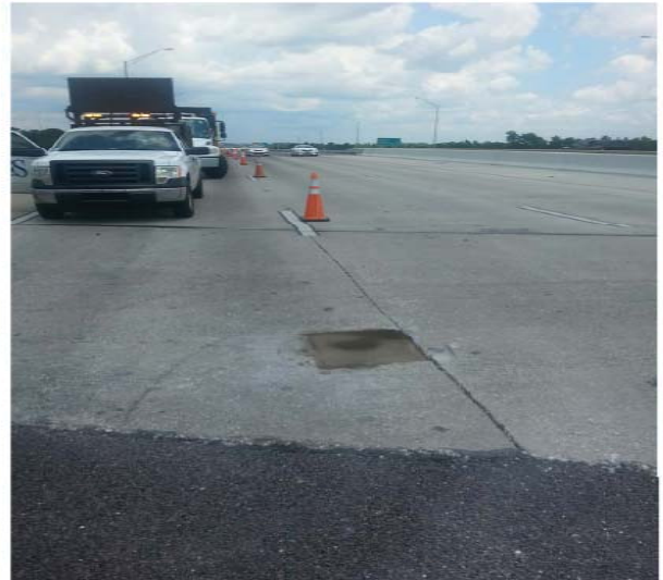
Photos 3 & 4 - Spall Repaired – Lee Vista Bridge Deck
