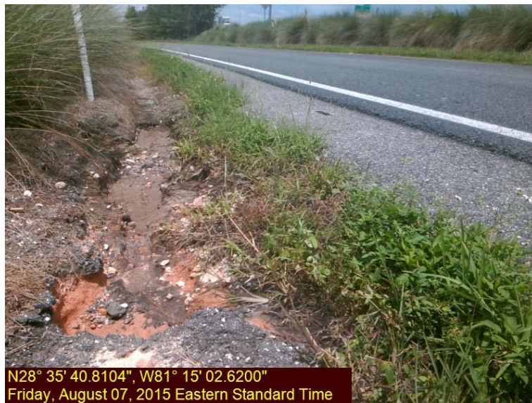
Photo 1 – Soil Shoulder Erosion
