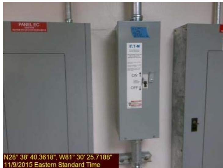
Photo 1 – UPS Shut off switch
