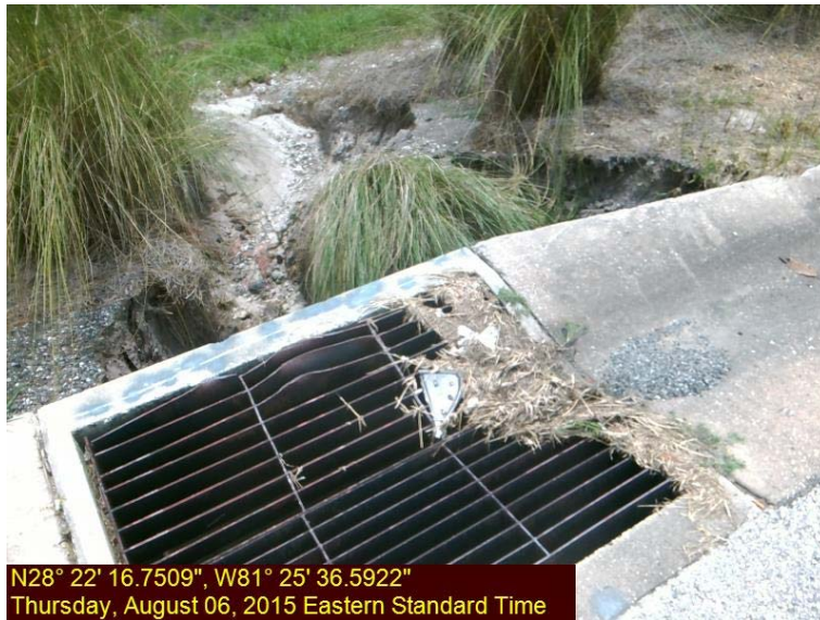
Photo 1 – Soil Shoulder Erosion
