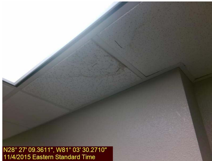
Photo 1 – Water intrusion in Hallway
