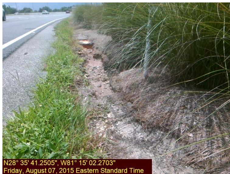
Photo 2 - Soil Shoulder Erosion
