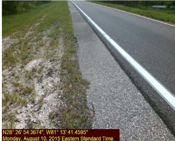
Photo 3 & 4 - Soil Shoulder Erosion
