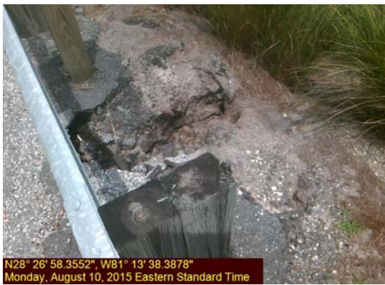
Photo 1 & 2– Soil Shoulder Erosion
