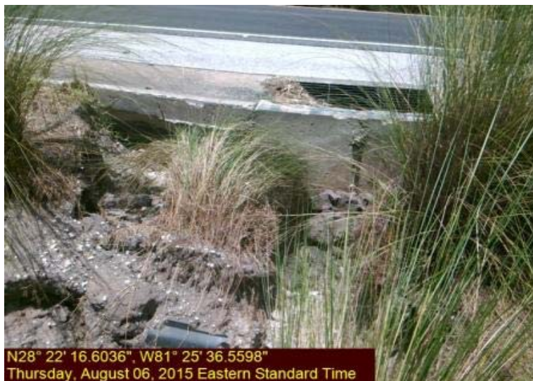
Photo 2 - Soil Shoulder Erosion
