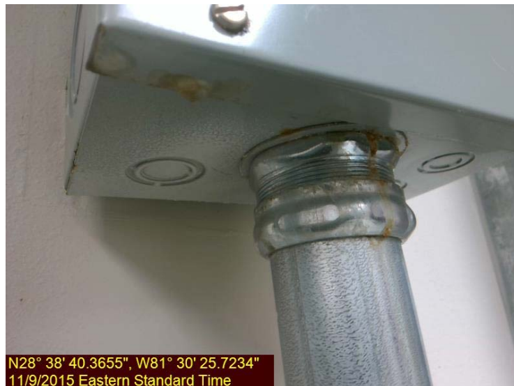
Photo 2 – Water dripping off UPS Shut off switch.
