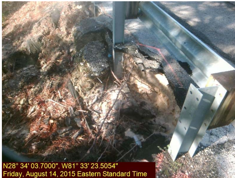
Photo 1 – Soil Shoulder Erosion
