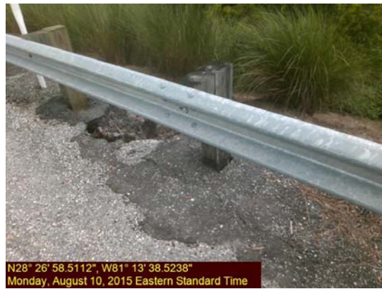
Photo 1 & 2– Soil Shoulder Erosion
