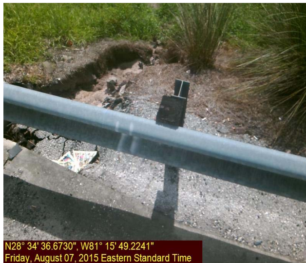
Photo 2 & 3 -Soil Shoulder Erosion
