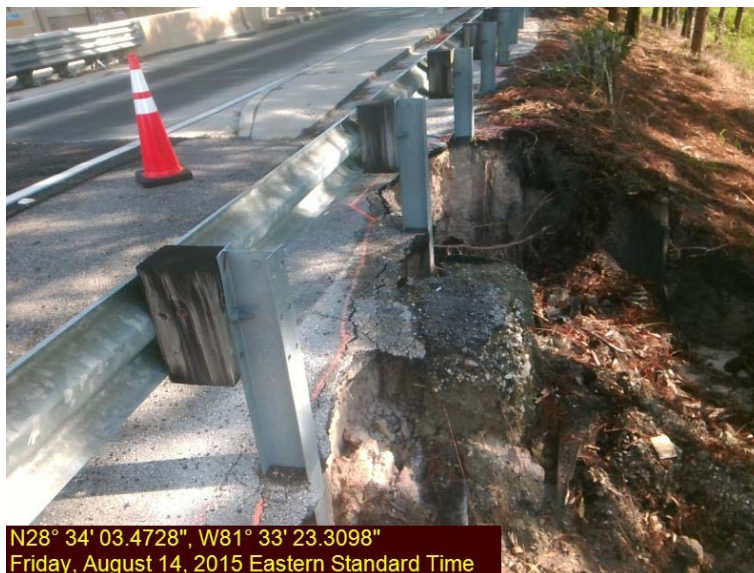
Photo 2 - Soil Shoulder Erosion
