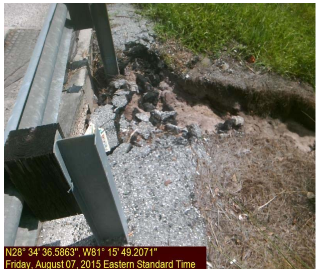
Photo 2 & 3 -Soil Shoulder Erosion
