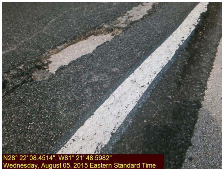
Photo 2 – Pothole - Subbase exposed
