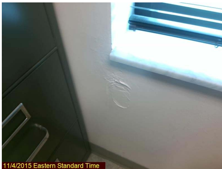
Photo 2 – Drywall damage from water intrusion (Supervisors office)
