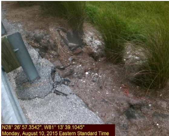
Photo 3 & 4 - Soil Shoulder Erosion
