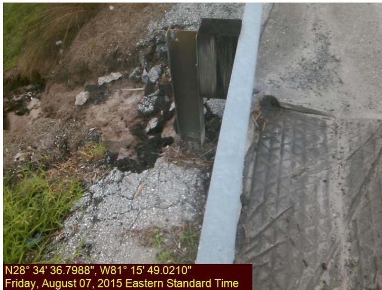
Photo 1 – Soil Shoulder Erosion
