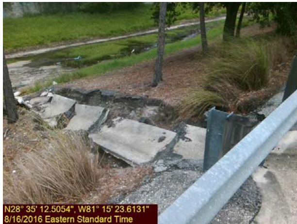
Photo 1 & 2 –36" deep erosion of Soil Shoulder and Front Slope. Conc. Flume collapsed and broken apart
