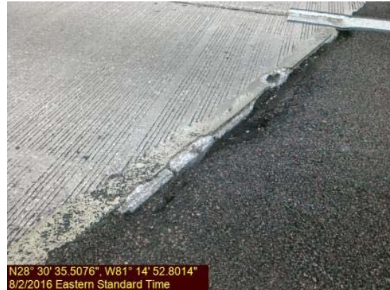
Photo 1 – 2 Pothole / Asphalt void adjacent south approach Curry Ford Bridge.
