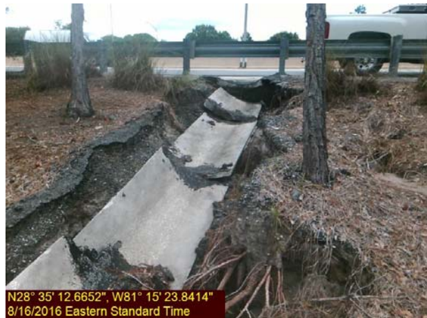
Photo 1 & 2 –36" deep erosion of Soil Shoulder and Front Slope. Conc. Flume collapsed and broken apart
