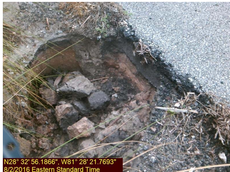
Photo 3 – Soil Shoulder erosion 18"-24 adjacent paved shoulder
