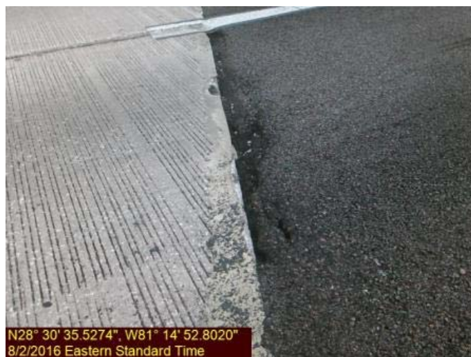
Photo 3 – Pothole / Asphalt void adjacent south approach Curry Ford Bridge
