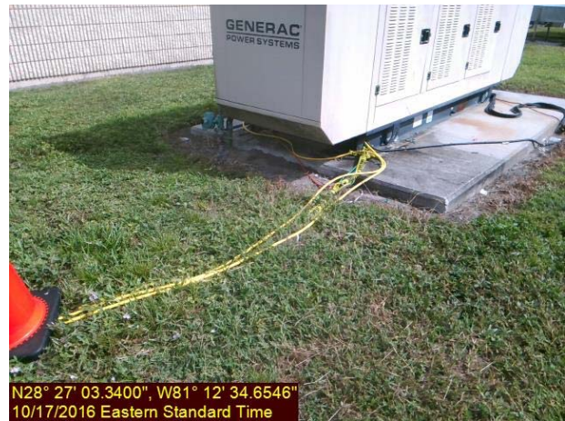
Photo 1 & 2 –Electrical wires laying on the ground unprotected.
