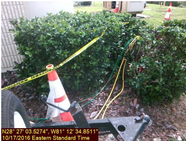
Photo 1 & 2 –Electrical wires laying on the ground unprotected.
