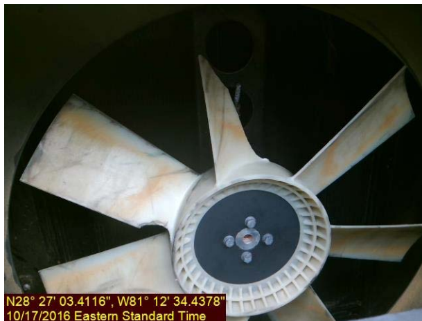
Photo 3 & 4 – Damaged fan and broken belt.
