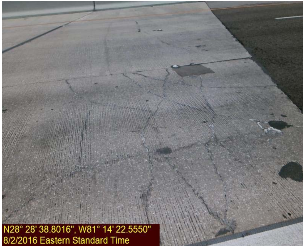
Photo 1 - 1/16 - 1/8 cracks in south approach slab (Lee Vista bridge no. 750375).
