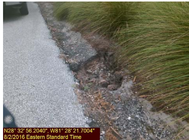
Photo 1 & 2 – Soil Shoulder erosion 18"-24 adjacent paved shoulder
