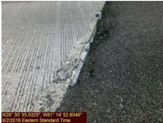
Photo 1 – 2 Pothole / Asphalt void adjacent south approach Curry Ford Bridge.
