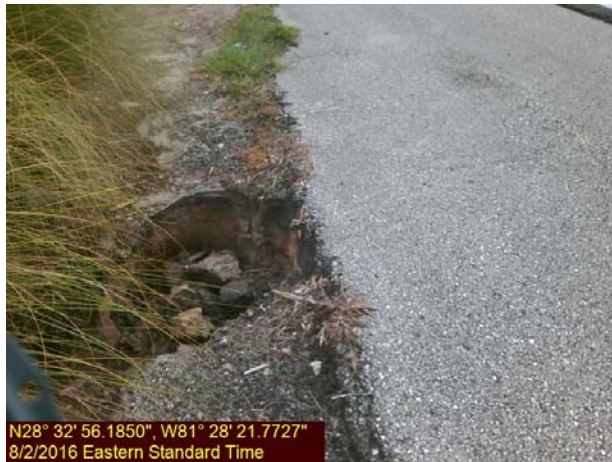
Photo 1 & 2 – Soil Shoulder erosion 18"-24 adjacent paved shoulder
