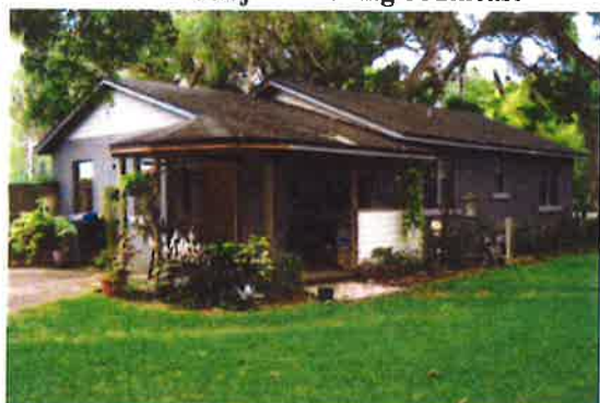
Rear View of Single Family Residence
