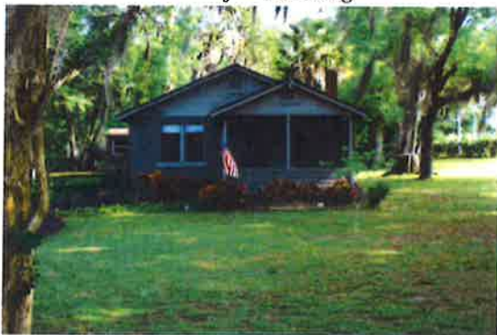
Front View of Single Family Residence
