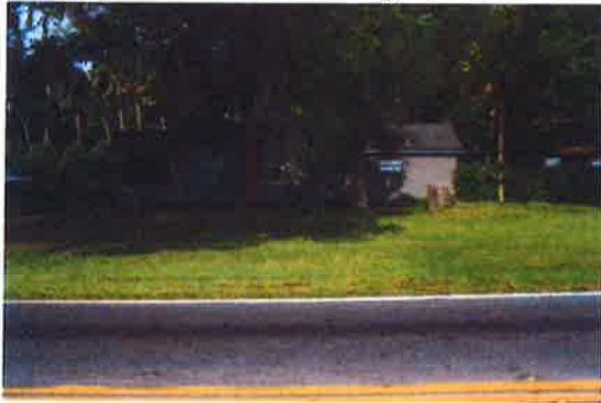
View of Subject Looking West
