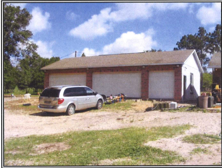
7. LOOKING NORTH AT THE DETACHED GARAGE
