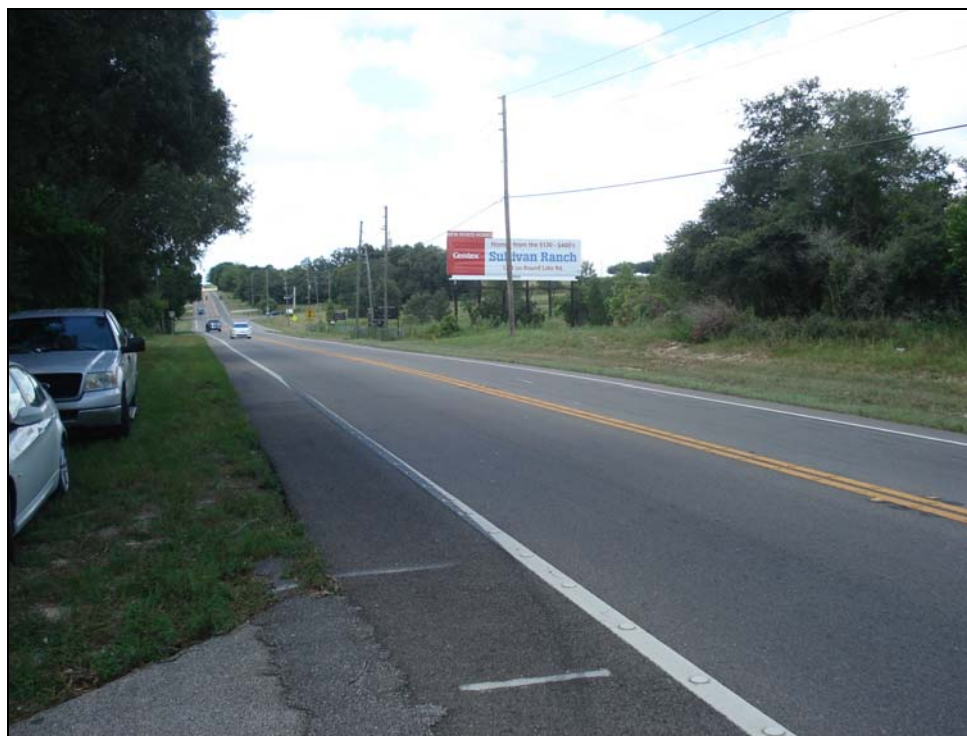
View of State Road 46, facing west
