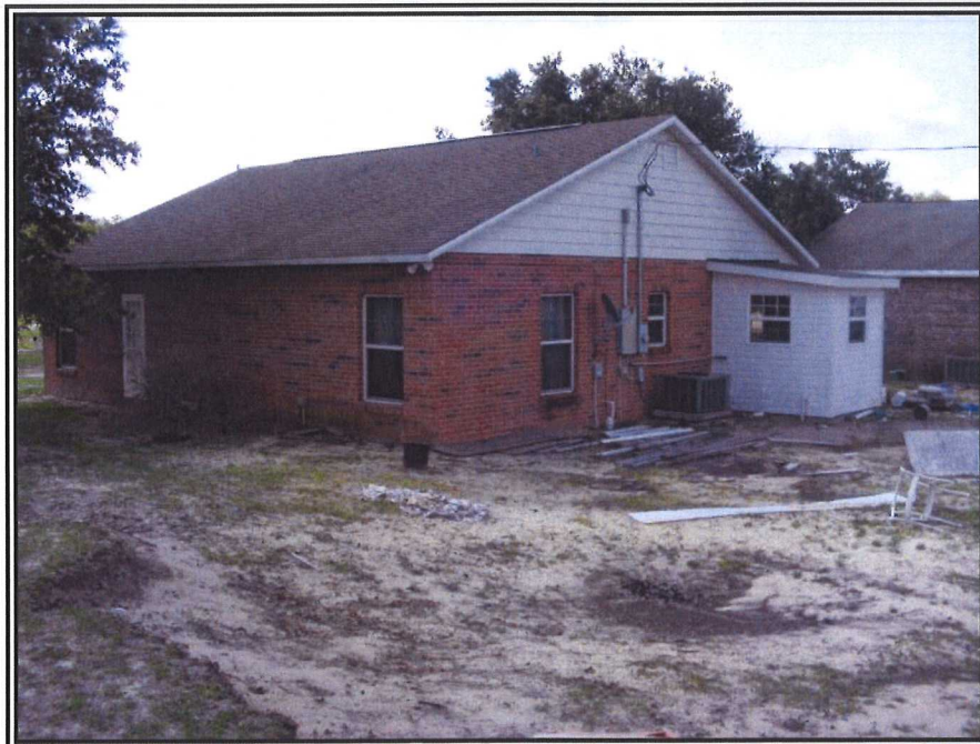
6. LOOKING SOUTHEAST AT THE REAR OF THE GUEST COTTAGE
