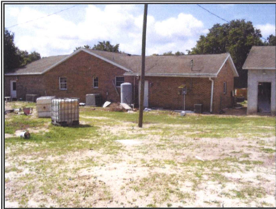
4. LOOKING SOUTH AT THE REAR OF THE RESIDENCE
