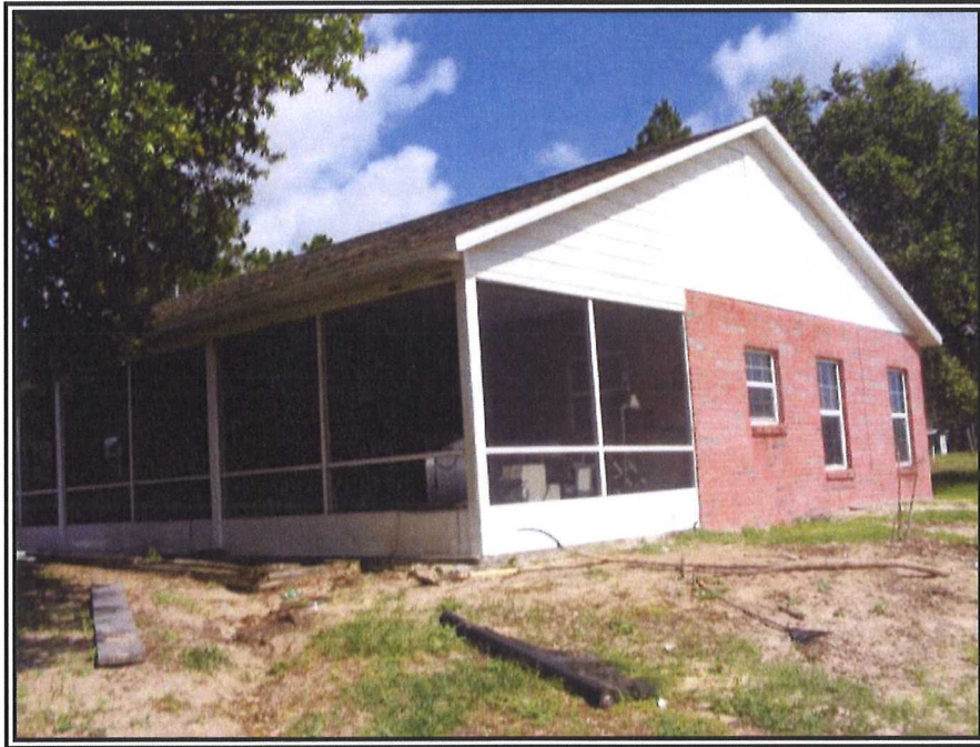
5. LOOKING NORTHWEST AT THE GUEST COTTAGE
