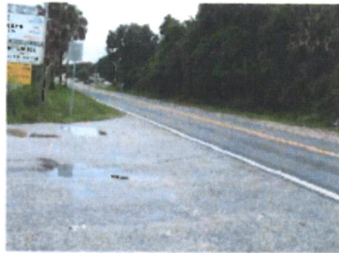
Intersection looking south along Plymouth Sorrento Road.
