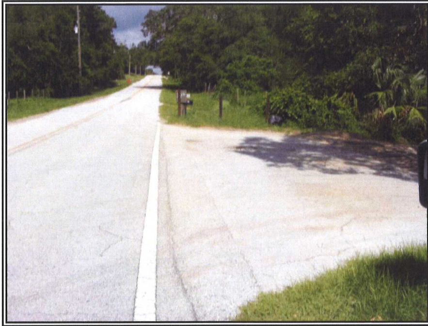
1. LOOKING WEST AT THE FRONTAGE ALONG HAAS ROAD
