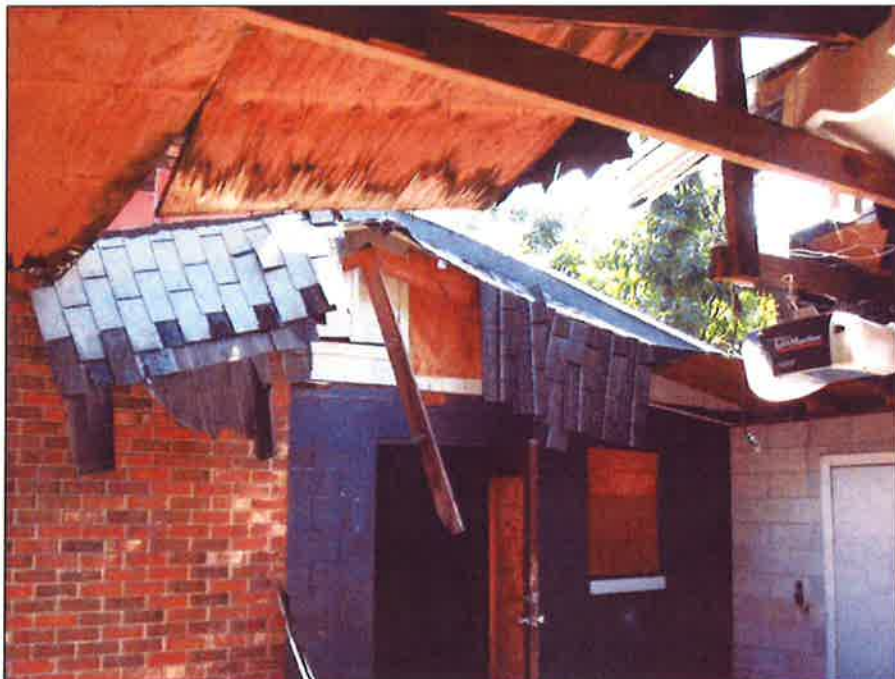
Interior view of the single family residence garage
