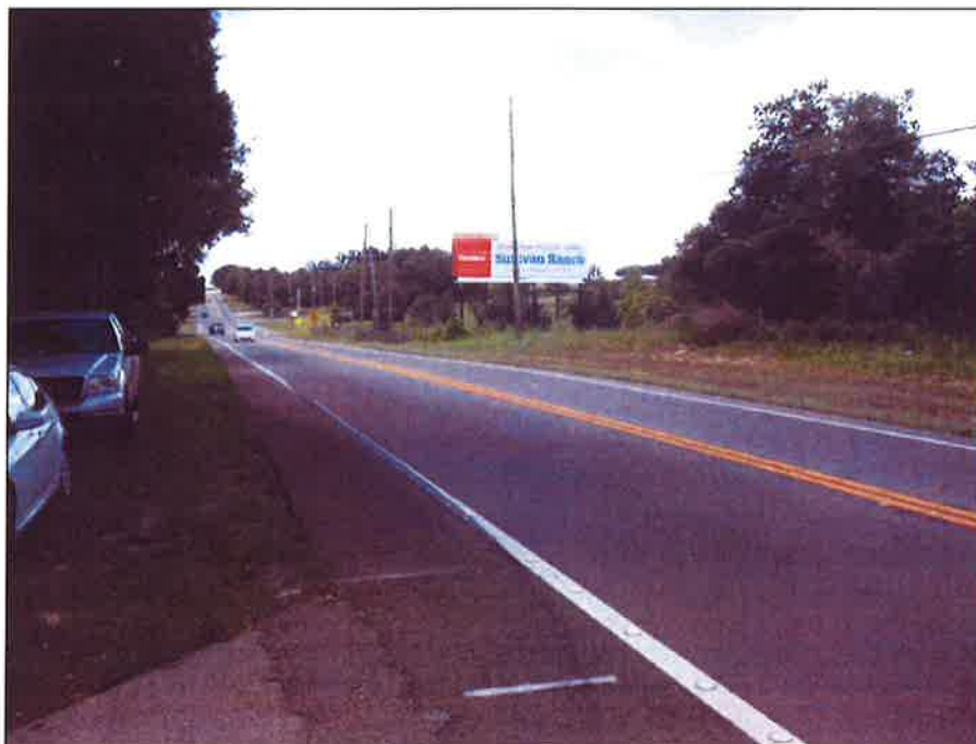
View of State Road 46, facing west
