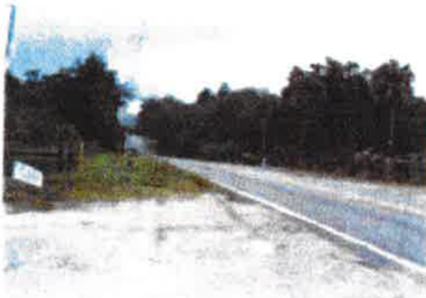
Intersection looking north along Plymouth Sorrento Road
