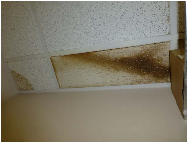
Figure 15 Damaged ceiling tiles SR 429 Forest Lake Mainline Plaza
