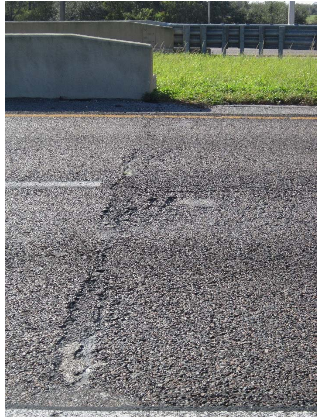
Figure 18 Raveling asphalt SR 528 Dallas Road Bridge
