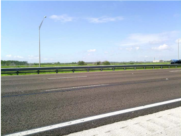
Figure 17 Faded pavement markings SR 528 adjacent to the airport
