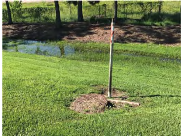
Figure 8 Boggy Creek Mainline Exterior Manhole Cover
