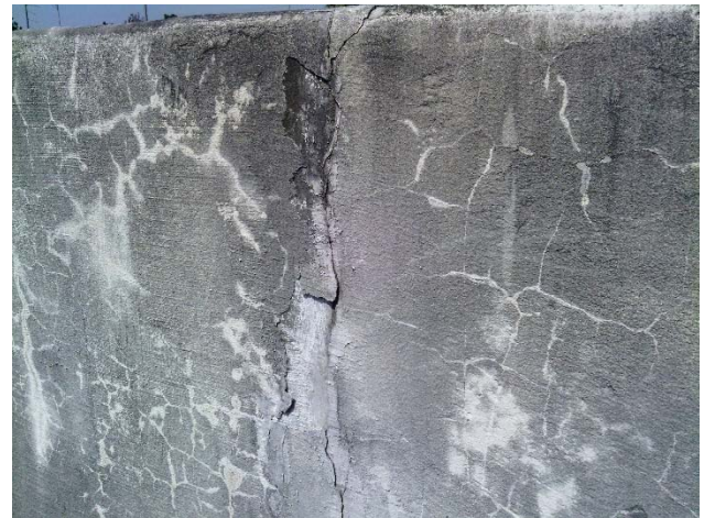
Figure 14 Barrier wall spalling SR 429 Forest Lake Mainline Plaza median
