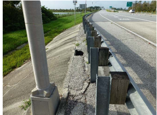
Figure 20 Depression along slope pavement at Goldenrod Mainline Plaza
