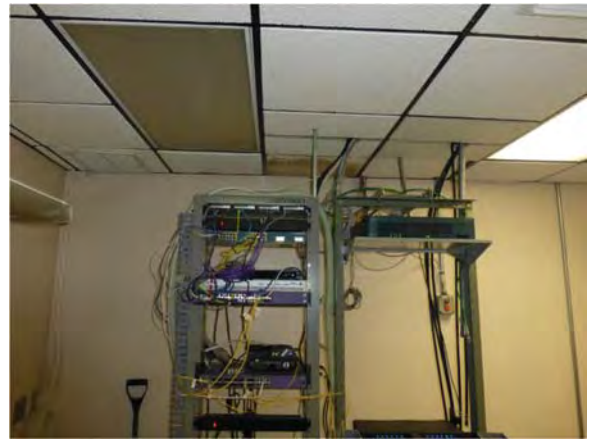
Figure 2 University Mainline CCTV Equipment Rack
