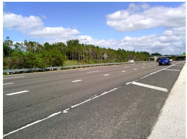
Figure 3 Pavement marking peeling SR 408 near Pine Hills Mainline Plaza
