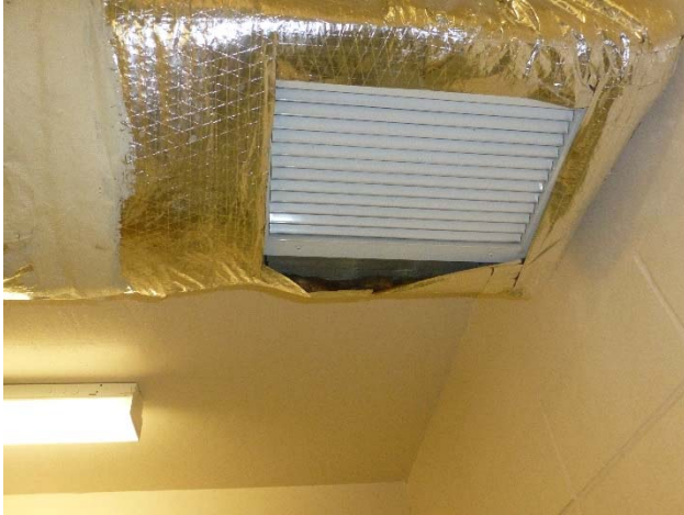
Figure 19 Minor duct repair needed SR 528 Dallas Boulevard On-Ramp Plaza
