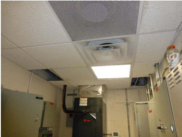
Figure 12 Missing ceiling tiles SR 417 University Ramp Plaza
