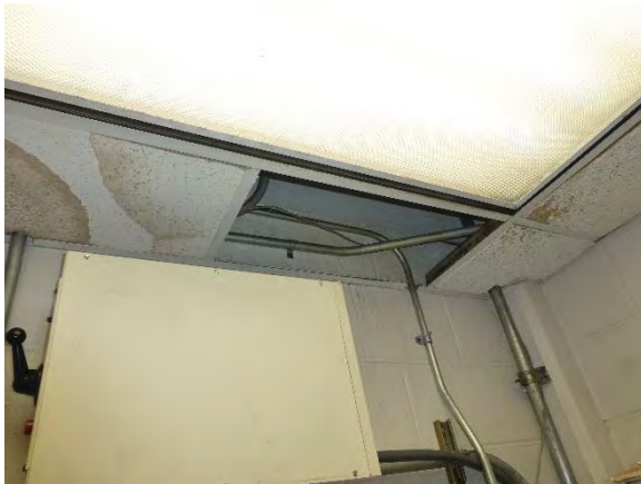
Figure 9 John Young Parkway Ramp On Missing Ceiling Tile
