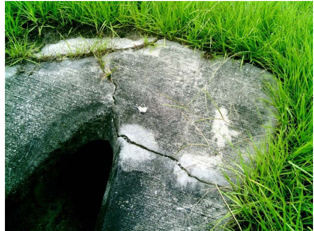
Figure 16 Cracked drainage structure at SR 429 Pond
