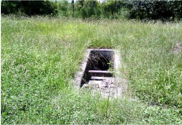
Figure 6 Drainage structure with vegetative obstruction at SR 414 Keene Road Pond
