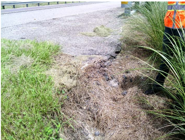
Figure 13 Roadside erosion northbound SR 429 at Franklin Street
