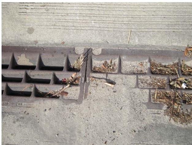
Figure 7 Obstructed bridge deck inlet SR 414 viaduct
