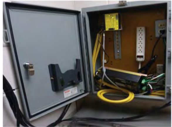
Figure 20 Landstar Ramp Off Light Curtain Controller
