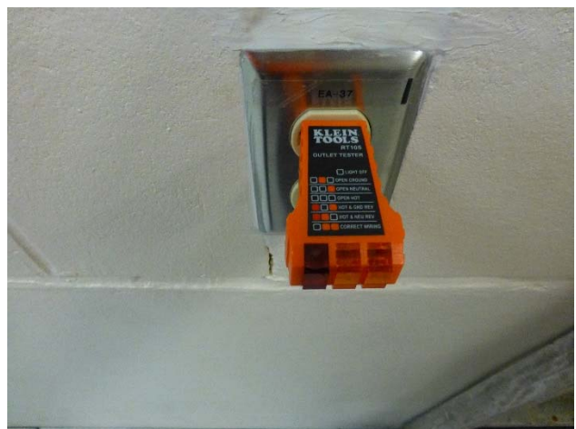
Figure 9 In-operable receptacle Coral Hill Mainline Plaza
