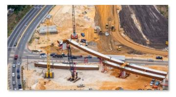
Half of the beams were up by the end of December. The operation required notifying the community each week about the latest schedule for the nighttime S.R. 46 road closures and detours needed to place and secure the beams.
