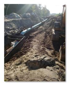
item along this section was the relocation of the Florida Gas Transmission line into a new 50-foot easement along S.R. 46 (photo, left).
