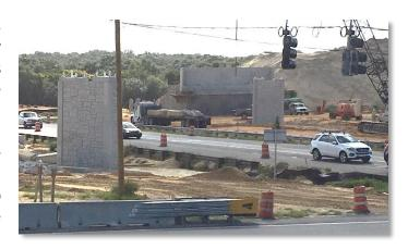
In November, crews were ready to begin installing the large, U-shaped beams for the flyover bridge. The beams ranged from 120 feet long on each end by the abutment walls, to 231 feet long spanning over S.R. 46 (photo, below).
