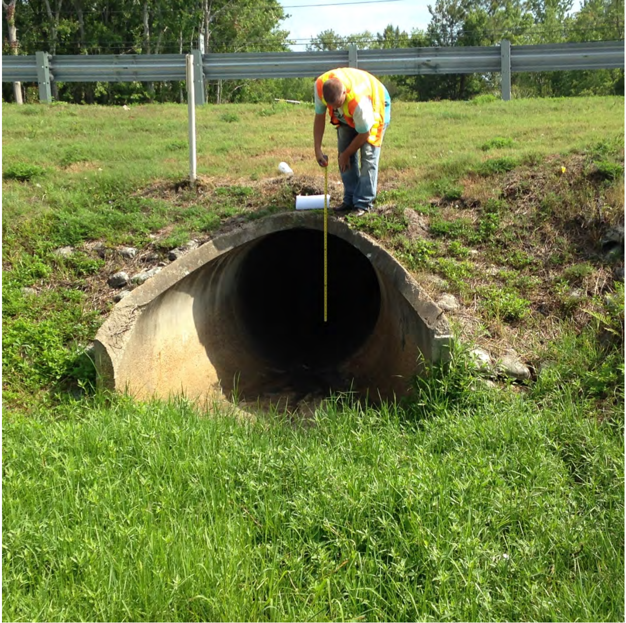
SR 50-CD7 (4' x 4' CBC & 1-54" RCP Jointed) (South Side of the Culvert)
