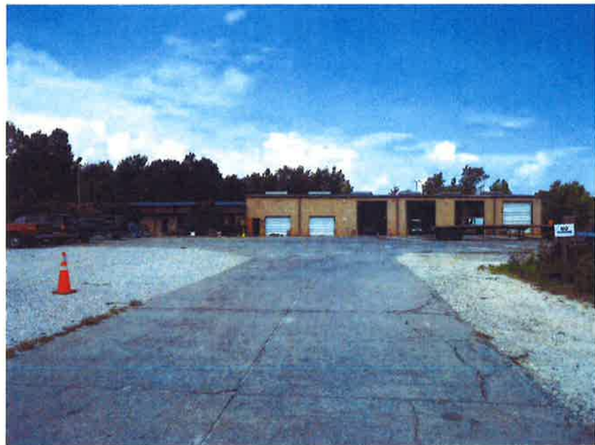
View of the subject improvements located to the rear of the property looking west. The office area is located on the left side and the warehouse area is located on the right side.
