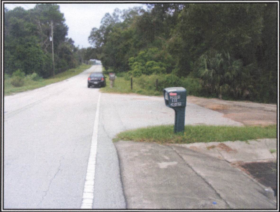
1. LOOKING WEST AT THE FRONTAGE ALONG HAAS ROAD
