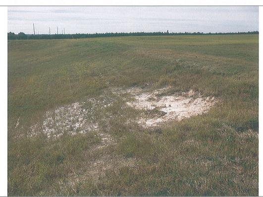
**Photo 2:** Bare spot located on the berm of storm water retention pond #3.
